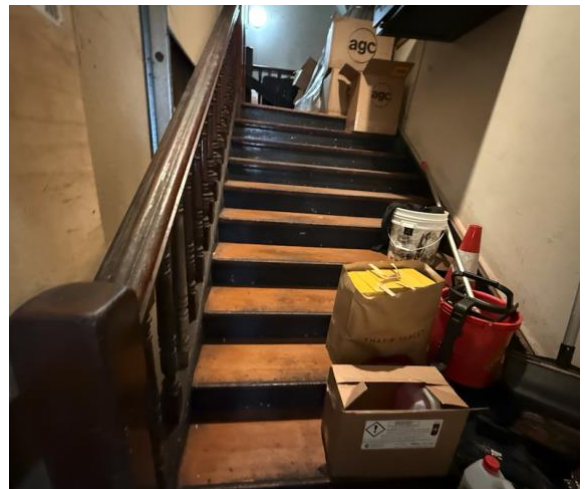
Figure 16 – Remnant staircase within ground floor tenancy
