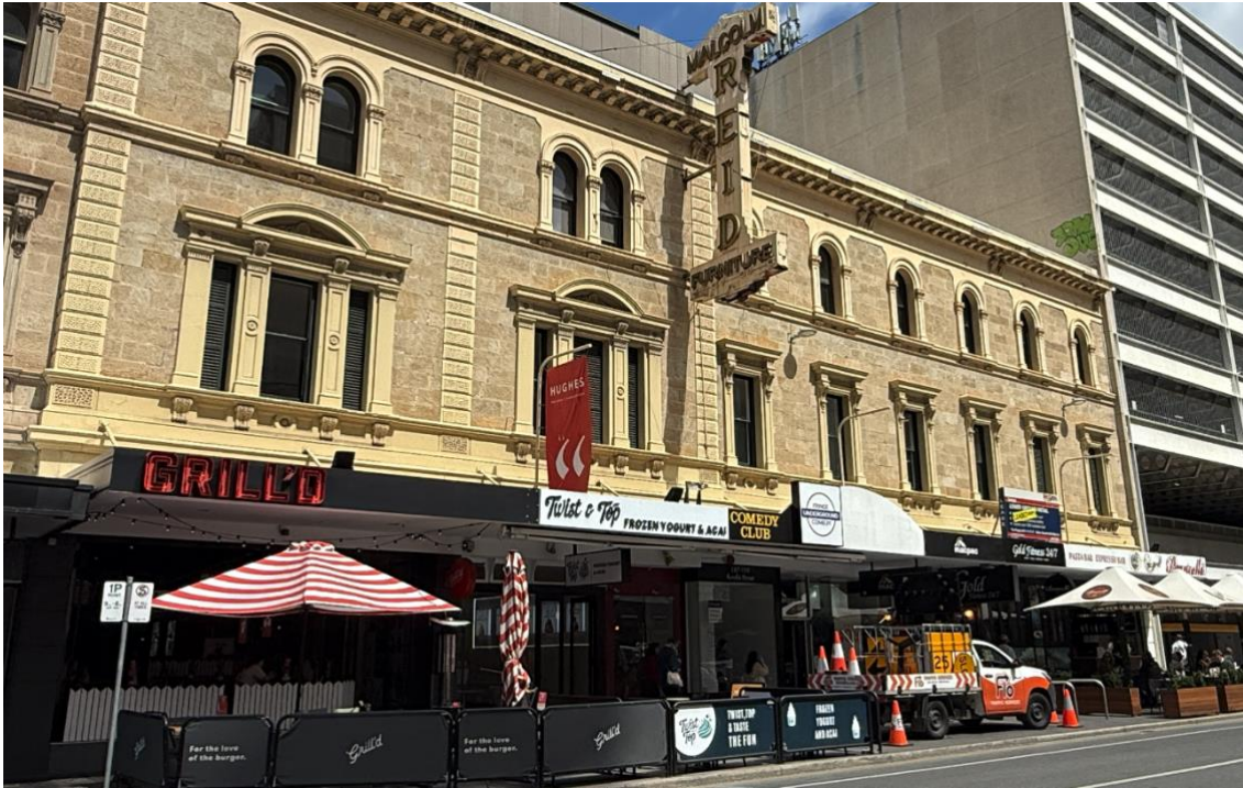
Figure 14 – Current awning / verandah, 187-195 Rundle Street Adelaide
