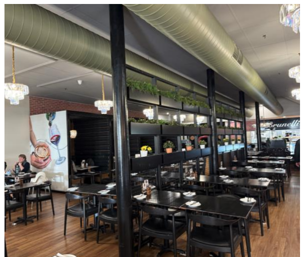
Figure 13 – Ground floor tenancy with remnant steel columns
