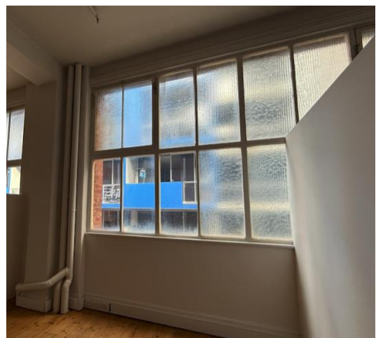
Figure 21 – York Street windows.
