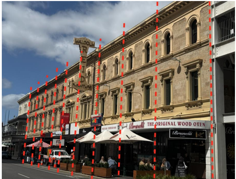
Figure 24 –Rhythm and spacing of fenestration reflects original 'terrace' shop and dwelling use, rather than large floor plate retail.
