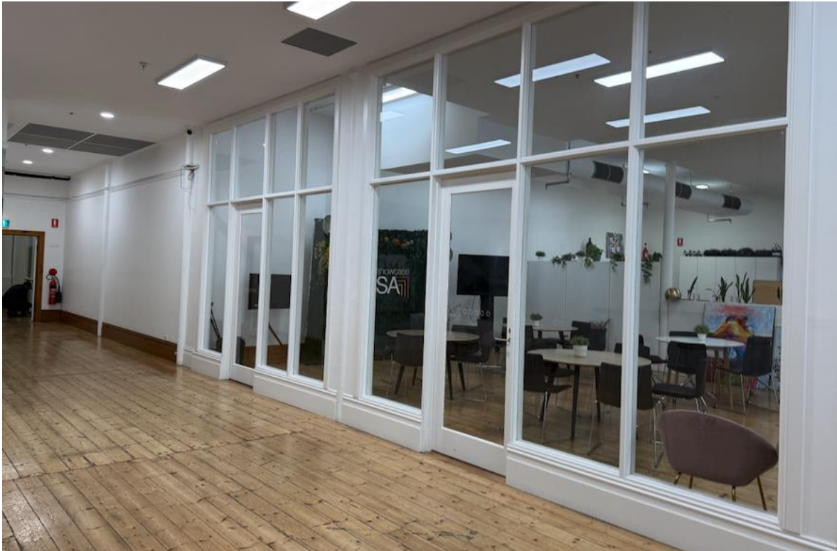
Figure 17 – First floor tenancies. Provenance of floor unknown, as it includes the infill of the original void. Glazed tenancy walls also clearly contemporary
