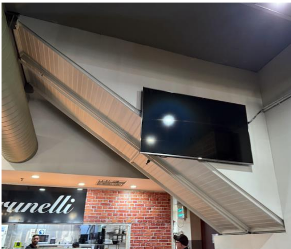
Figure 15 – Remnant staircase within ground floor tenancy
