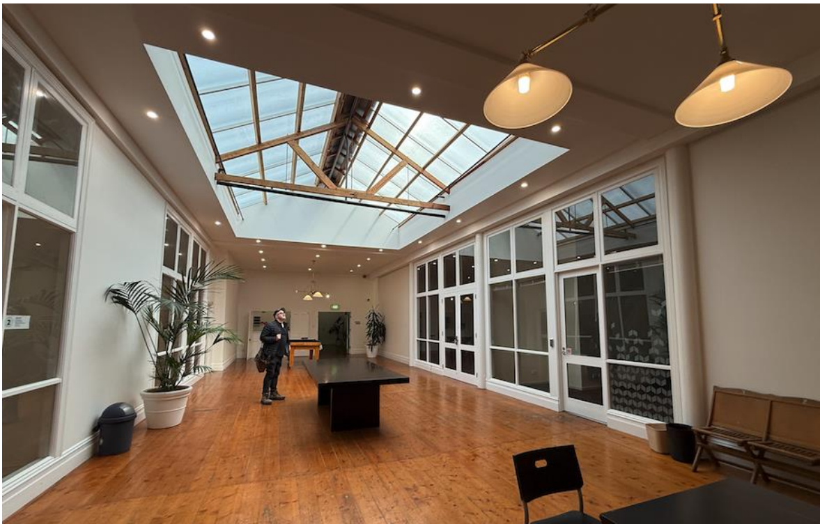
Figure 18 – Second floor tenancies. Provenance of floor unknown. Glazed tenancy walls also clearly contemporary, as is skylight
