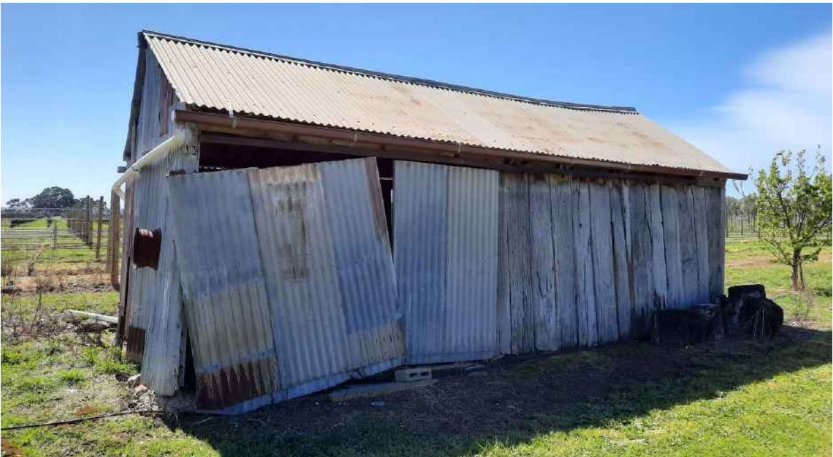
Early slab timber shed with later corrugated steel alterations (GGA, 2021).
