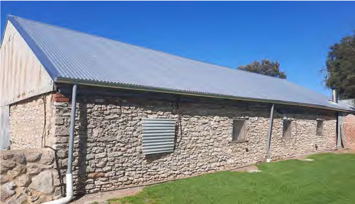
Early masonry construction and corrugated iron to early outbuilding (GGA, 2021).
