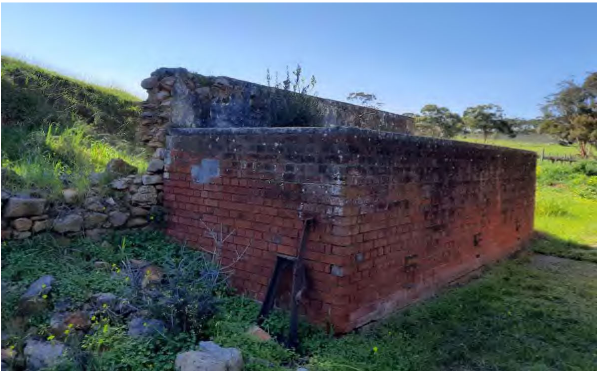
Three surviving slate fermenting tanks relating to former upper level of cellar with intact brick exterior shell (GGA, 2021).
