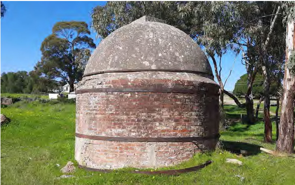
Brick tank with rendered masonry dome with cast-iron banding, immediately south of excavated site (GGA, 2021).
