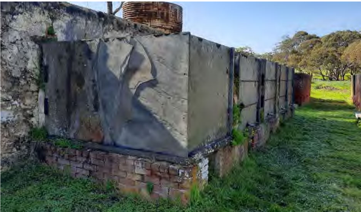
Five intact slate fermenting tanks abutting original north-east wall of former Tintara Winery cellar. Further three slate cellars to the immediate south-east (with brick lining) (GGA, 2021).
