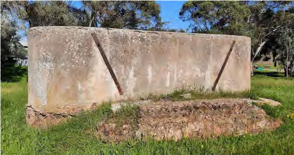
One of two rendered masonry water tanks immediately south-west of excavated site (GGA, 2021).
