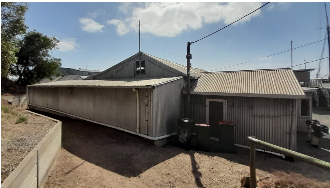
Rear view of workshop sheds.
