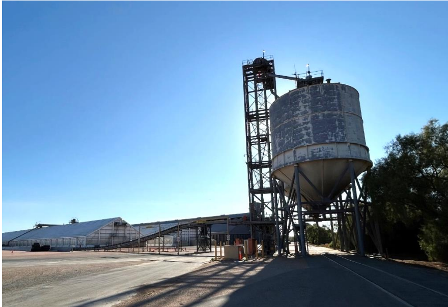
Conveyor belt system connected to railway outloading bins.
