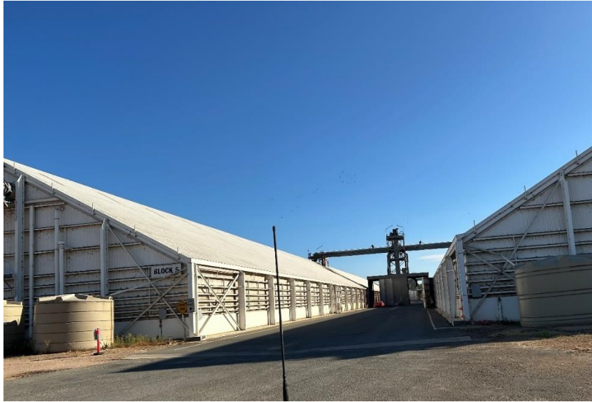
Southern elevation of paired sheds with shared receiveal hopper and elevator.
