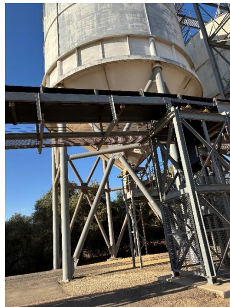
Conveyor belt system connected to railway outloading bins.
