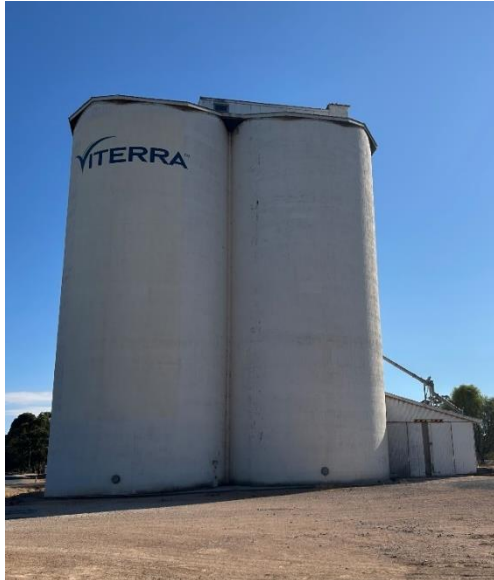
Southern concrete vertical silo (left) of the town site with receival hopper (right).
