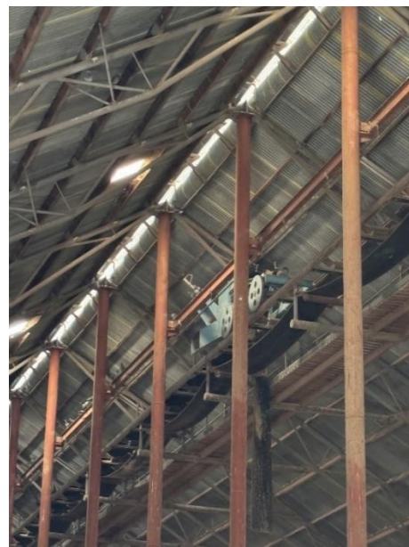
Interior of the horizontal shed silo (left) with grain conveyor (right).
