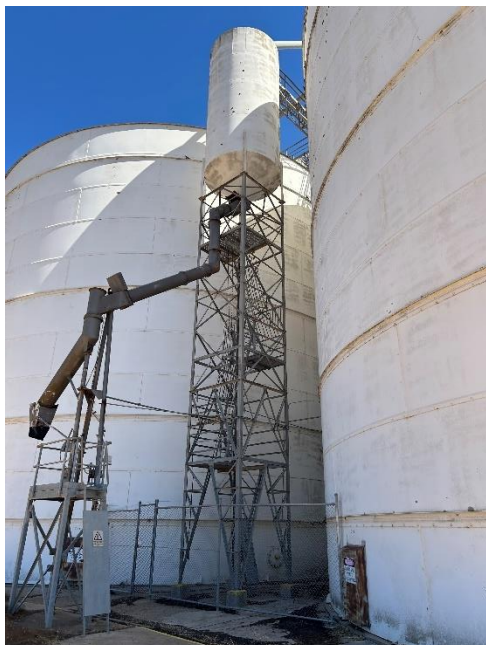
Outloading bin and outloading chute (left) and receive hopper enclosure (right).
