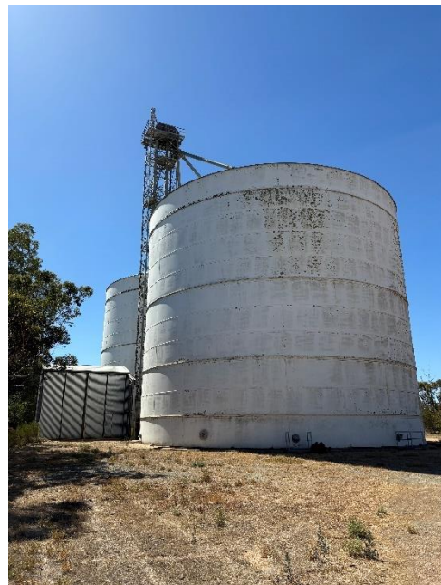
Outloading bin and outloading chute (left) and receive hopper enclosure (right).
