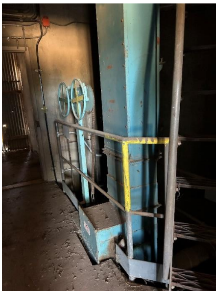
Interior of the concrete vertical silo showing the grain elevator (left) and the railway outloading chute to the silo's western side (right).
