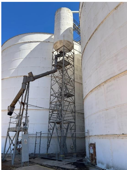
Outloading bin and outloading chute (left) and receival hopper enclosure (right).
