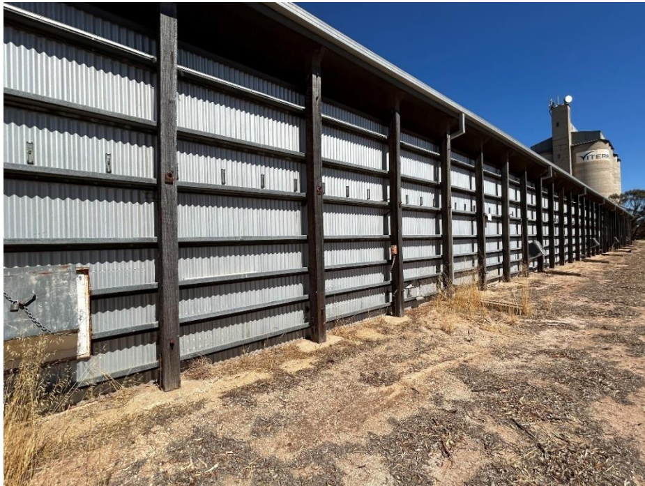
Northern elevation of the horizontal shed silo showing the building's timber and steel external structure.
