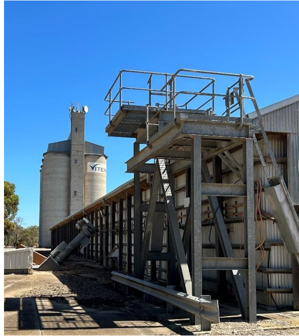
Outloading shoot to the concrete vertical silos northern elevation (left) and the southern elevation of the horizontal shed silo (right).
