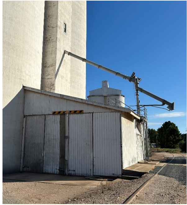
Southern concrete vertical silo (left) of the town site with receival hopper (right).
