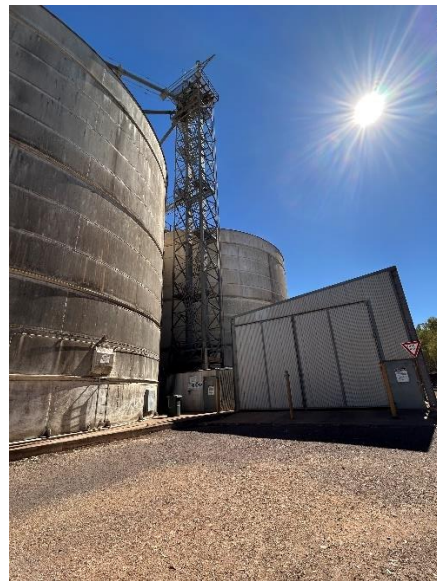
The steel vertical silo with exposed grain elevator and receival hopper (right).
