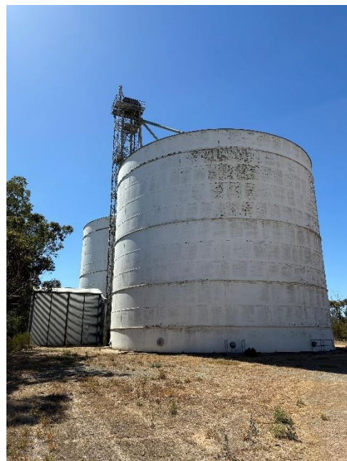
Outloading bin and outloading chute (left) and receival hopper enclosure (right).
