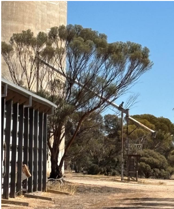
Outloading shoot to the concrete vertical silos northern elevation (left) and the southern elevation of the horizontal shed silo (right).
