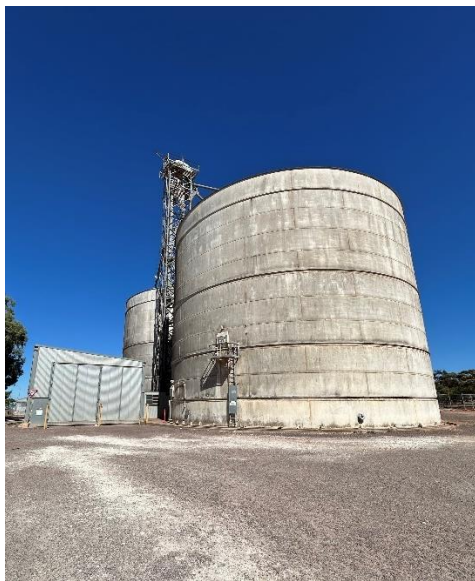
The steel vertical silo with exposed grain elevator and receival hopper (right).
