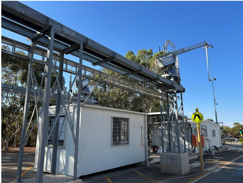
Classification centre with automatic grain probe system.
