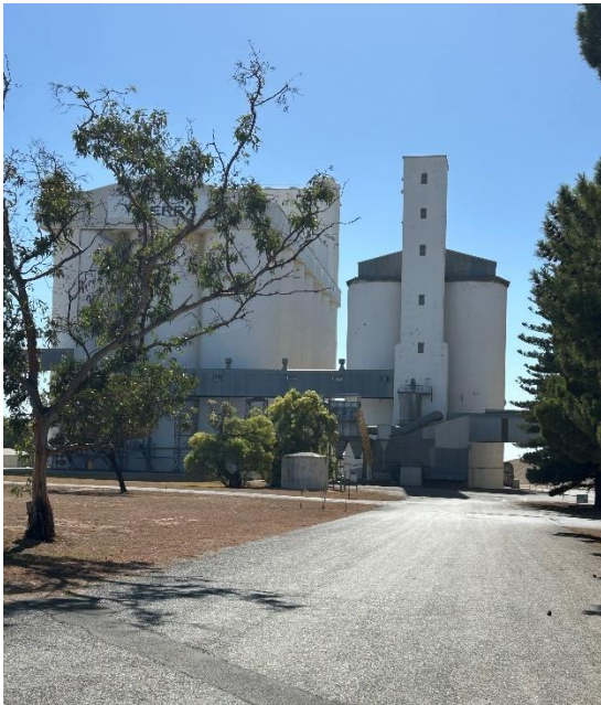
The 21-cell and 16-cell concrete vertical silos at Ardrossan (left) and the view north-east alongside the 24-cell and 36-cell concrete vertical silos.
