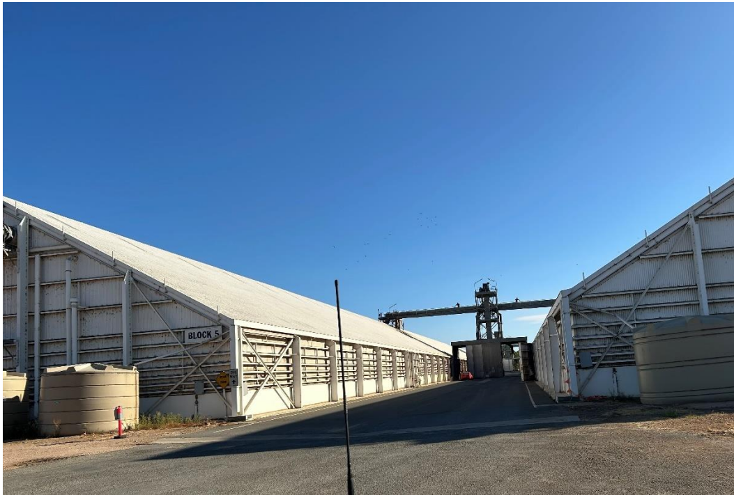
Southern elevation of paired sheds with shared receival hopper and elevator.
