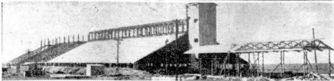
Eastern elevation of the horizontal shed silo at Ardrossan during construction in 1952. The grain elevator and hopper receival shed are on the right.
