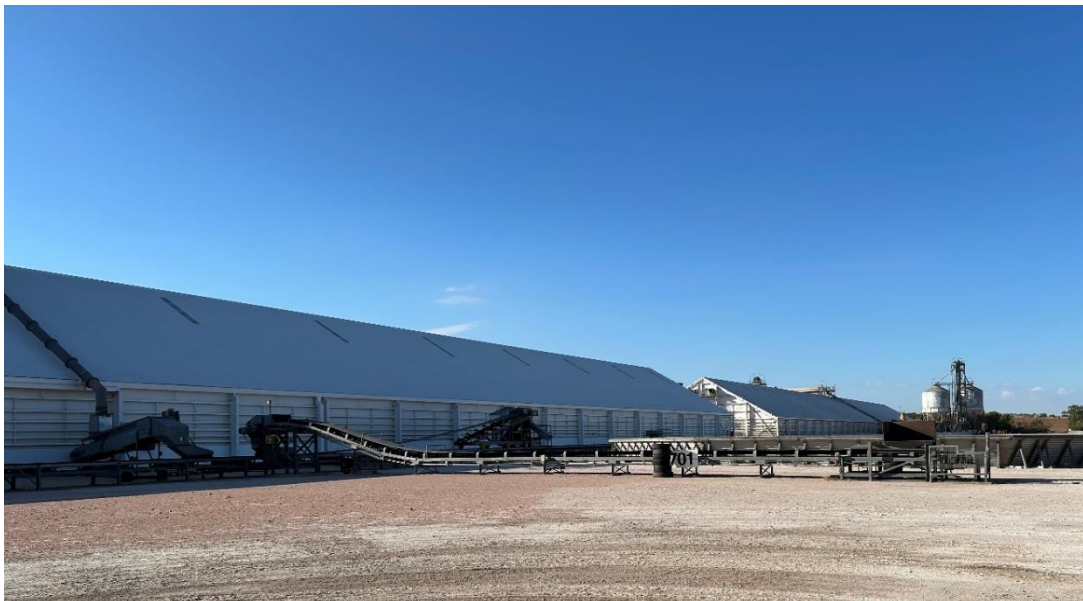
Paired sheds and conveyor system at the Gladstone bunker site in March 2025.
