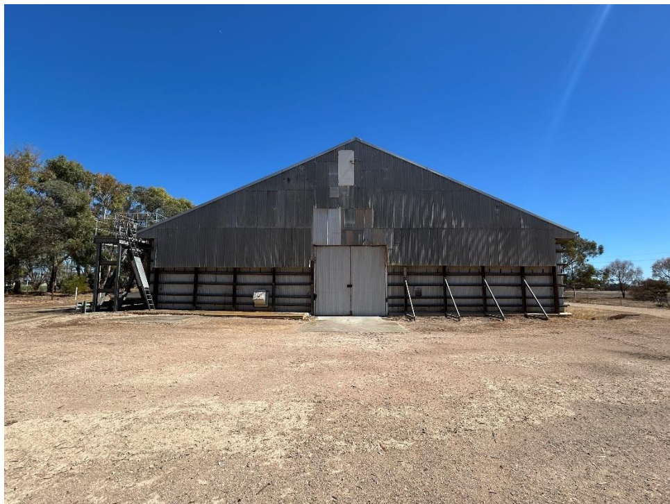
Eastern elevation of the horizontal shed silo.
