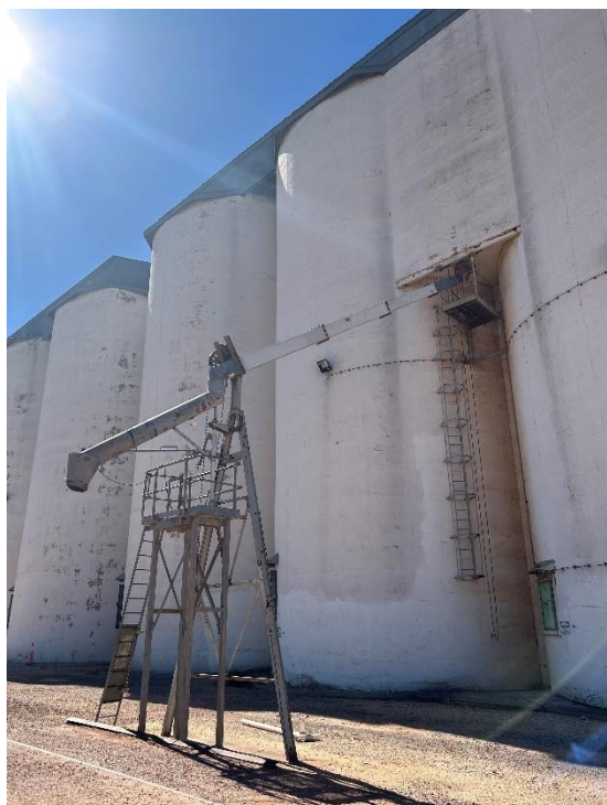
Detail of railway outloading spout (left) and receival hopper (right) of the northern concrete vertical silos.
