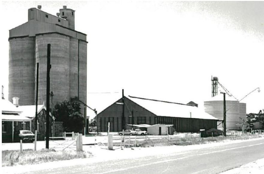
Railway Station Complex and Silos at Balaklava (SHP 12942). All three silos, cylindrical concrete vertical (left), horizontal (centre), and cylindrical steel vertical (right) were built by SACBH. The horizontal 'shed-style' silo was the first storage erected on the site in 1956, but has since been demolished.
