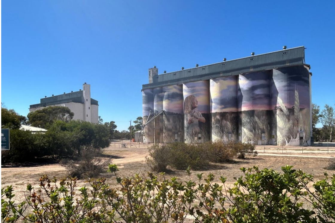
Kimba Bulk Grain Handling Complex.
