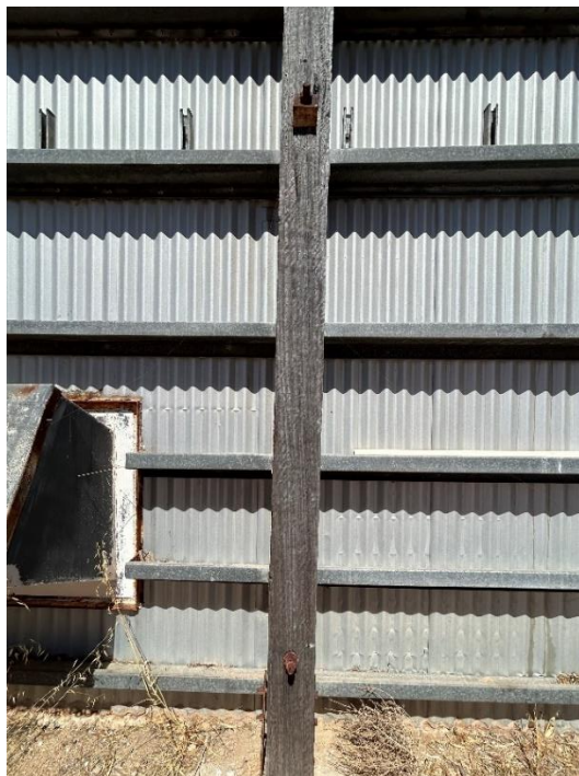
Additional support (left) and timber posts to the exterior of the horizontal shed silo (right).
