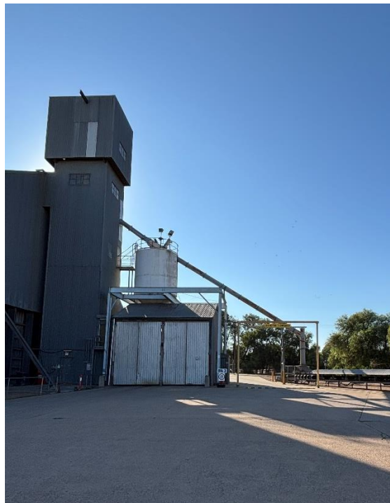
Grain elevation, receival hopper and outloading chute to eastern elevation of the horizontal shed.
