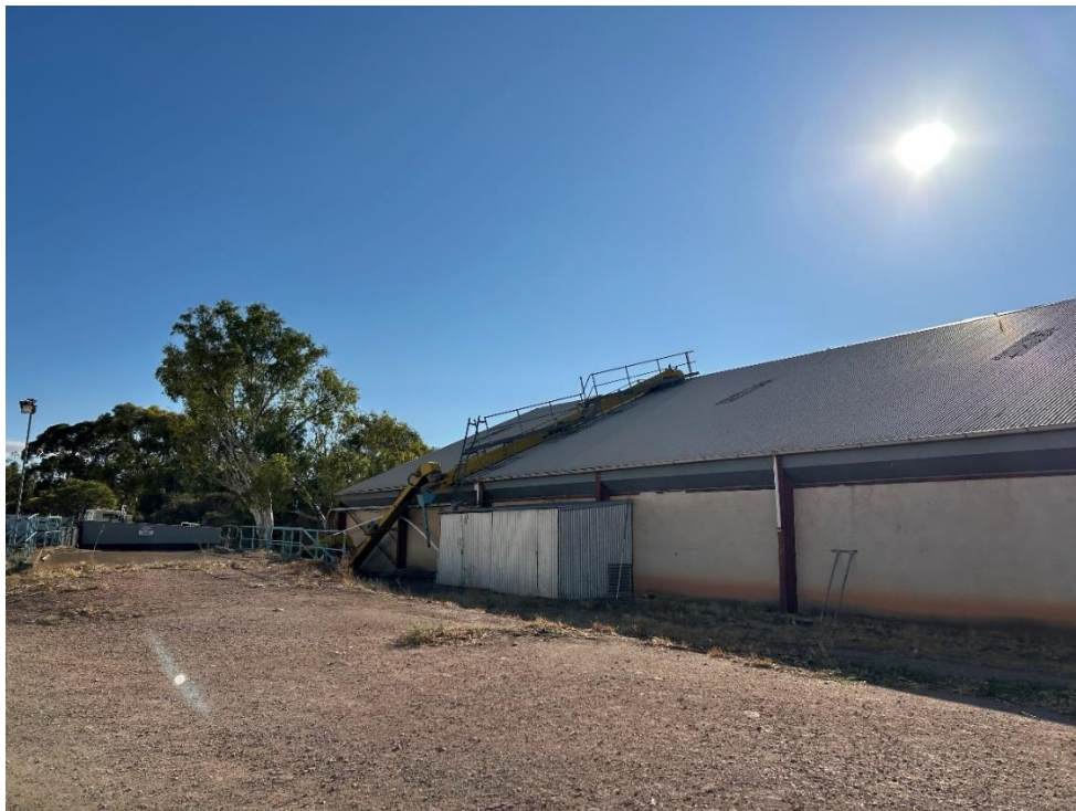
Western elevation of the horizontal shed silo.
