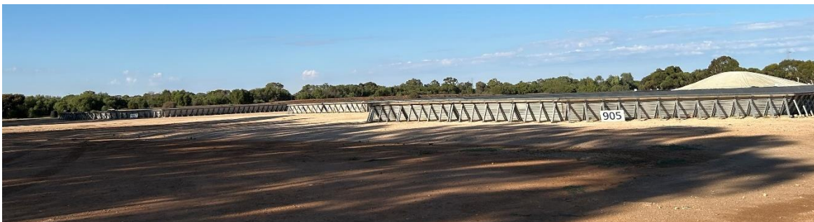
Bunker storage looking west.
