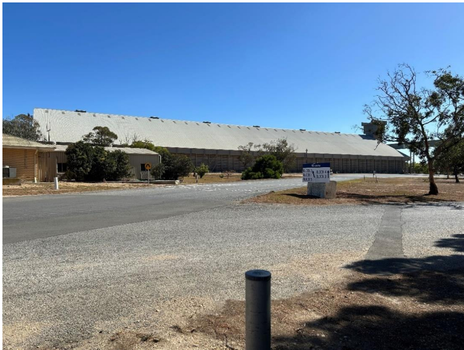
The horizontal shed constructed c.1969.
