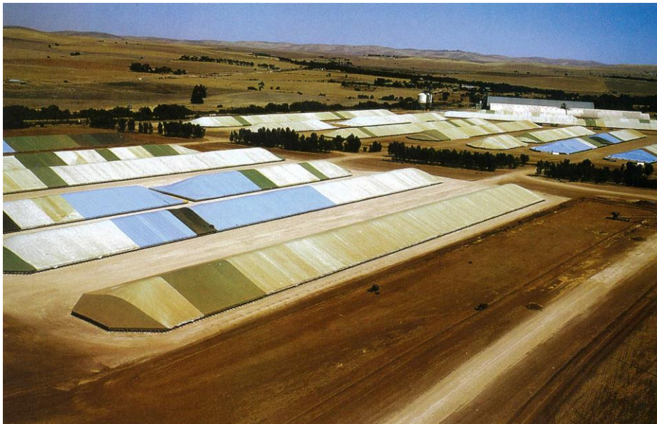
Bunker storage at Gladstone during the 2001-2002 harvest. Gladstone received a record 553,162 tonnes of grain during the season.
