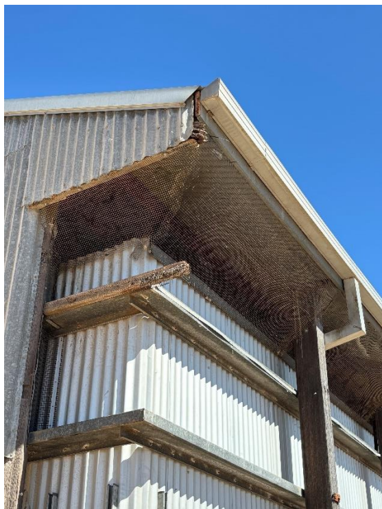
Mesh netting and gutter system of the horizontal shed (left) and direct cell outloader (right).
