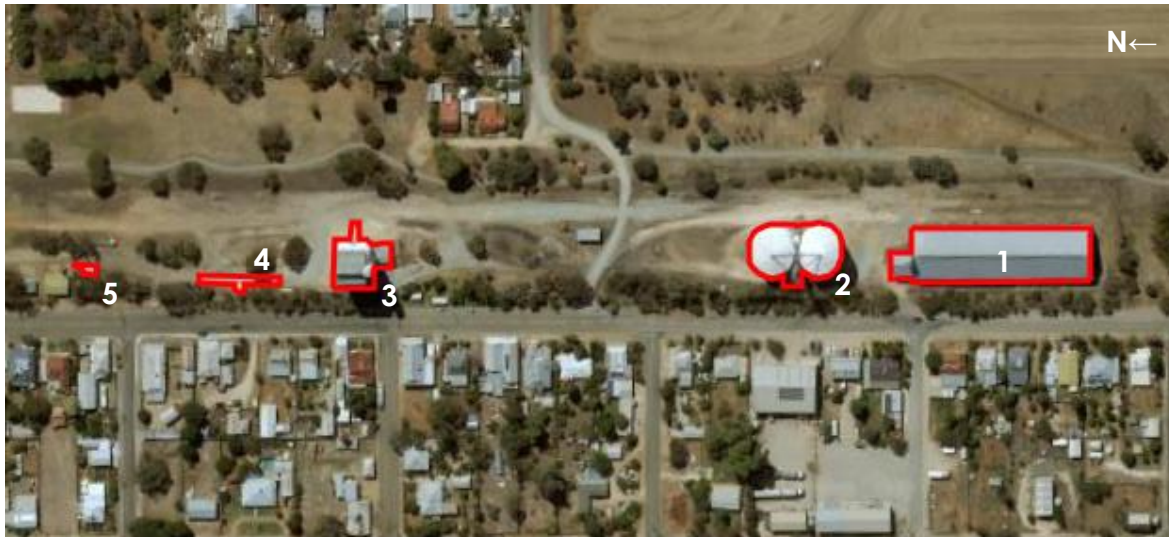
Aerial view of the Brinkworth Bulk Grain Handling Complex showing main elements.
