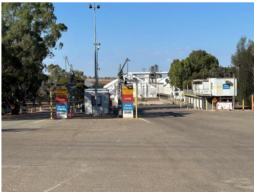
Classification centre erected in 2019 with paired sheds in background.
