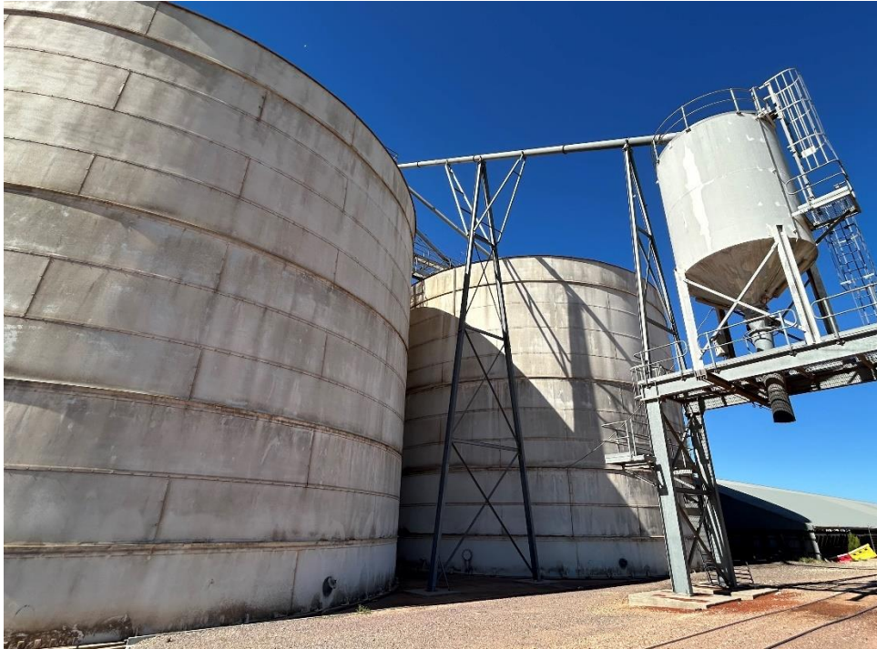
Steel vertical silo connected to railway outloading bin.
