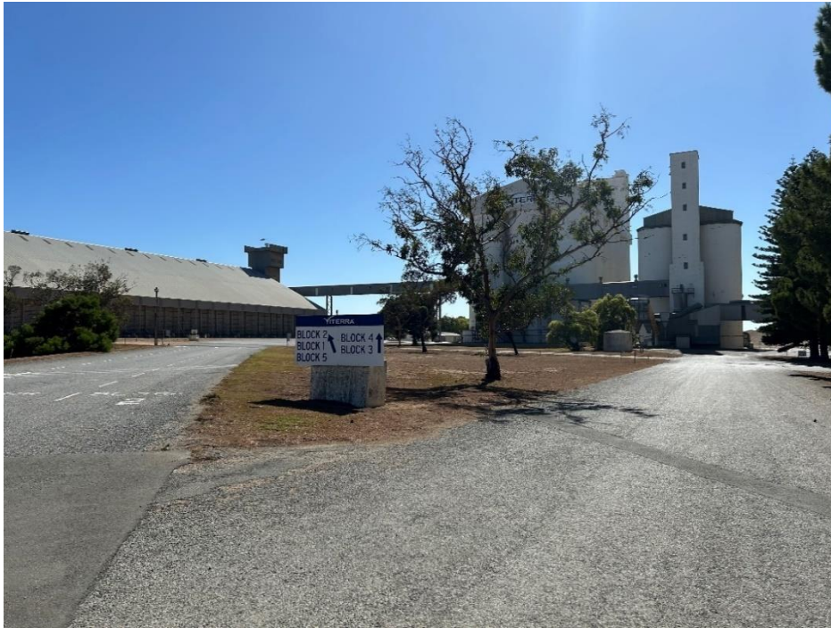
Storage at the Ardrossan Bulk Grain Handling Complex connected by an elevated enclosed conveyor system.
