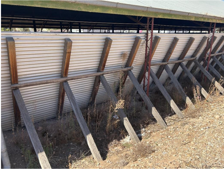
Retaining walls built of galvanised corrugated iron and timber.
