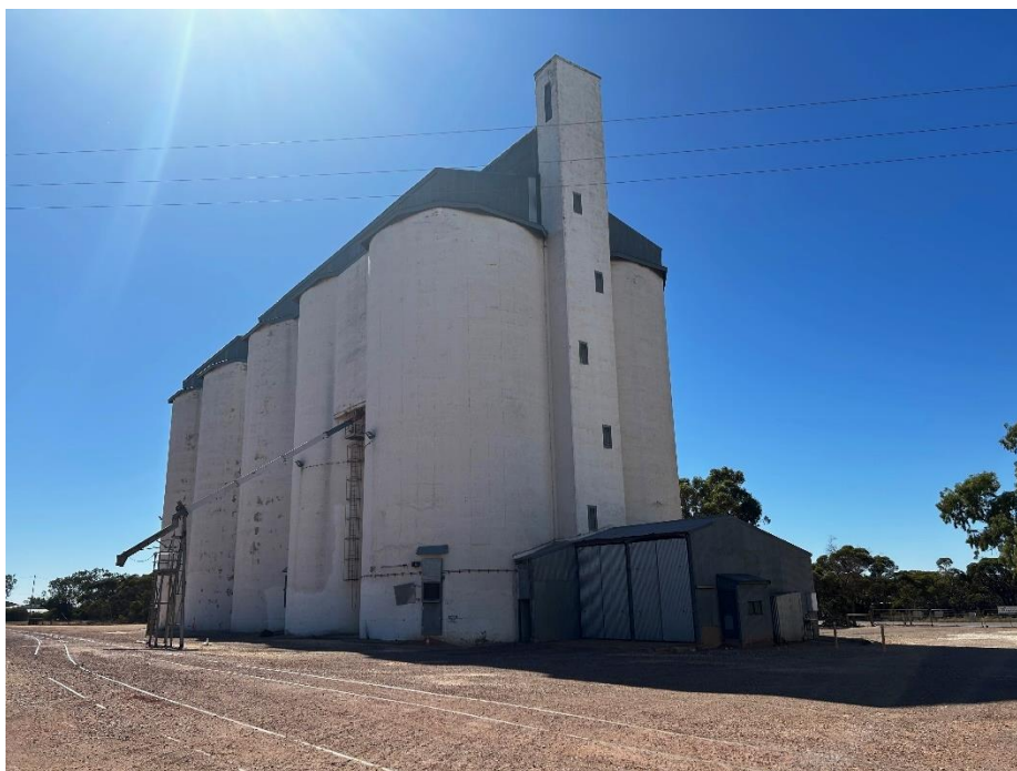
The northern concrete vertical silo showing the receival hopper shed, grain elevator, direct cell outloader, and railway outloading spout.
