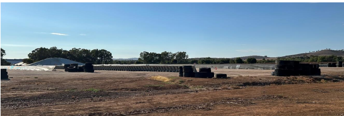
Bunker storage looking south east. When filled with grain, each bay is covered with tarpaulins and secured with tyres.
