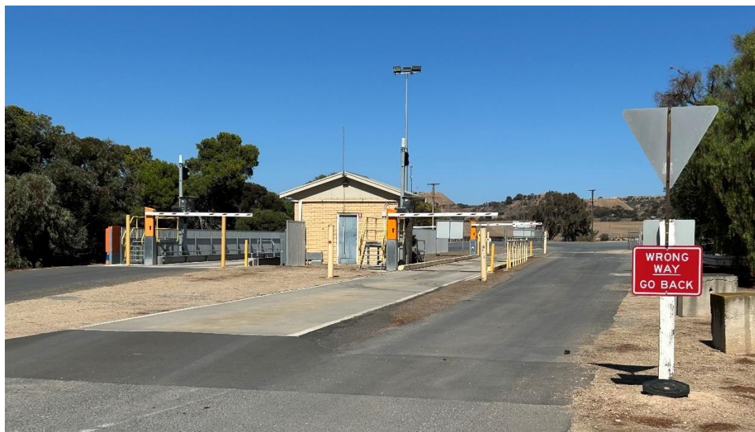
Two of the weighbridges.
