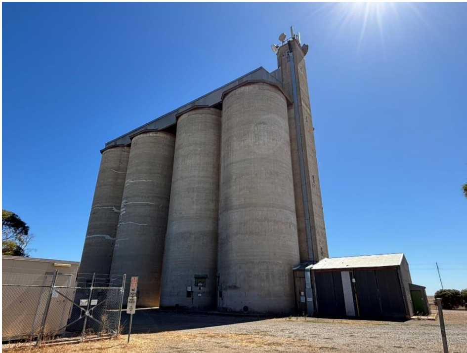
The concrete vertical silo at Paskeville.
