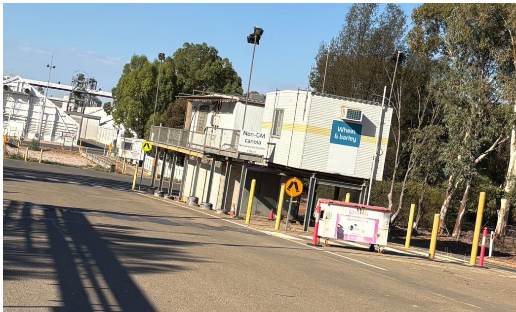
Eastern classification offices with weighbridges and paired sheds in background.
