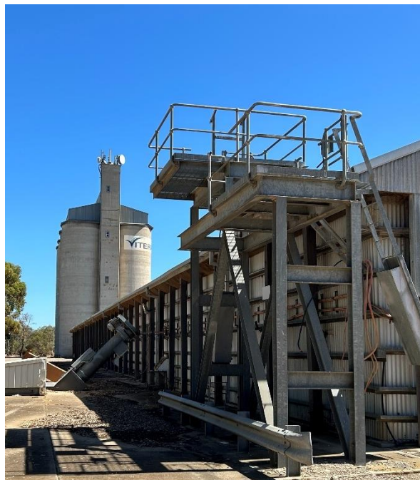
Outloading shoot to the concrete vertical silos northern elevation (left) and the southern elevation of the horizontal shed silo (right).
