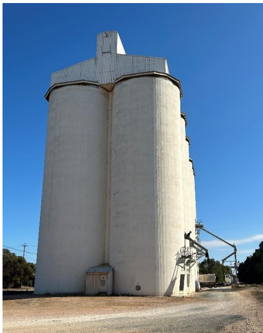
Northern concrete vertical silo (left) and treadplate weighbridge and weighbridge office (right).
