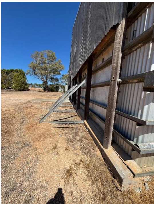
Additional support (left) and timber posts to the exterior of the horizontal shed silo (right).
