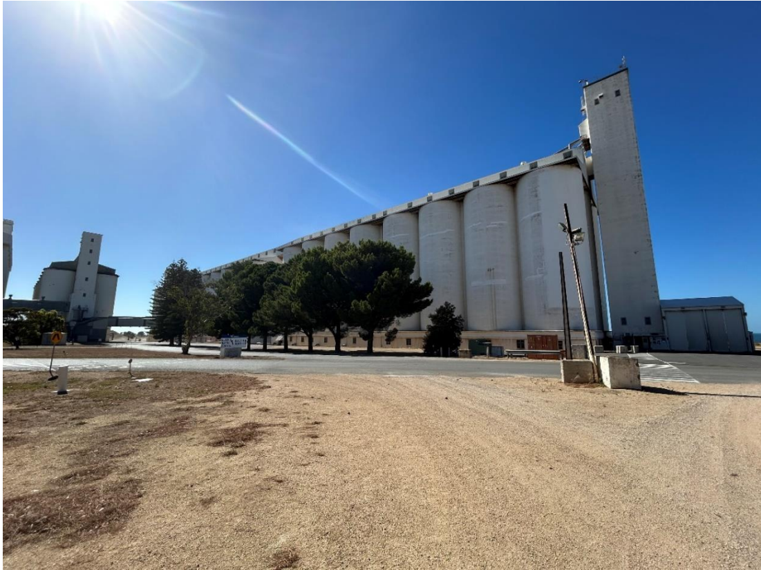
The 24-cell concrete vertical silo at Ardrossan.
