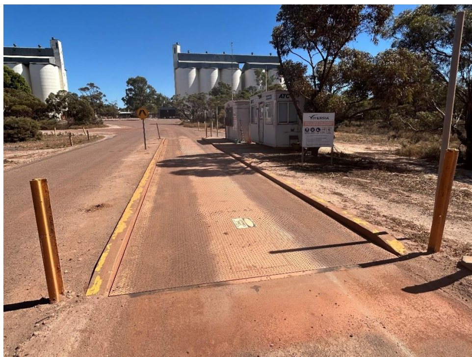
Weighbridge and weighbridge offices with concrete vertical silos in the background.
