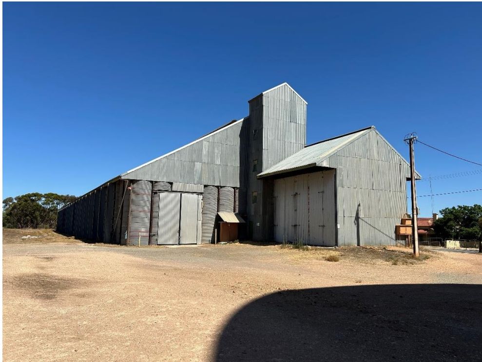
Northern elevation of horizontal shed silo.
