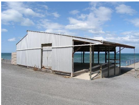
The goods shed at Port Julia (SHP 16681), built 1920.
