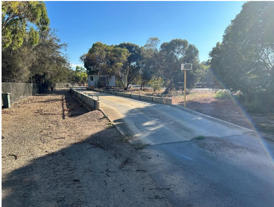
Eastern weighbridge and weighbridge office.
