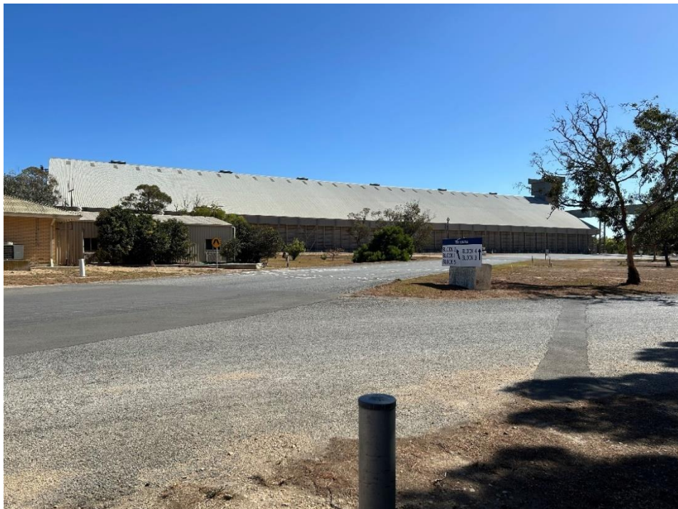
The horizontal shed constructed c.1969.
