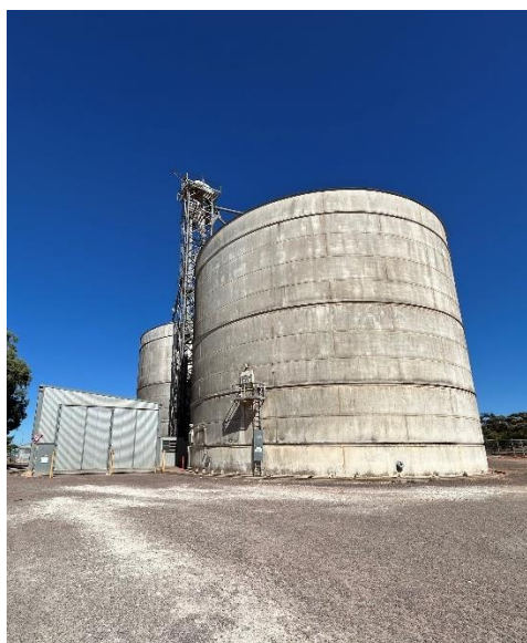
The steel vertical silo with exposed grain elevator and receive hopper (right).
