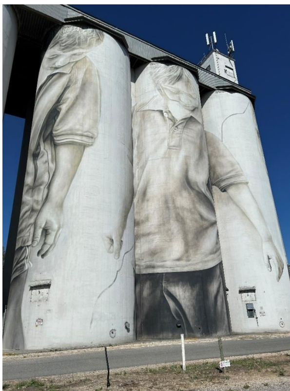
Detail of the eastern elevation of the silos.
