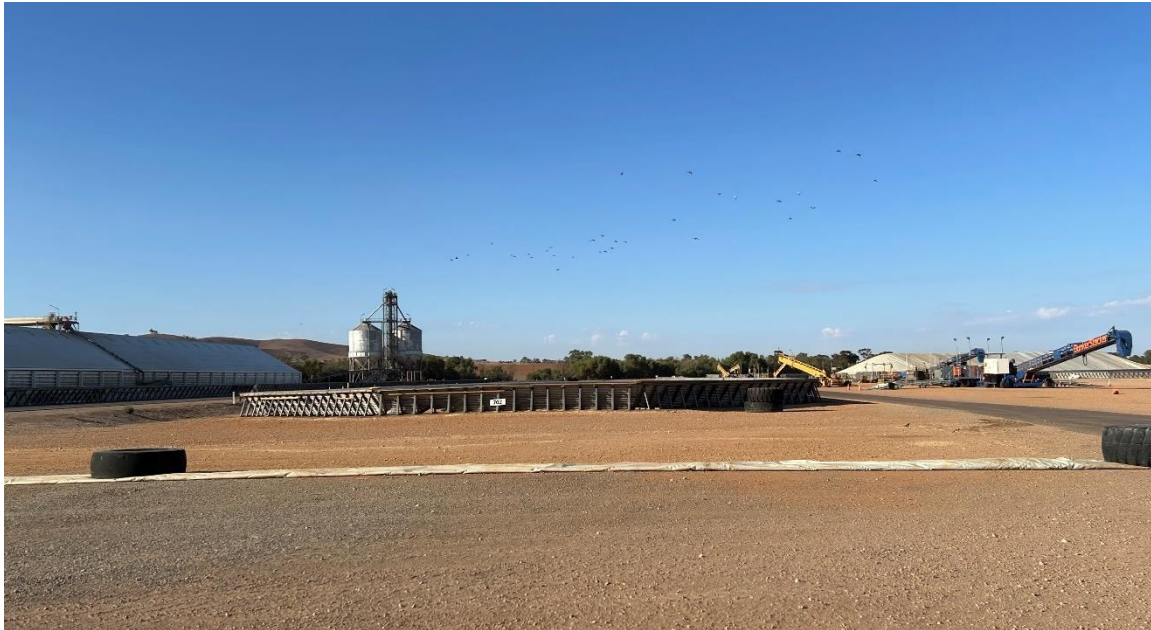
Edge of bunker storage with railway unloading bins.
