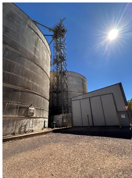
The steel vertical silo with exposed grain elevator and receive hopper (right).
