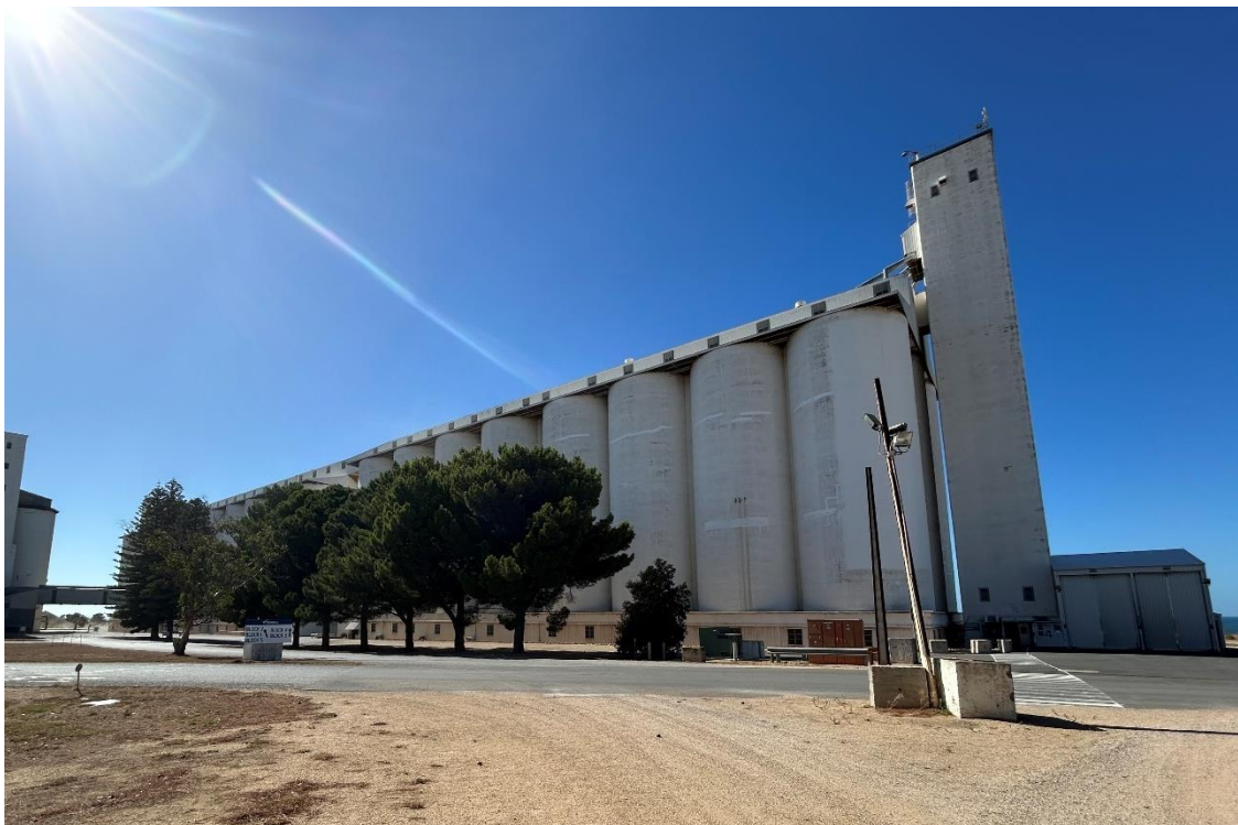
24-cell and 36-cell concrete vertical silos at Ardrossan.
