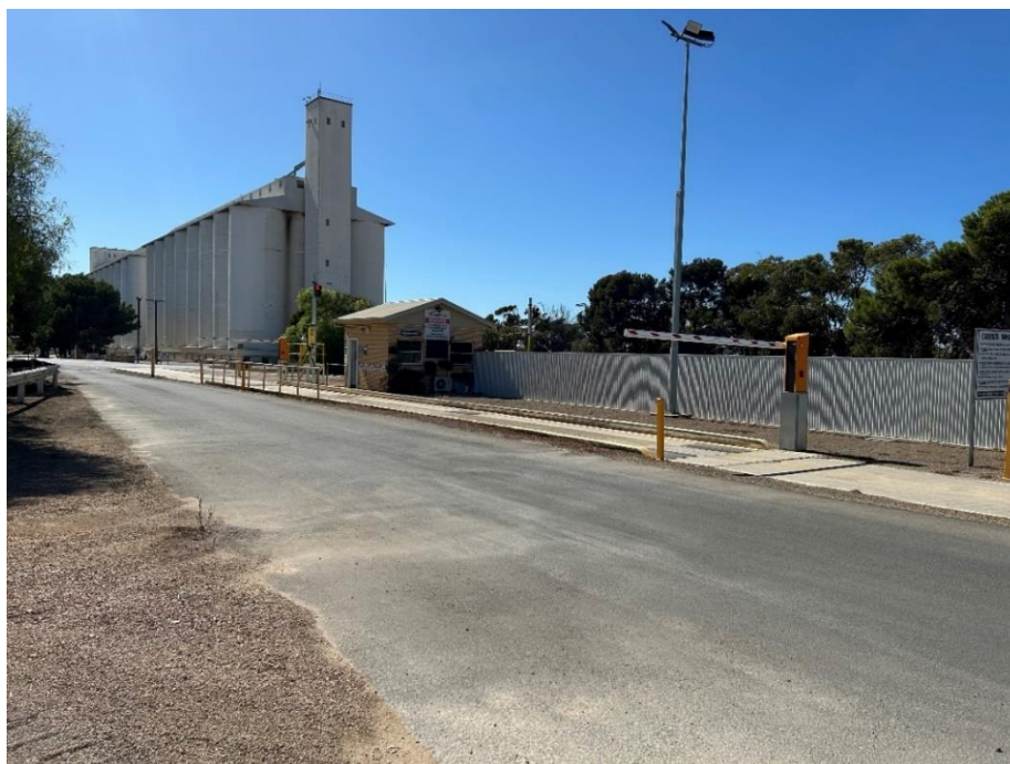
The northern weighbridge with concrete vertical silos in the background.
