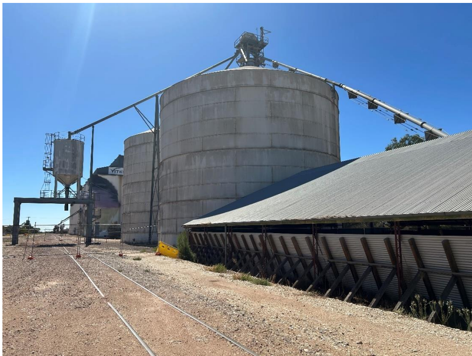
The gravity chute connecting the steel vertical silo with the horizontal shed silo.
