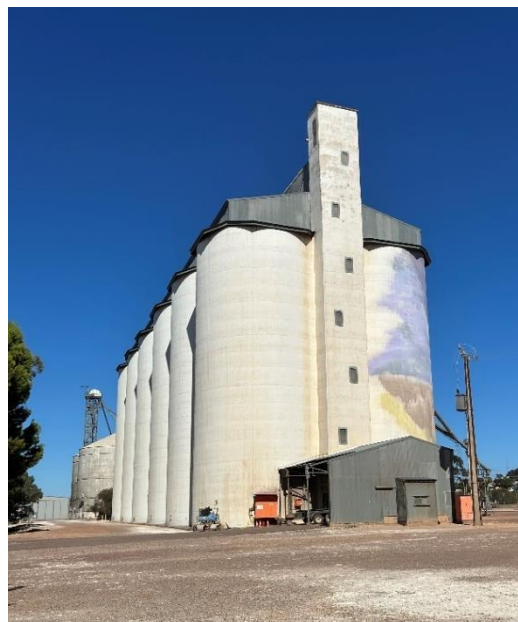
A direct cell outloader (left) and the southern elevation of the southern concrete vertical silos (right).
