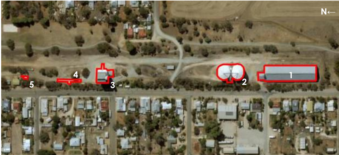
Aerial view of the Brinkworth Bulk Grain Handling Complex showing main elements.
