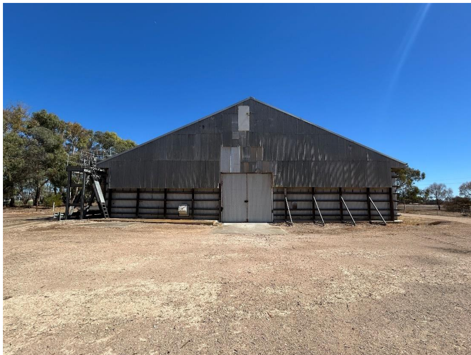
Eastern elevation of the horizontal shed silo.
