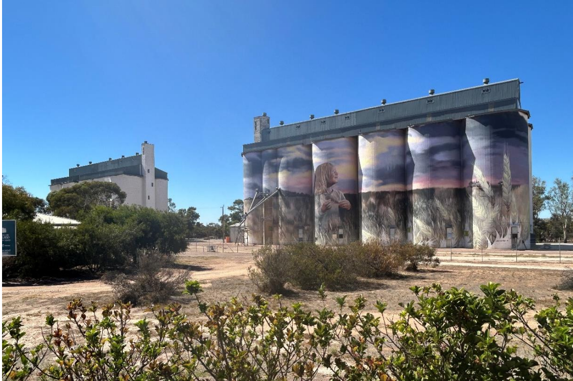
Kimba Bulk Grain Handling Complex.
