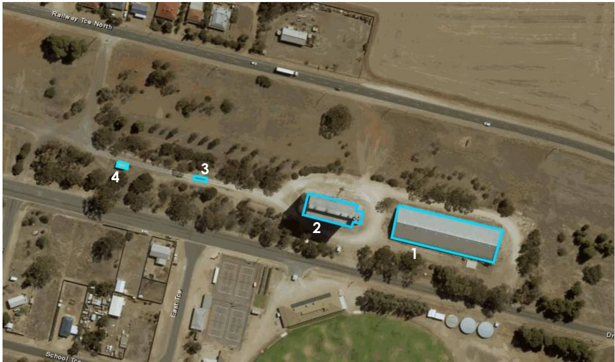
Aerial view of the Paskeville Bulk Grain Handling Complex showing main elements.
