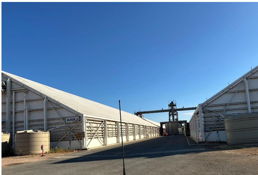
Southern elevation of paired sheds with shared receive hopper and elevator.
