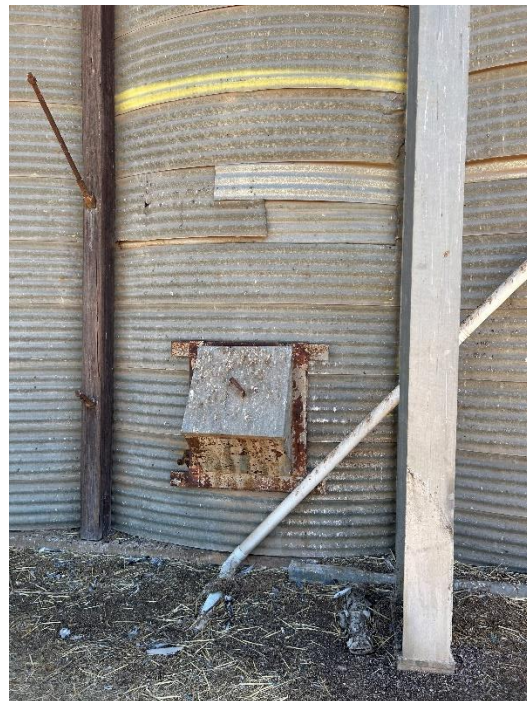
Switchboard, grain elevator tower and receival hopper (left) and detail of the curved corrugated steel walls with direct cell outloader (right).
