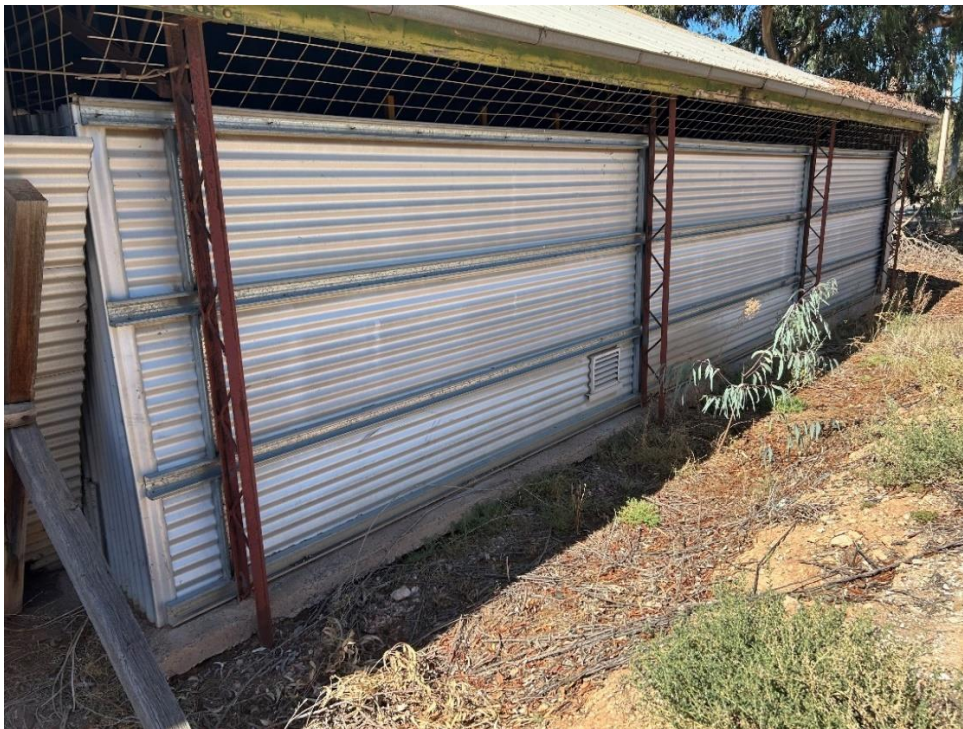
Southern end of horizontal shed silo.
