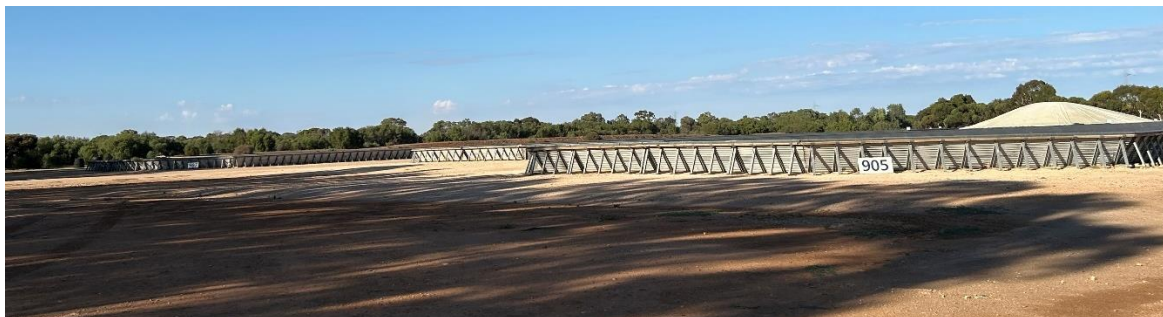
Bunker storage looking west.
