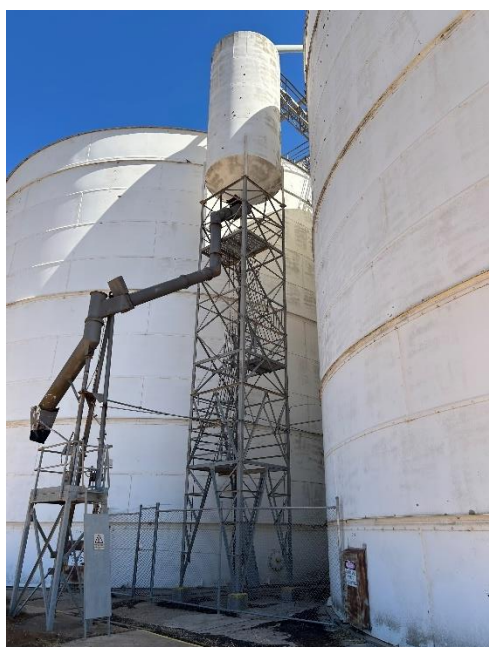
Unloading bin and unloading chute (left) and receive hopper enclosure (right).
