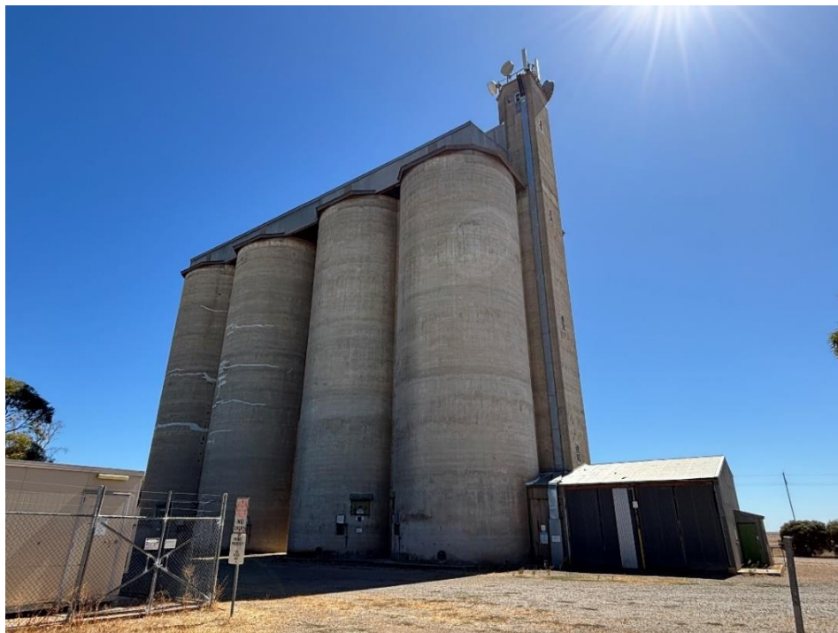
The concrete vertical silo at Paskeville.
