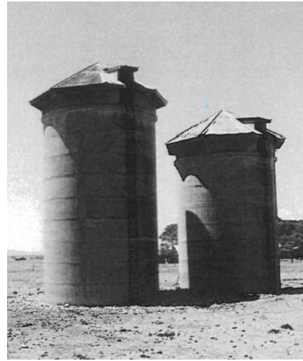
Pair of vertical concrete silos built in South Australia at Gumville Station, Melrose in 1919 (SHP 16242).
