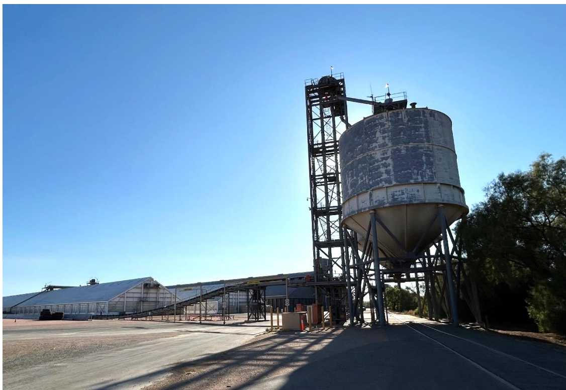
Conveyor belt system connected to railway outloading bins.
