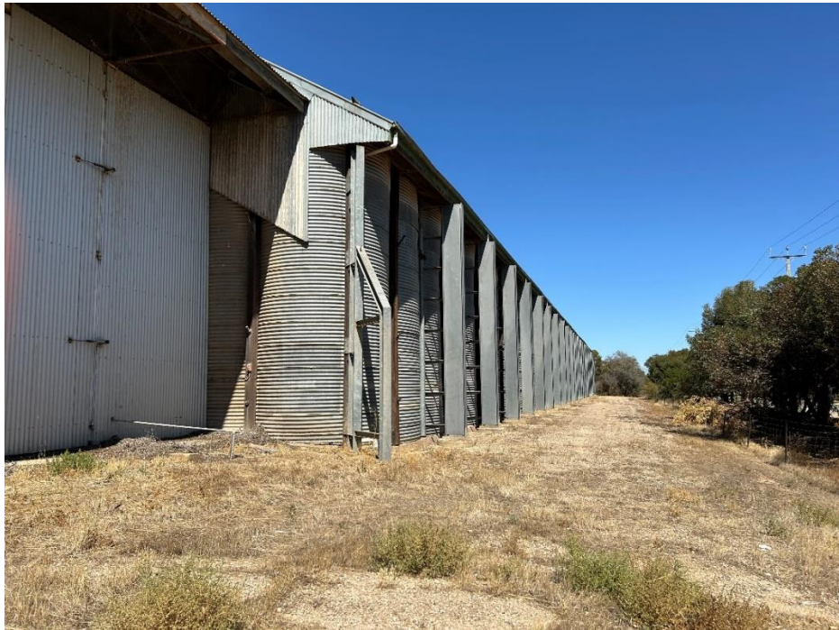
Eastern elevation of the horizontal shed silo showing external reinforcement columns.
