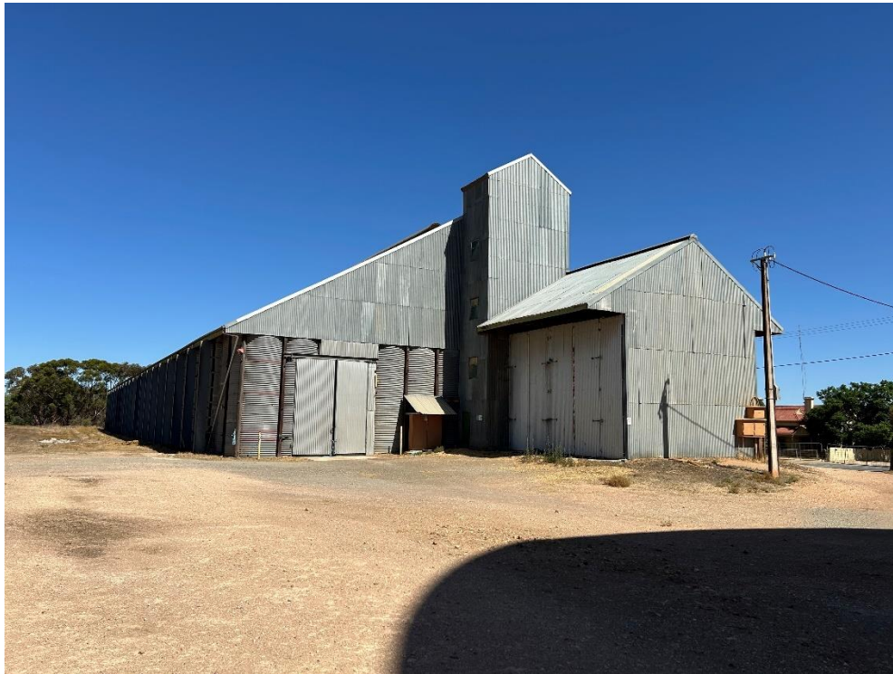
Northern elevation of horizontal shed silo.
