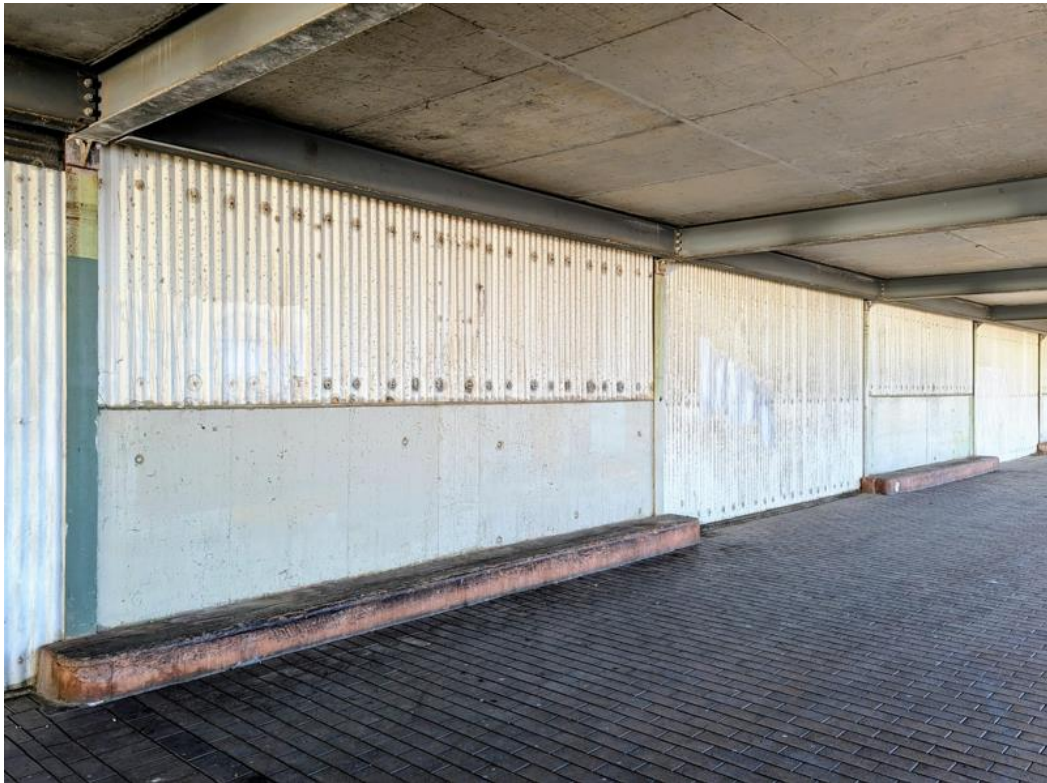
Figure H. Wharf side view (under balcony) showing original concrete kerbing which was located between original sliding door openings (June 2025 photographer [REDACTED])
