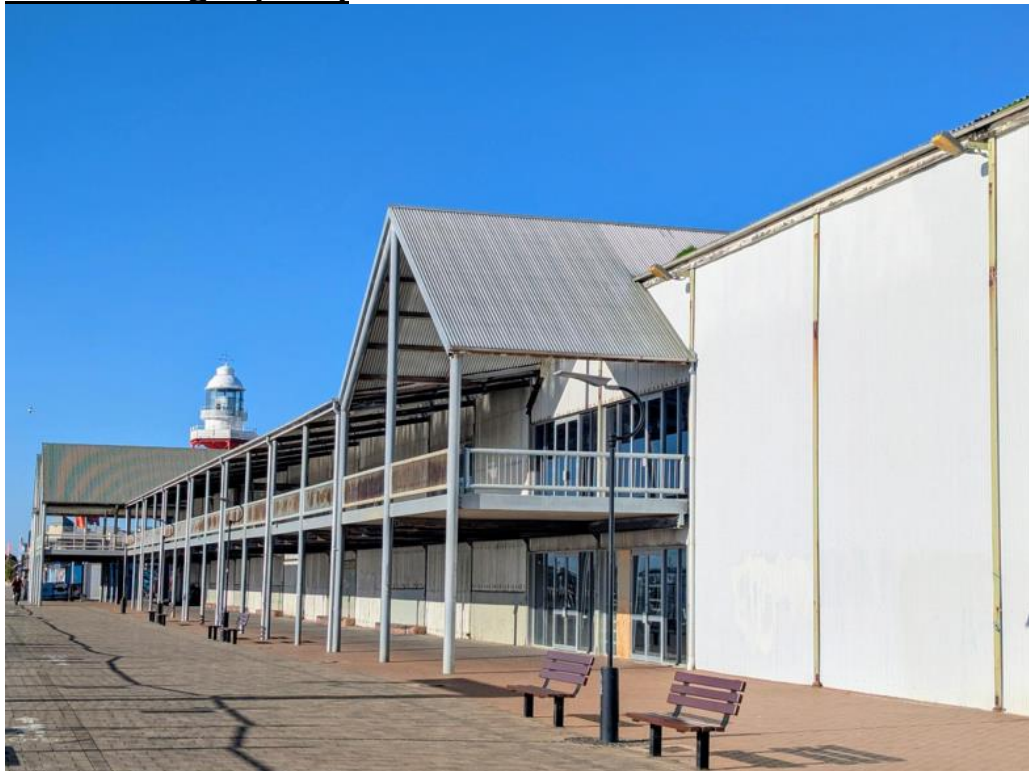
Figure G. Wharf side view showing the added verandah (locations A in foreground, and C to rear – refer Figure B. New roofing is steel One line of colour paver 'rail line' on the left (June 2025 photographer [redacted])
