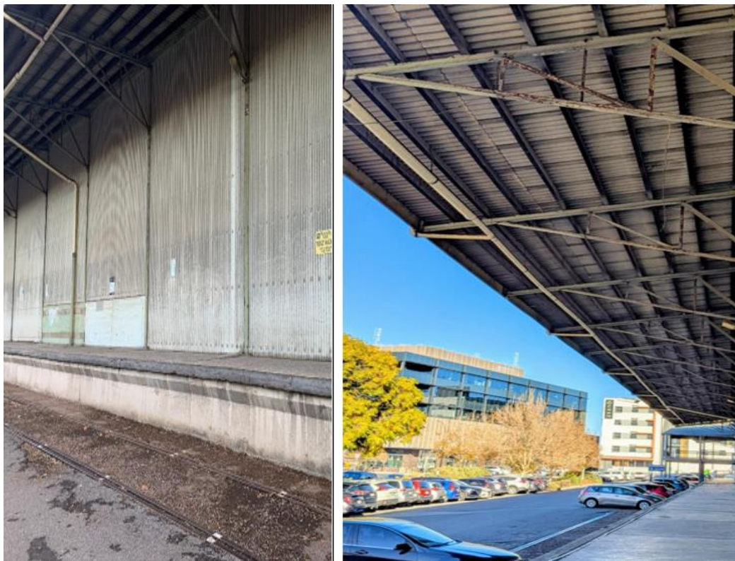
Figure K. Landside of shed showing elevated loading apron (11ft 3"), rail tracks and the original overhead verandah detail (June 2025 photographer [redacted])
