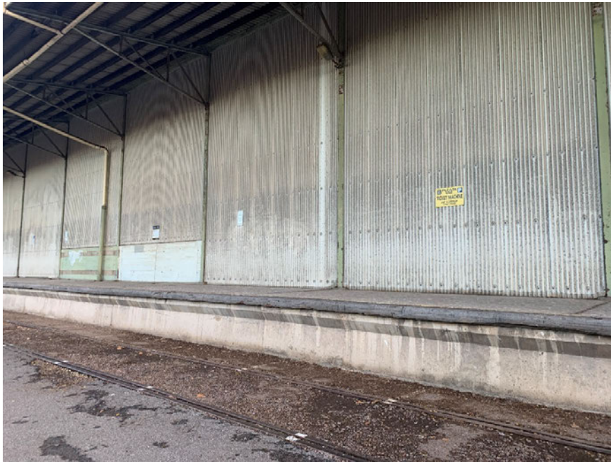
Figure 5 South Face of former Cargo Shed #1 showing elevated rail car loading apron and original tracking. Photo June 2025
