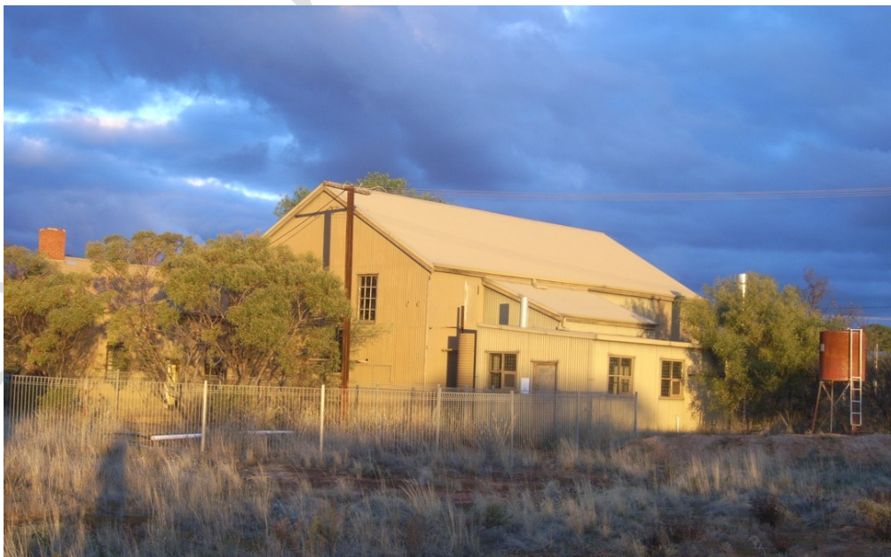
Exterior of battery shed, showing lean-to additions on western side.
