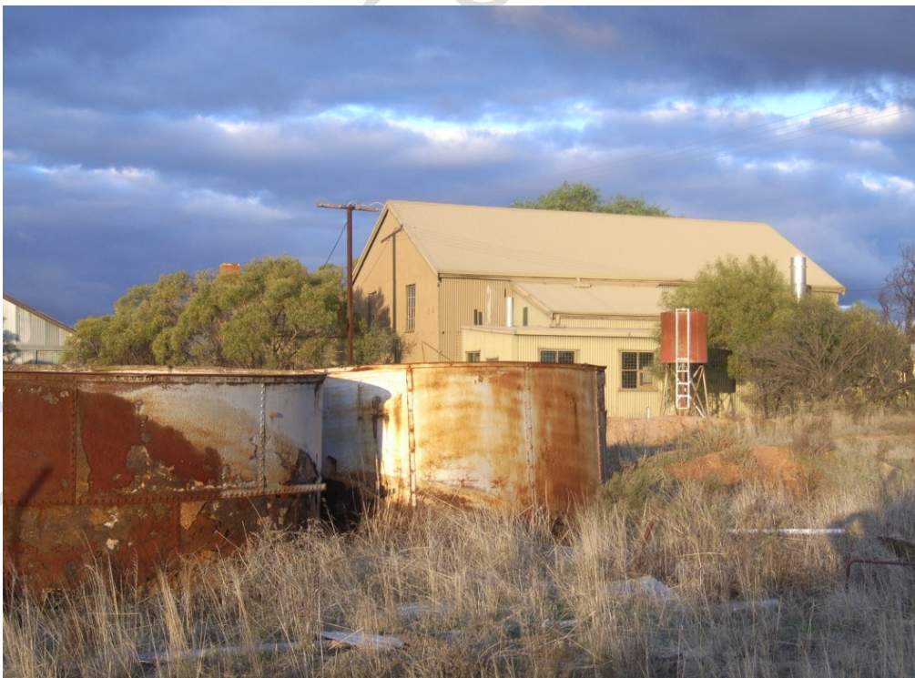
Western side of battery shed; note iron tanks associated with cyanidation plant (moveable components) in left foreground.
