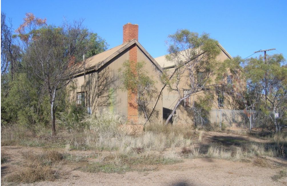
Office building on left; note brick chimney.
