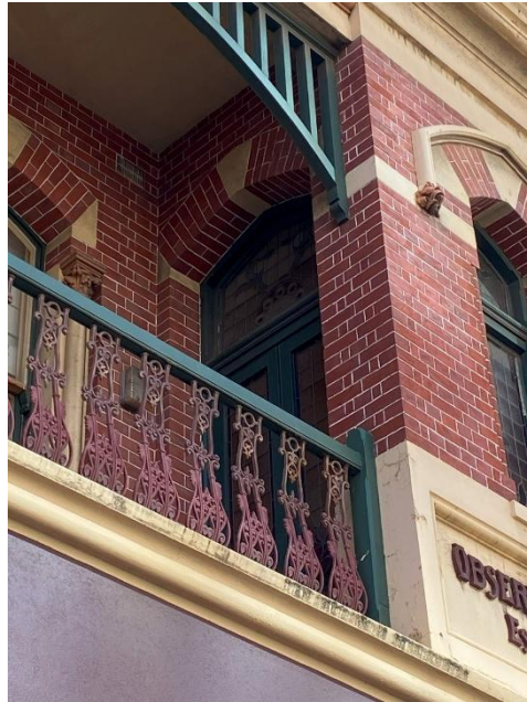
Fanlight and French doors leading to balcony, located on eastern and western side of lower section of first storey.
