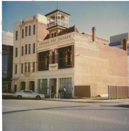
Observatory house c.1982-1985. Note signage on eastern elevation now covered by adjacent building.
