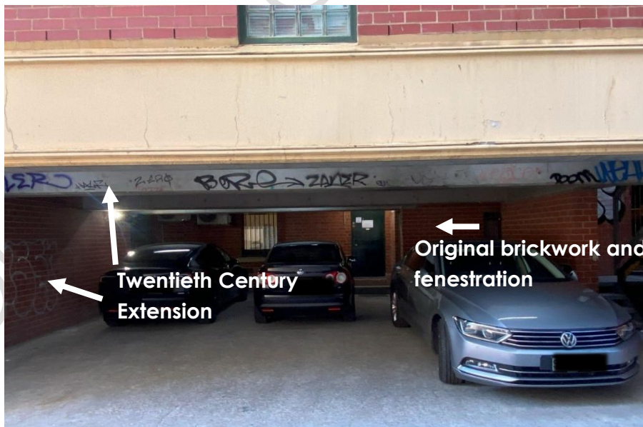
Rear of building, note original brickwork and fenestration.
