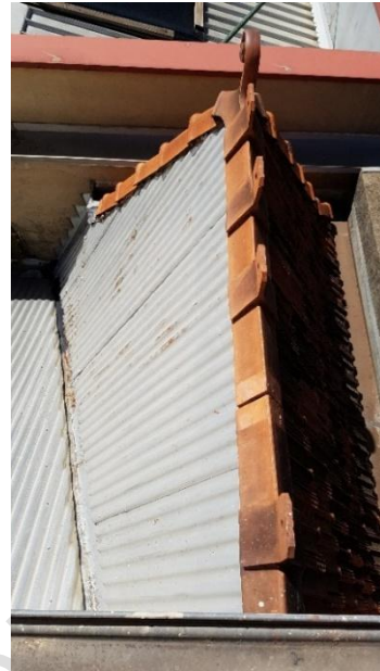
Portion of hipped roof with terracotta tiles, decorative capping, ridging and finial on southern elevation, and galvanised steel on northern side.
