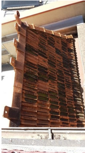
Portion of hipped roof with terracotta tiles, decorative capping, ridging and finial on southern elevation, and galvanised steel on northern side.
