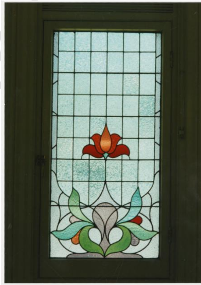
Portion of window holding leadlight, as seen from interior of building.
