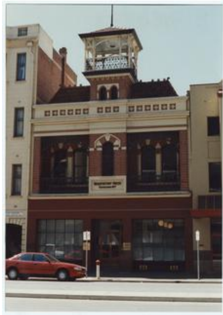
Southern elevation of Observatory House c.1999
