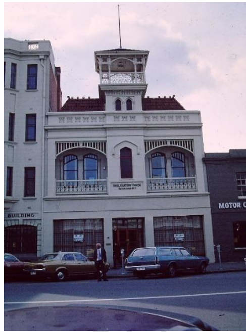
Southern elevation of Observatory House c.1970s Note the altered fenestration at ground level and painted facade.
