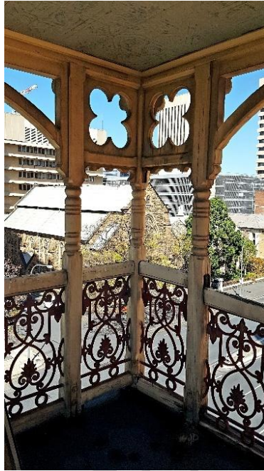
View of north-western corner of belvedere. Note the iron balustrade, timber joinery, decorative fretwork and pressed metal ceiling.
