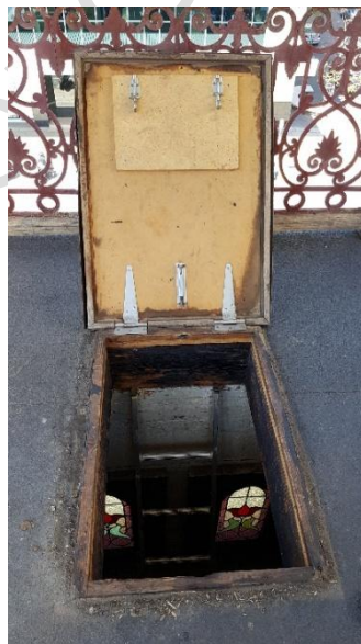
Door to access belvedere.
