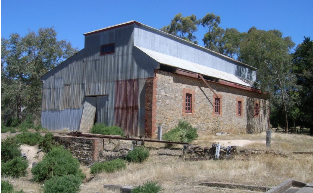
Store, viewed from the northwest.
