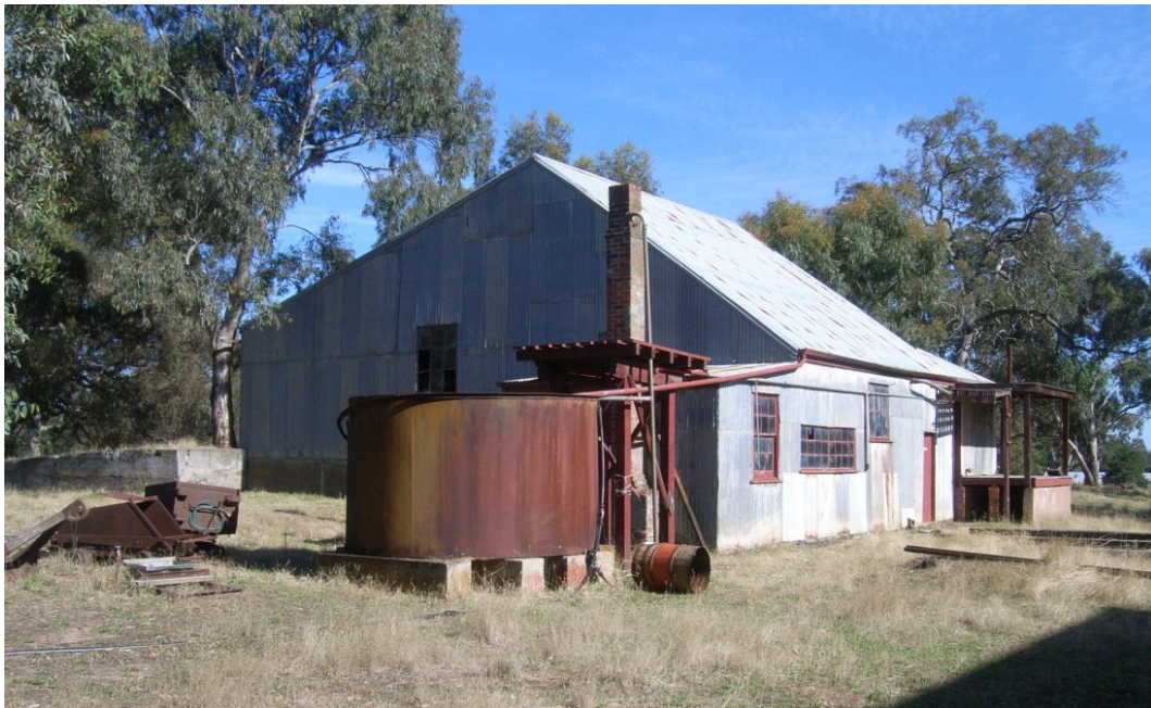
Battery shed, view from south.
