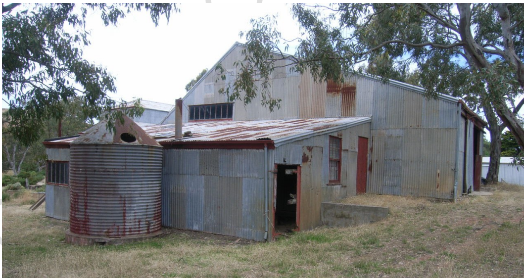
Battery shed viewed from north.
