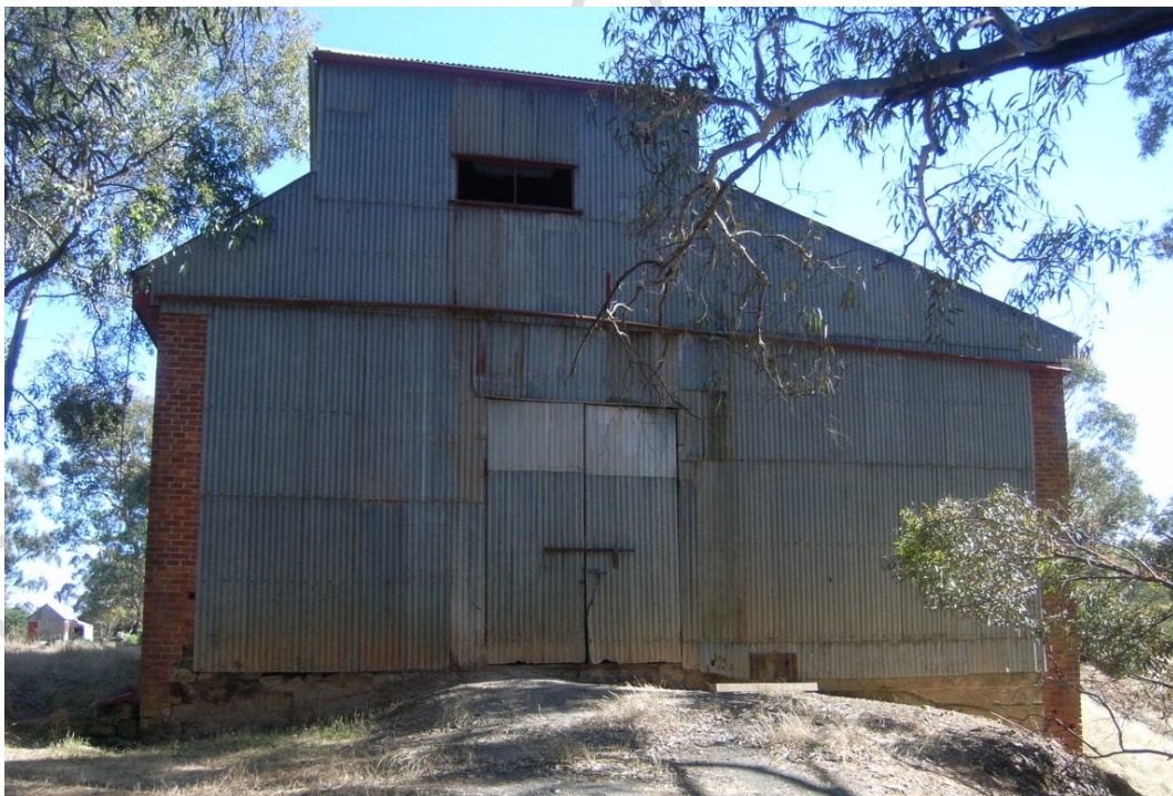
Store, viewed from the south.
