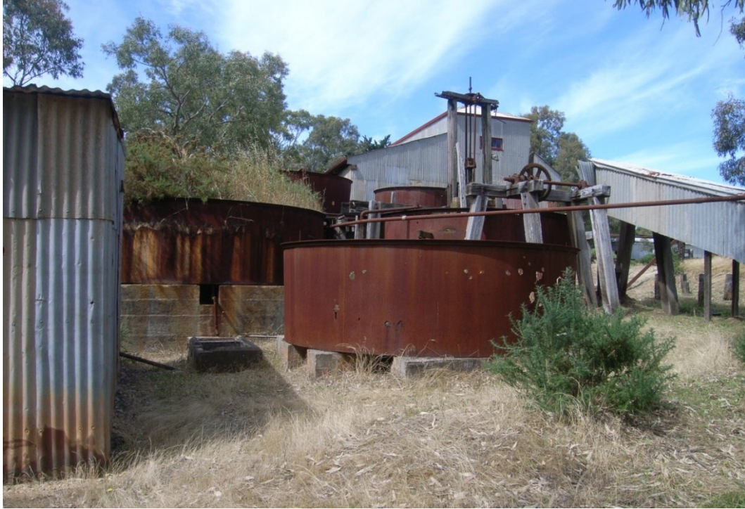
Western cyanidation plant, viewed from north.
