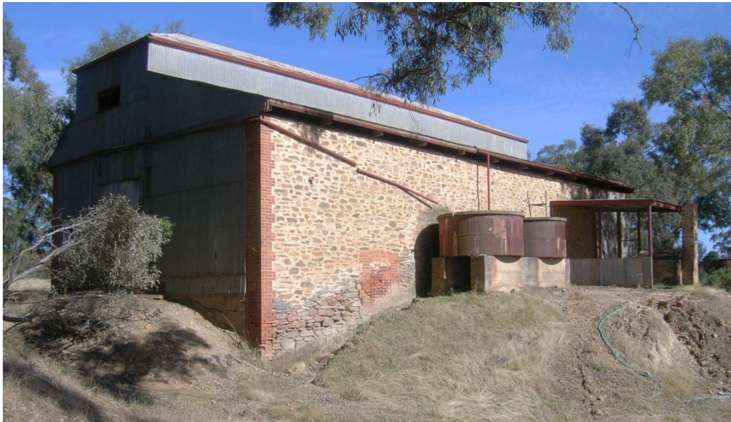
Store, viewed from the southeast.
