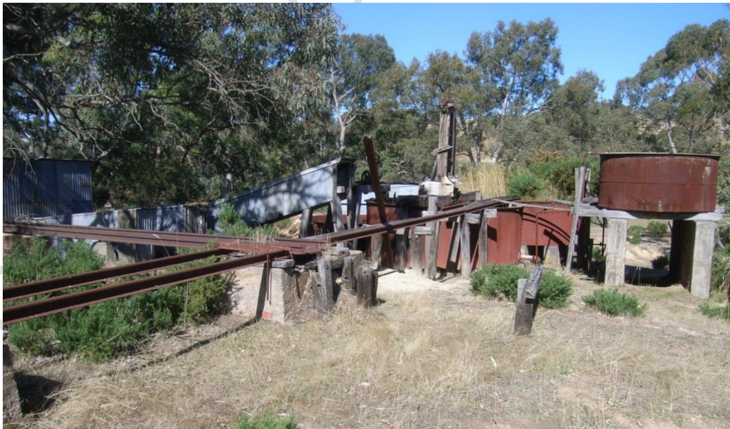
Western cyanidation plant, viewed from west.
