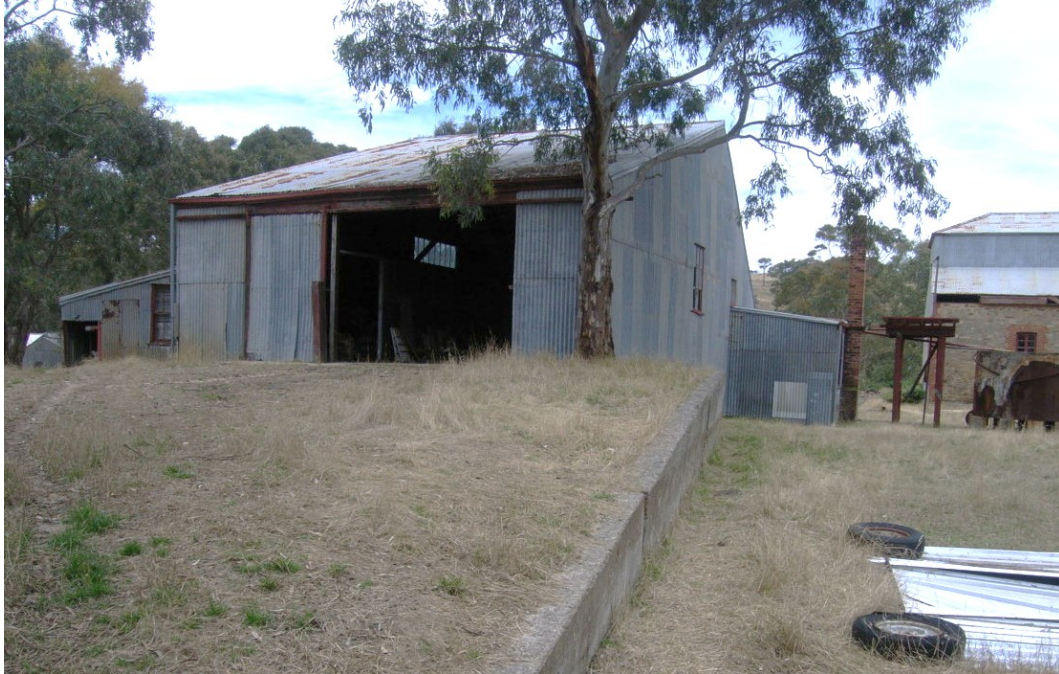
Battery shed viewed from the west, note earthen ramp and retaining wall in foreground, covered weighbridge pit on right.
