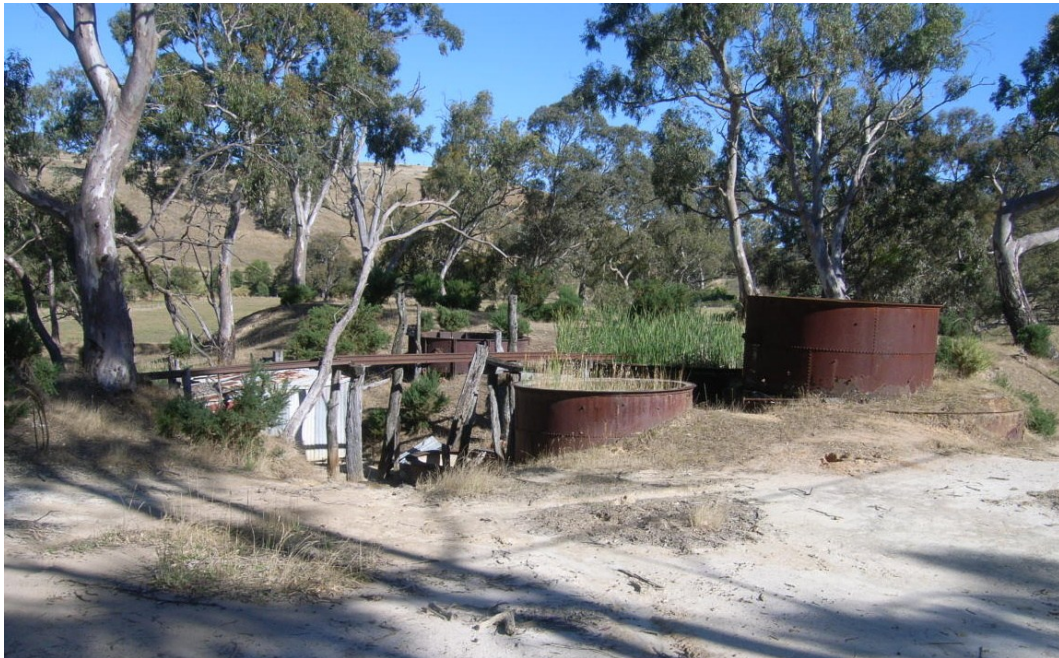
Eastern cyanidation plant, viewed from west.
