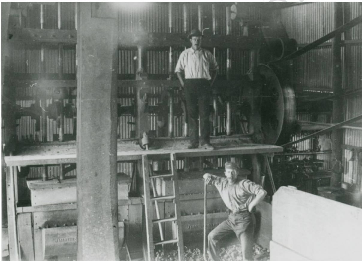
Stamp battery and operators at the Arltunga Cyanide Works, NT, c.1898.
