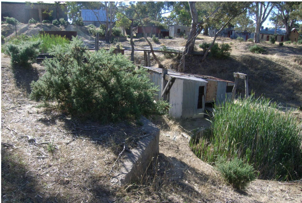
Eastern cyanidation plant, viewed from east.
