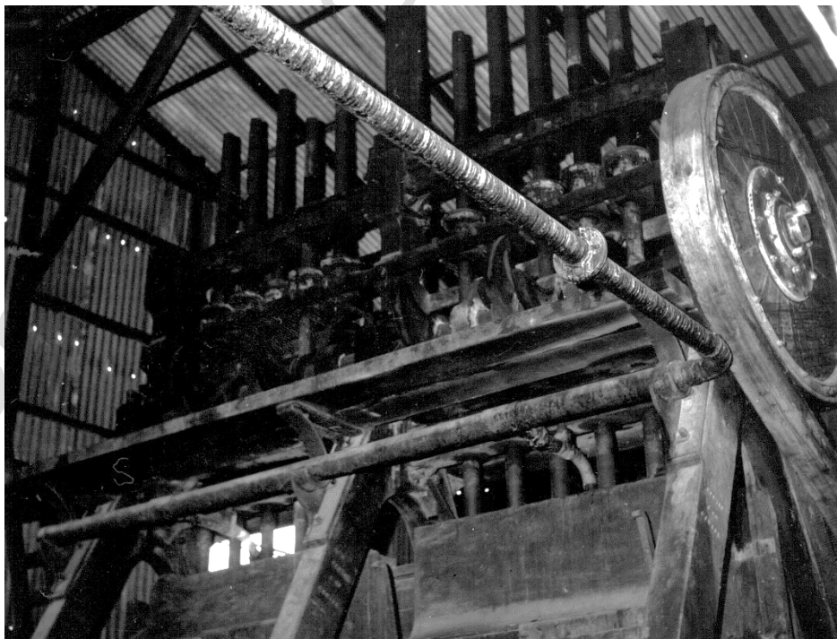
Stamp battery plant (built 1889, relocated 1935–1936), March 1985.
