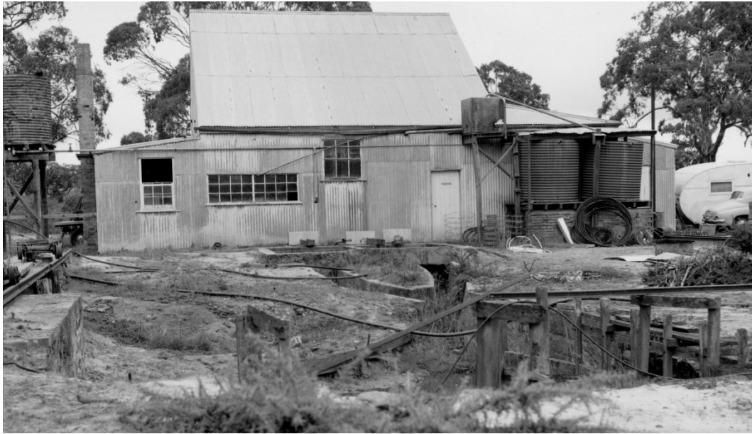
Battery shed with part of new cyanide works in foreground (both built 1935–1936), March 1985.
