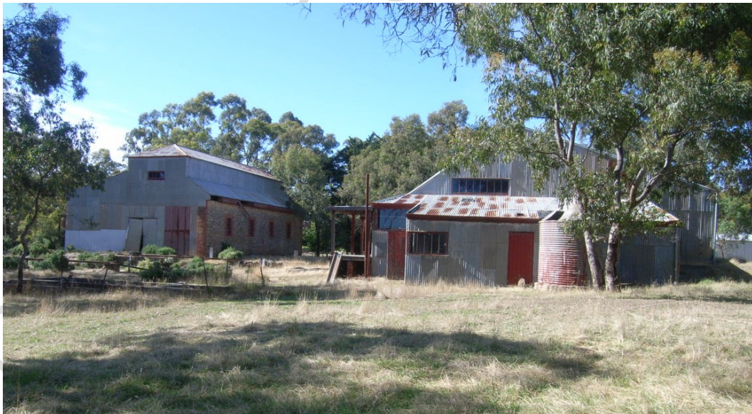
Store (left) and battery shed (right) viewed from the north.
