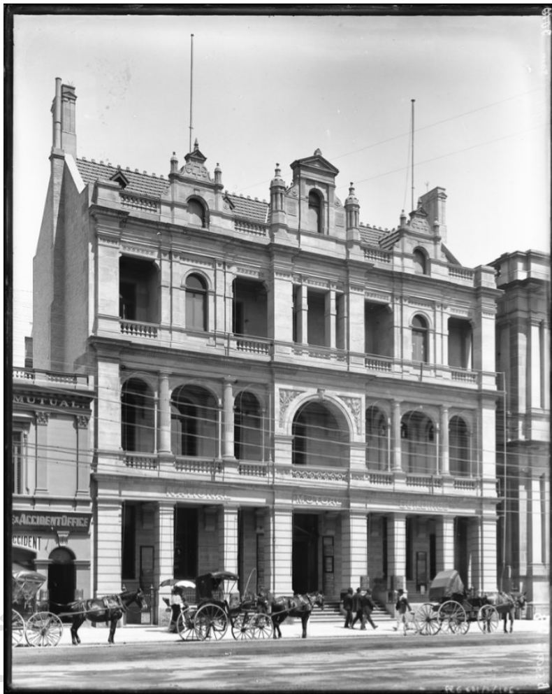
The recently-completed National Mutual Life Association Office Building, 1901.
