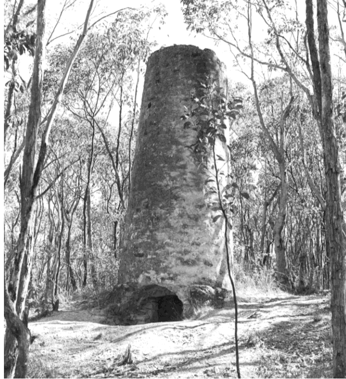
Circular stone chimney built in 1869 by the Beatrice Mining Company, January 1983.
