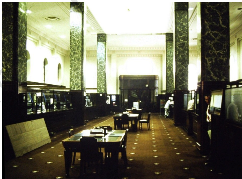
Banking chamber interior, January 1982.
