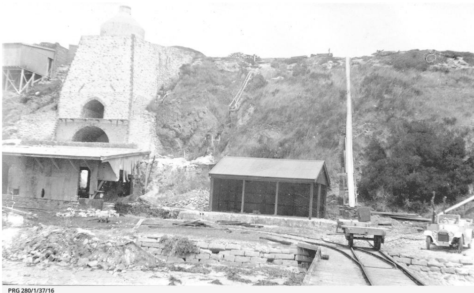
Lime Kiln in Wool Bay, 1923. Note the associated structures, such as the packing and storage shed, shoot, tramway and front working area with associated structure, since demolished. Some foundations of associated structures remain.
