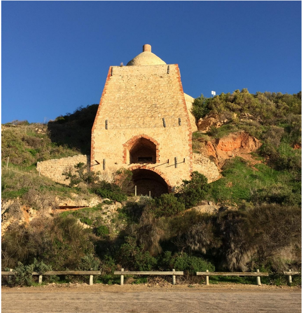
Wool Bay Lime Kiln and Jetty SHP 10112, 28 June 2015.
