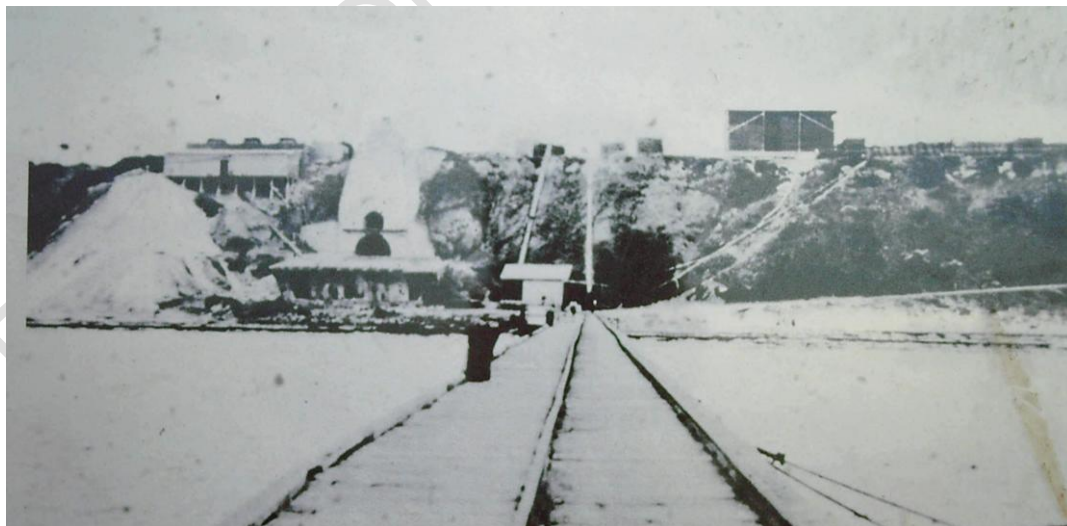
Wool Bay Lime Kiln and Jetty looking west, date unknown. The tops of three smaller lime kilns can be seen to the left of the image. Associated structures from the grain industry can also be seen such as the grain shed to the right of the image. A tramway can be seen on the jetty.
