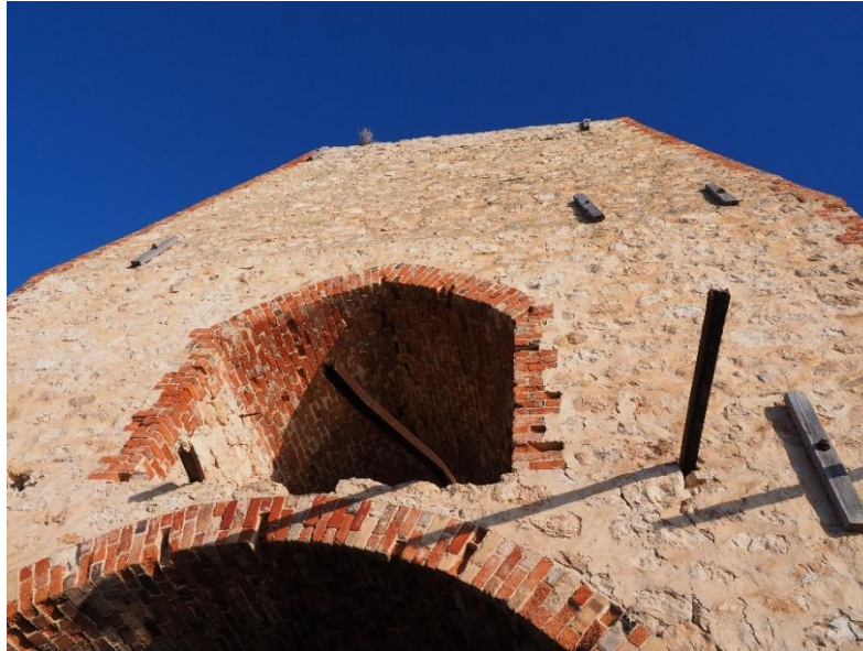
View of upper vault on eastern elevation. Note the tie rods as well as cantilevered joists which once supported a platform to access the upper vault.
