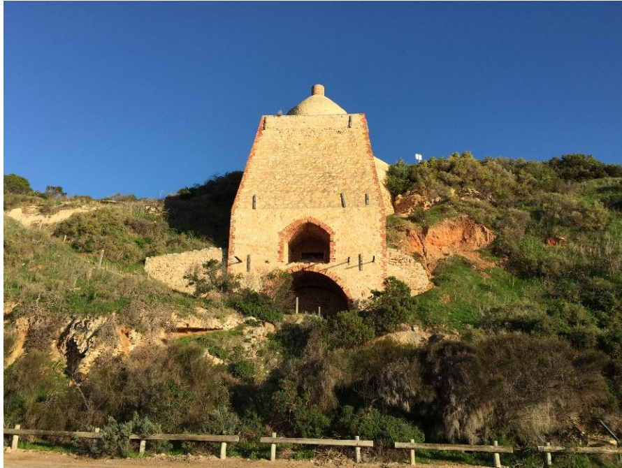
Eastern elevation of lime kiln, note rebuilt dome and chimney.
