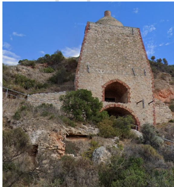
View of lime kiln looking west, March 2024. Note the remaining rubble limestone foundation of the kiln's working area in front of the kiln.
