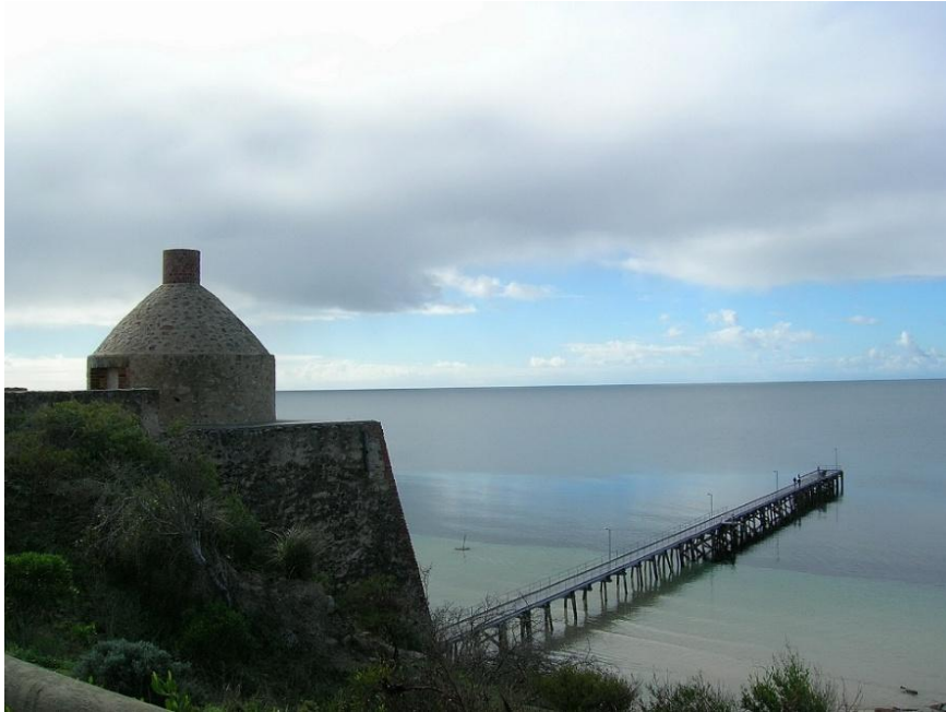
View of lime kiln and jetty, looking north-east. Note the spatial relationship between the lime kiln and jetty.
