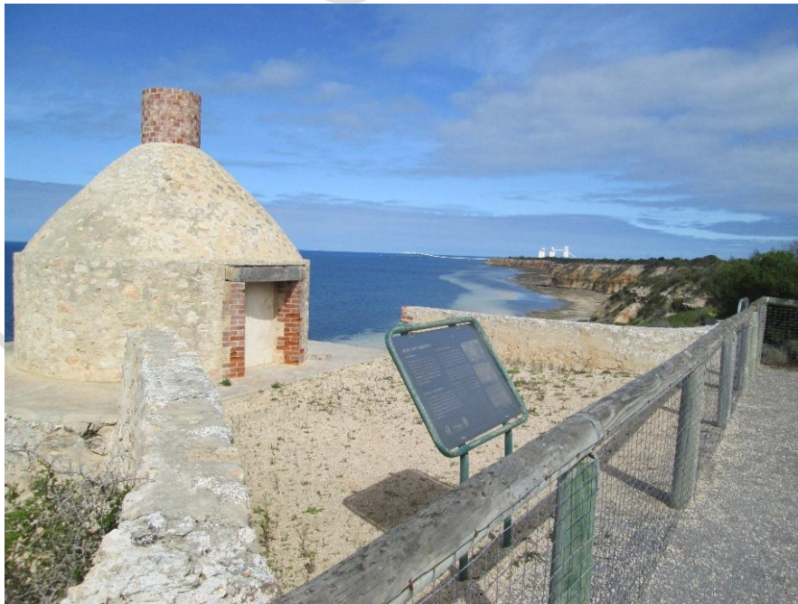
Western elevation of lime kiln, featuring the reconstructed dome and chimney. The wing walls can be seen on either side.
