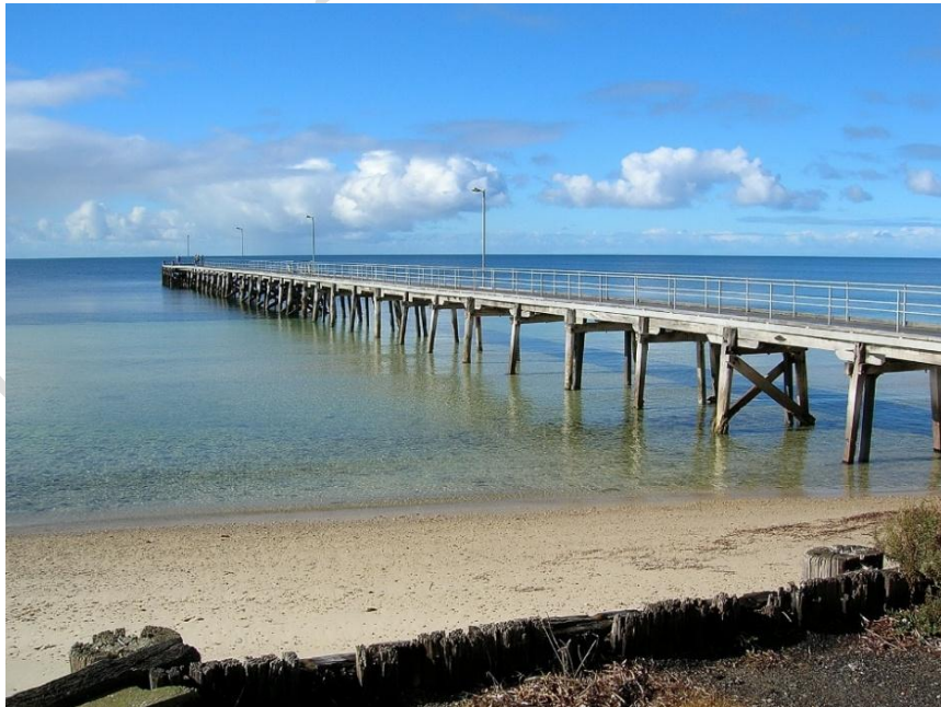
View of jetty. Note cross bracing to one of the bents, and the addition of a third steel pile to some of the bents on the right side of the image.
