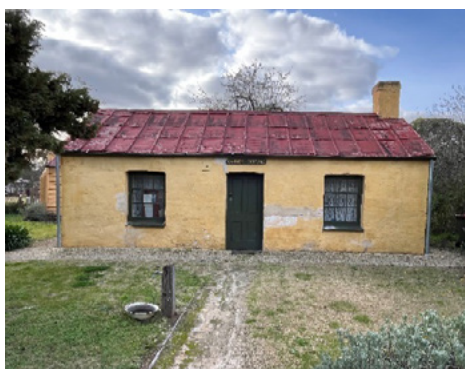
Gammon Cottage (1880s), showing early construction methods including metal tile roof, DEW 2024
