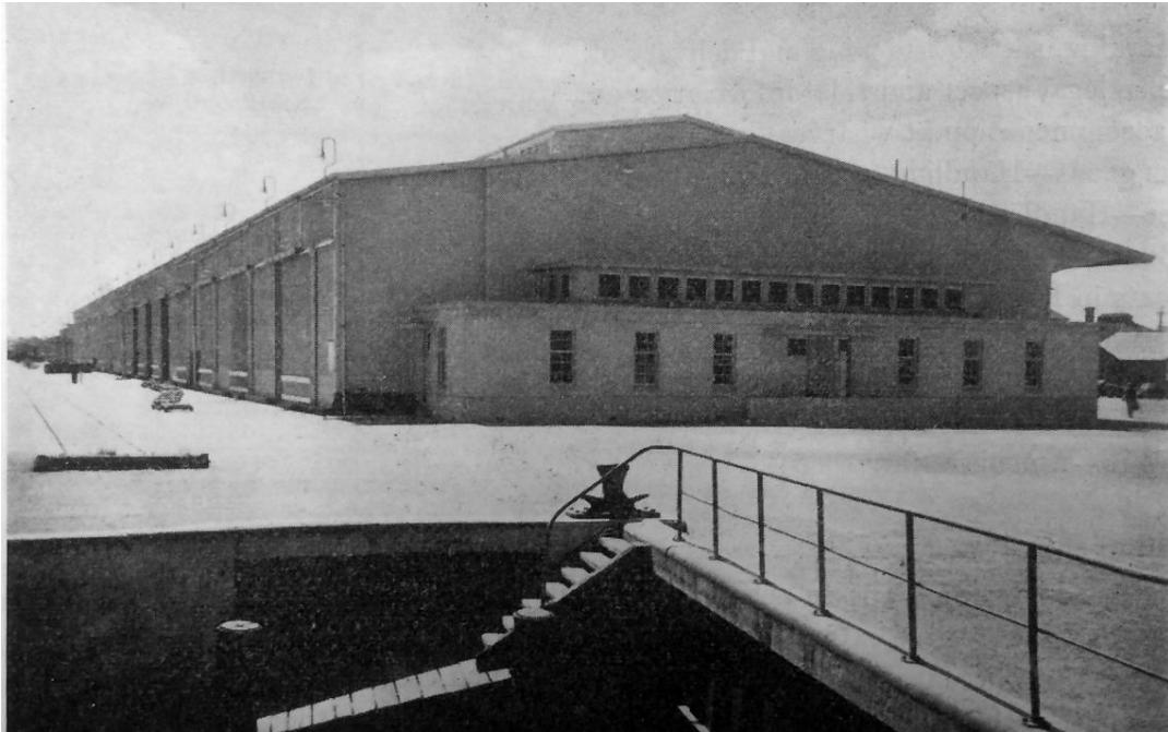
Plate 13: Cargo Shed No. 1, at completion. (1953)(SAHB Annual Report, 1953)
