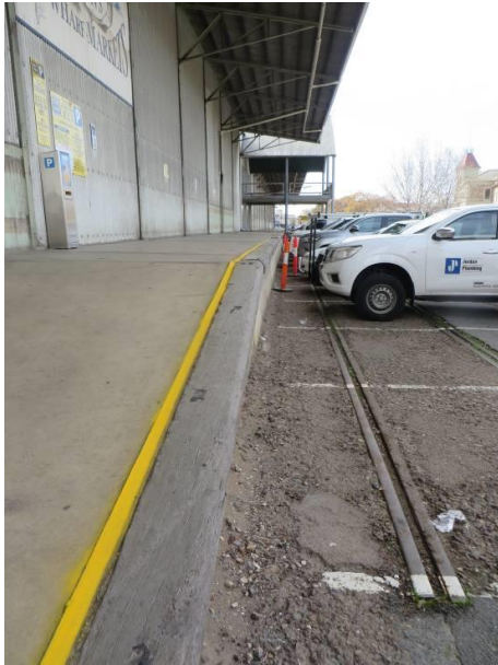
Photo 3: Cargo Shed No. 1, looking east, showing apron roof over the elevated loading platform and surviving rail lines. (Stephen Schrapel, 2016)
