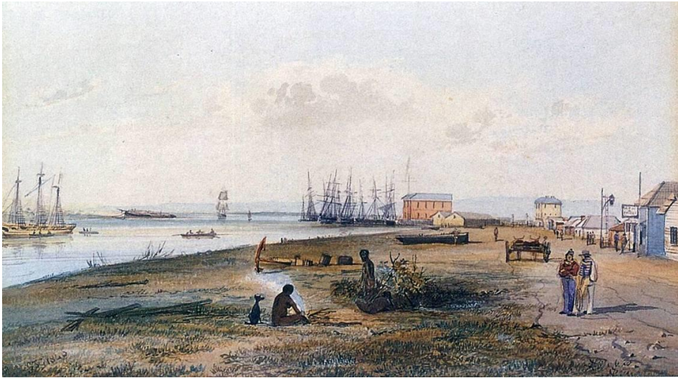
Plate 1: Port Adelaide looking east along North Parade by S T Gill. The SA Government Sheds are the gabled ended structures in the background, beyond which are the two-storied SA Company warehouses. [Watercolour on paper (1846), Art Gallery of South Australia, gift of B W Baganal, 1941]
