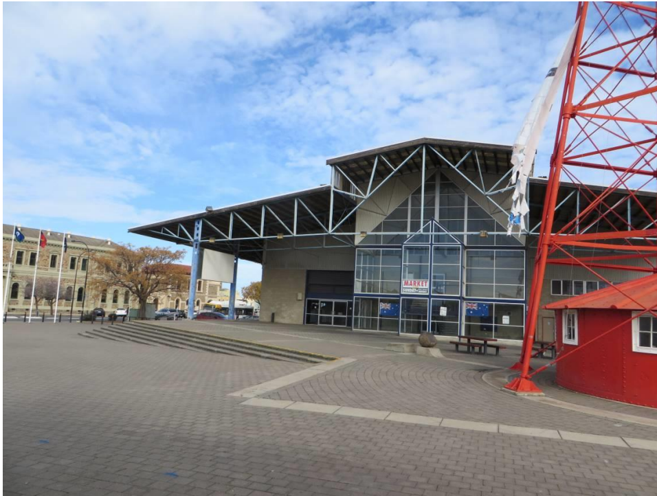
Photo 1: East end of Cargo Shed No. 1, looking west (Stephen Schrapel, 2016)
