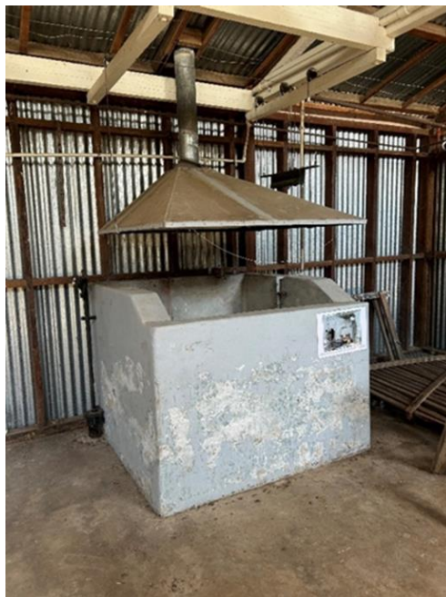
Image: The linen sterilizer located within the laundry block. Source: DEW files.
