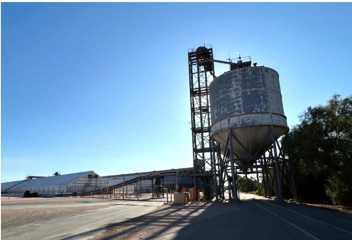
Image: Conveyor belt system connected to railway outloading bins.
