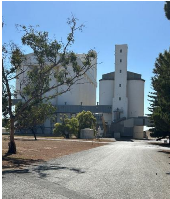
Image: The 21-cell and 16-cell concrete vertical silos at Ardrossan. Source: DEW Files.
