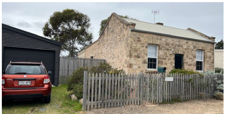
View showing two successive lean-to additions built to the rear of a cottage in “Little Scotland”. DEW 2024
