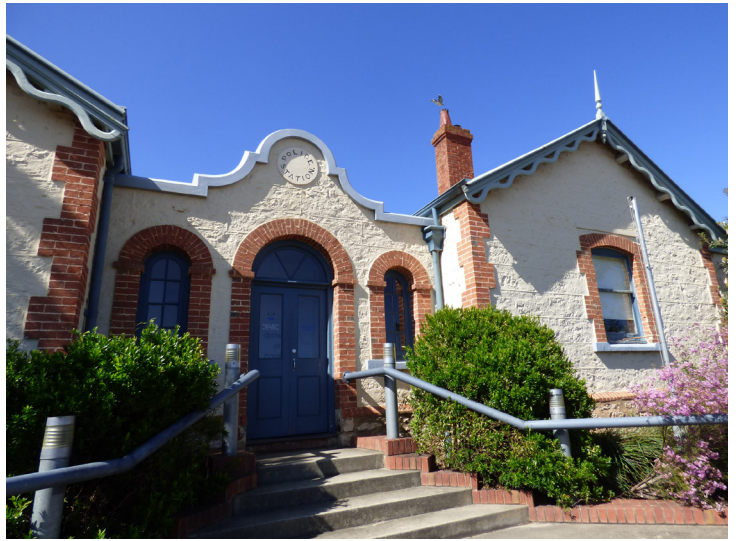
Police Station and Courthouse, vertically-proportioned, timber-framed, sash windows and half round fanlight. DEW 2019
