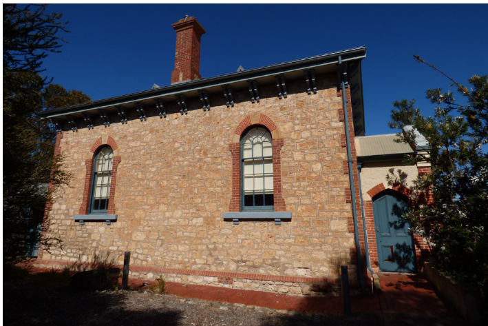
Goolwa Court House, exposed stone wall with brick detailing. DEW 2019
