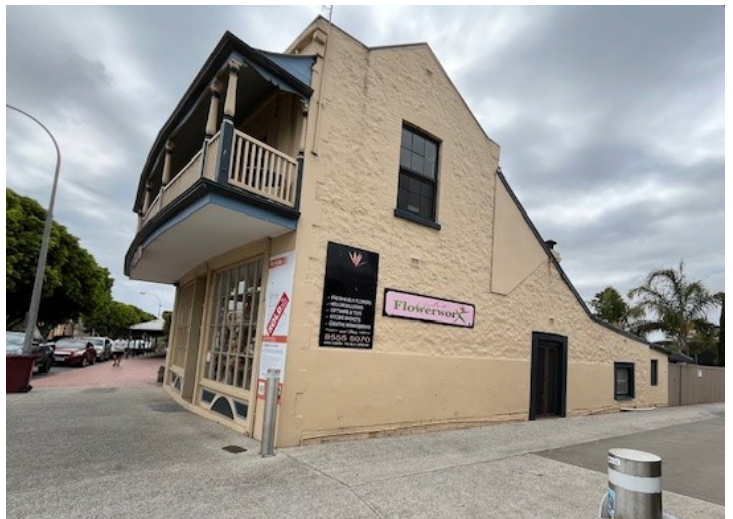
Bow-Fronted Shop, Cadell Street, c.1850s. The front wall of the store follows the allotment boundary, giving a bow-shaped appearance. DEW 2024
