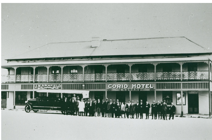
Corio Hotel, showing passengers assembled with an omnibus parked on Cadell Street, c.1920, State Library of SA, SLSA B 17518
