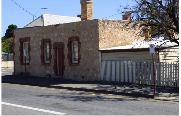
Traditional, weatherboard-clad outbuilding in the “Little Scotland” precinct. DEW 2024
