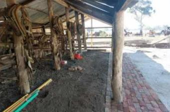
The Clayton Heritage Farm Museum showcases Australian vernacular farmyard technologies and construction techniques ranging from the 1870s to 1930s. Many of the timber posts supporting the stable roof were set directly into the ground and had rotted away, damaged timber was cut out and replaced in matching, compatible timber, and improved stormwater drainage installed.
