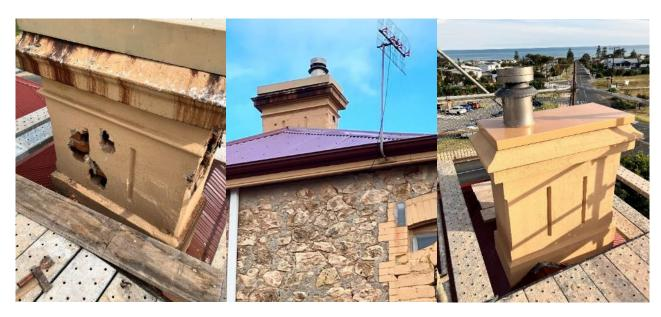
Mindacowie Guest House Chimney Restoration Works – Chimneys were at risk of collapsing; they were removed to a point where the brickwork was solid enough to build up from. The chimneys were taken down below roof height and re-built to their original dimensions. Old red bricks and lime mortar was used to rebuild the chimneys, and they were then rendered using lime render.
