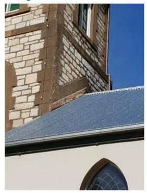
Gruenberg was settled in 1853 by Germans from Hahndorf. The Gruenberg church was built in 1864 with the addition of the tower built in 1914. The church received a grant of \$8,750 in Round 1 of the Program. The funding allowed the roof to be replaced using traditional heritage galvanised iron and the correct roofing techniques. The new roof looks amazing and will ensure this fabulous State Heritage Place will be protected from the elements for many years to come.
