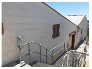
The Kays Brothers winery received a grant of \$10,000 for southern wall restoration including paint removal, removal of hard cement pointing and re-pointing in lime mortar. The Kay Brothers winery in McLaren Vale was originally the Amery Farm established in the 1850s by Richard Baker Aldersey. In 1891, the Kay Brothers, Herbert and Frederick, purchased the farm including 130 hectares. They immediately planted grapes and built the winery which has been in operation ever since.
