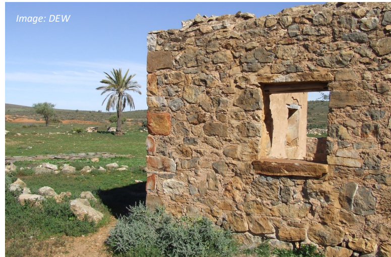
Ruins of the office at Kanyaka Station complex, Quorn (SHP 10192), established 1852
