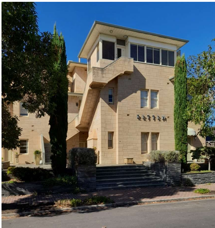
Image: Retten (flats) Source: DEW Files.
