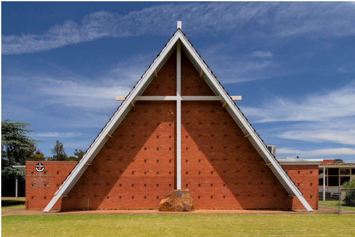
Image: former Salisbury Methodist Church. Source: DEW files.
