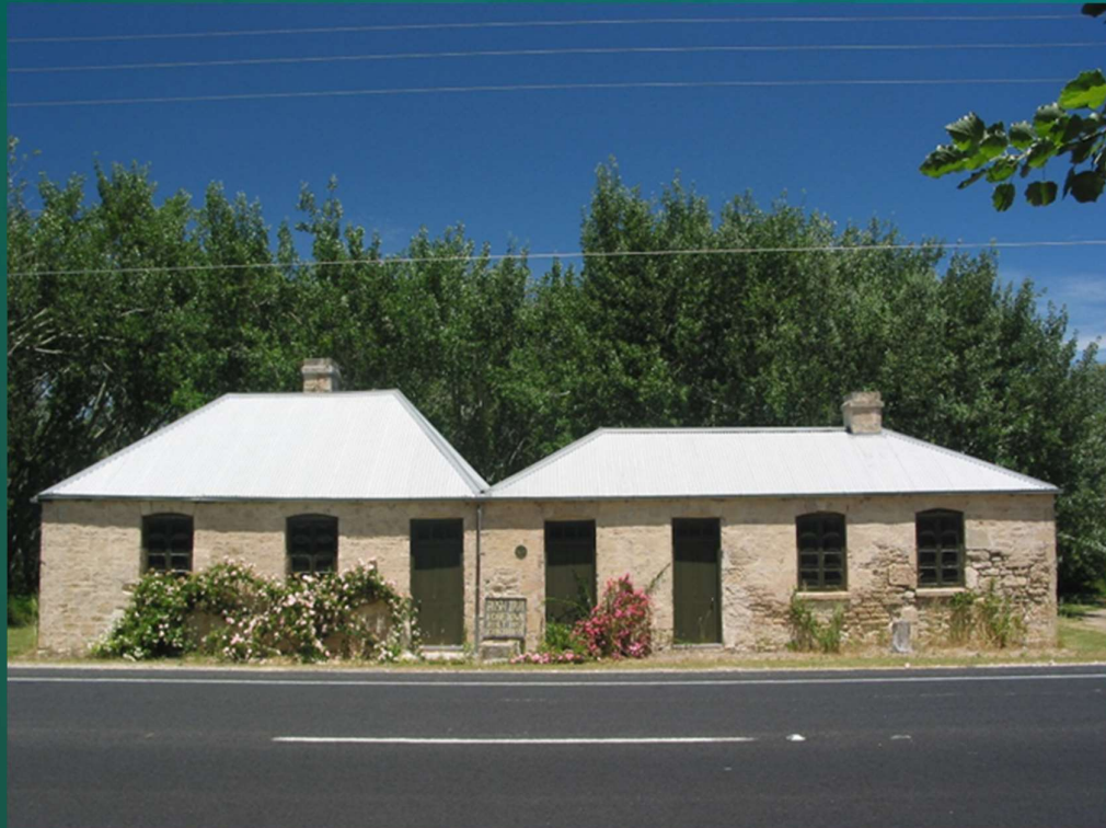
Image: The Bush Inn following conservation works, including repointing, 2003. Source DEW files.
