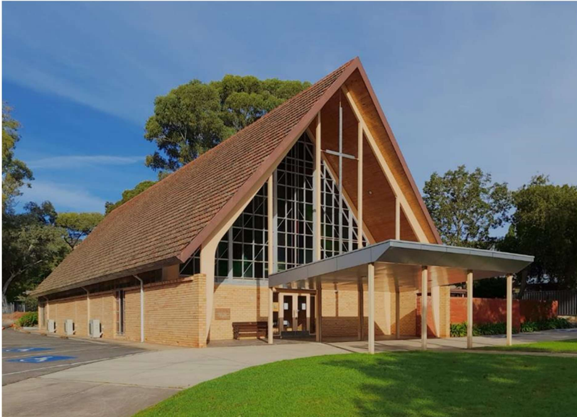
Image: John Vianney's Catholic Church (note carport added 2015). Source: DEW, 11 May 2023.
