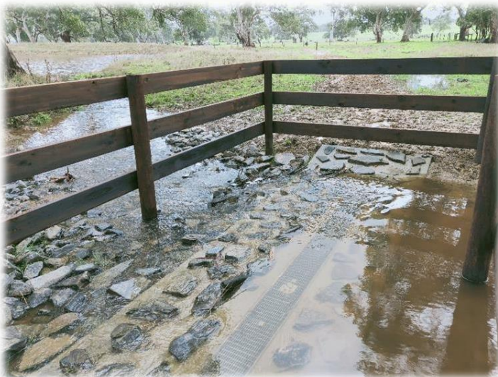
Image above. Gravity device inlet with a low profile sits in the dam inlet.
