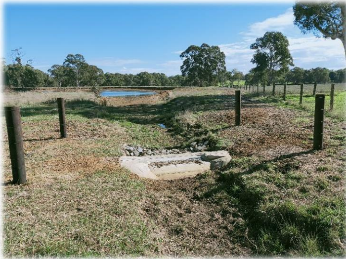
Image above. Gravity device inlet with a low profile sits in the dam inlet.
