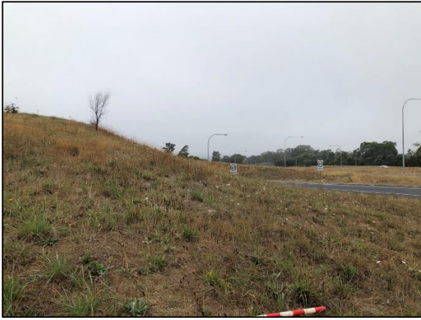
Figure 10. Location CH955, facing east.
