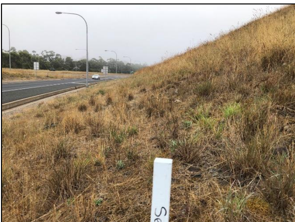
Figure 8. Location CH862, facing west.
