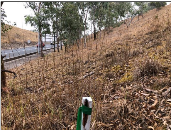
Figure 6. Location CH625, facing west.
