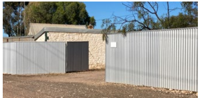
Moonta Mines, stone outbuilding with skillion roof, DEW 2022
