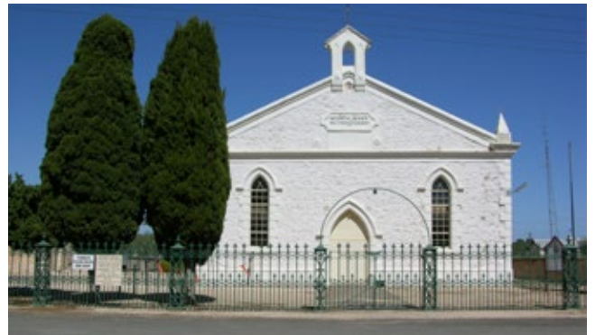
Moonta Mines, former Methodist Church, DEW 2005
