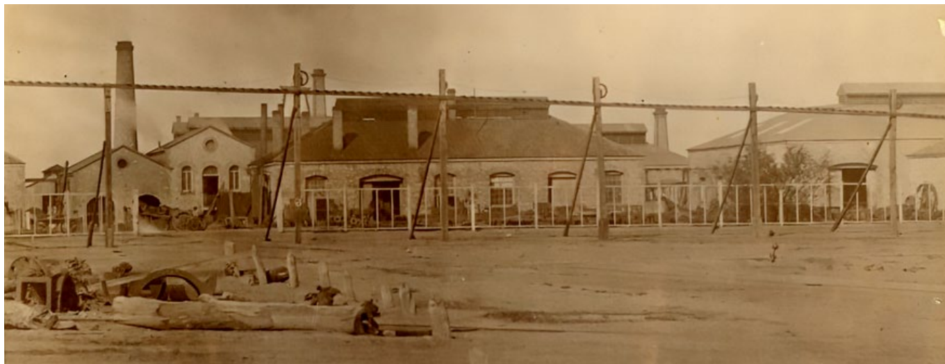
Richman's Engine House, circa 1884, State Library of South Australia, SLSA B 10513.
