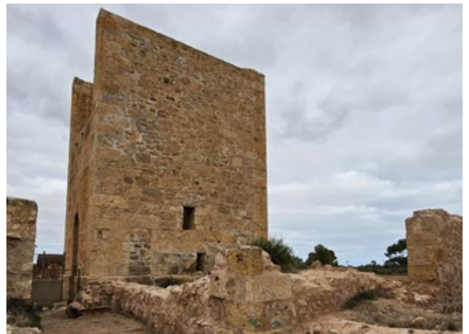
Moonta Mines, Hughes Pump House, stone quoins. DEW 2024
