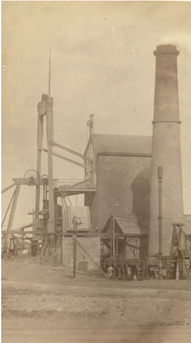
Hughes' Pumping House, circa 1884, State Library of South Australia, SLSA B 10510.
