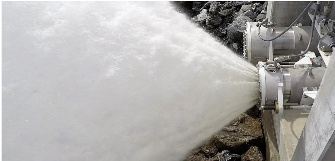
Figure 11 Cone valve diffuser nozzle
