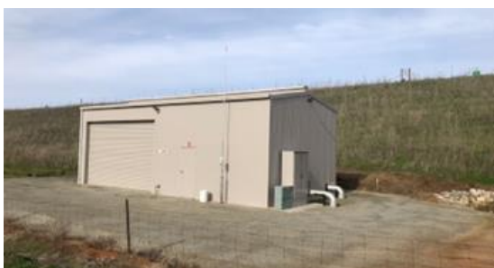
Figure 3.3: Auburn Terra Rossa Embankment
