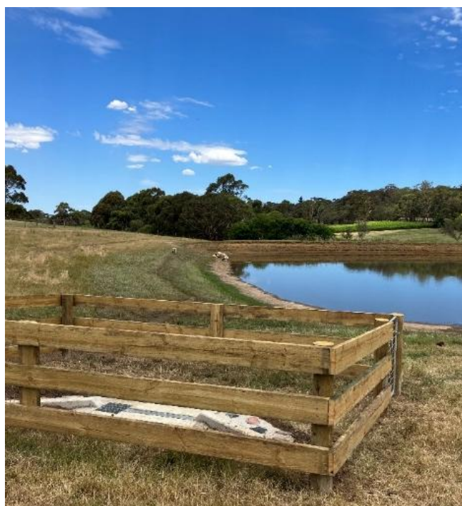
Low flow device installed by Flows for the Future.
