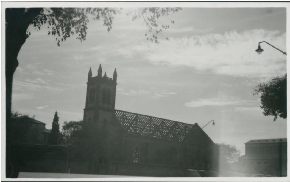
The old St Patrick's Church in the process of demolition, 1959.
