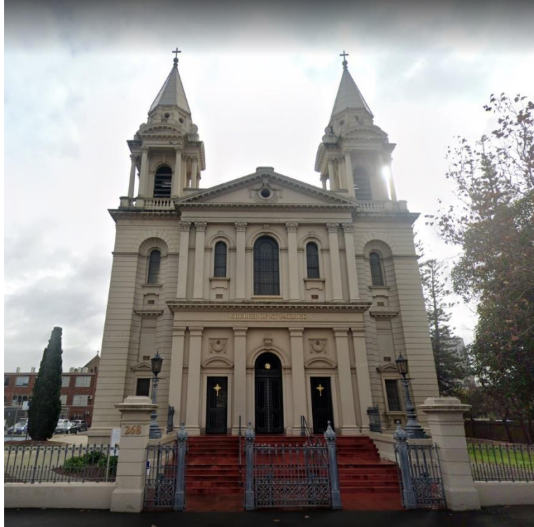
Front elevation of St. Patrick's Catholic Church, July 2023
