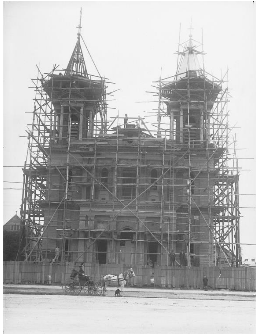
St Patrick's Catholic Church under construction, c.1913-1914
