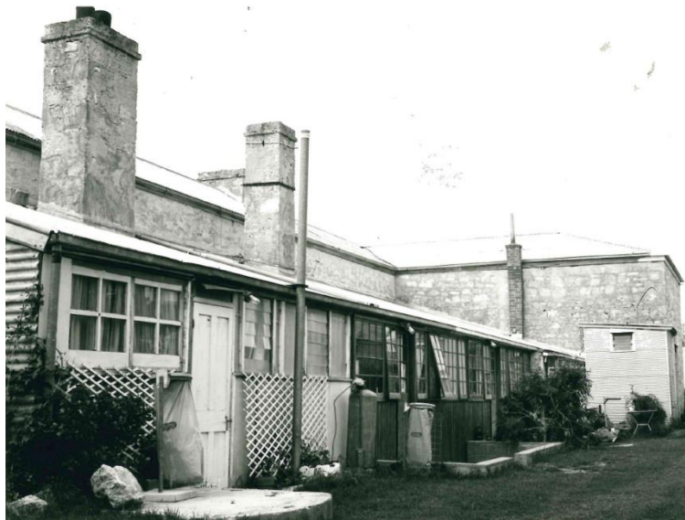
Rear of the building showing lean-tos and stone chimneys, c.1983.
