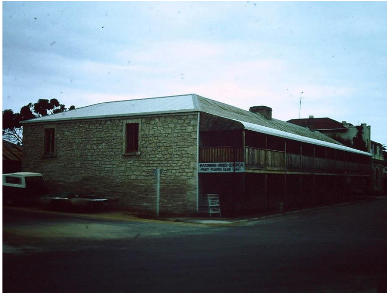
North-east corner of the building, c.1983.
