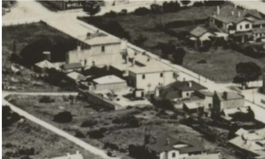
Closeup of an aerial view of Robe showing the terrace cottages have been extended to integrate the store into them on the north-eastern corner, c.1940.
