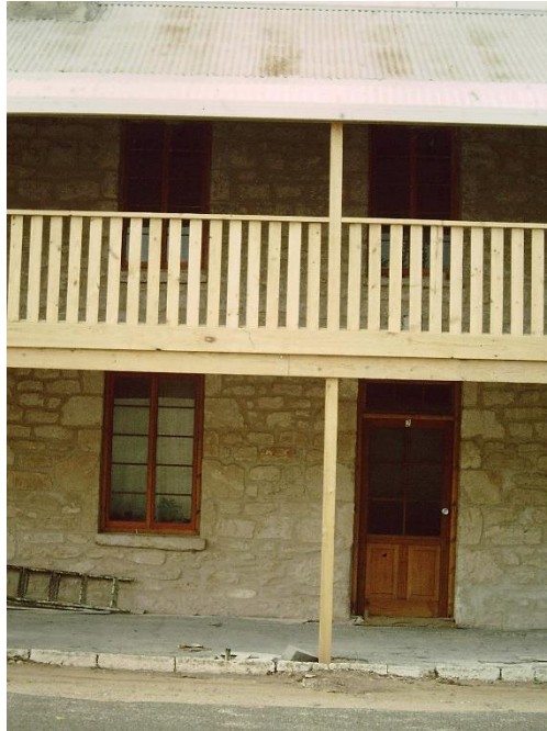
Image shows a newly erected timber balcony, c.1983.
