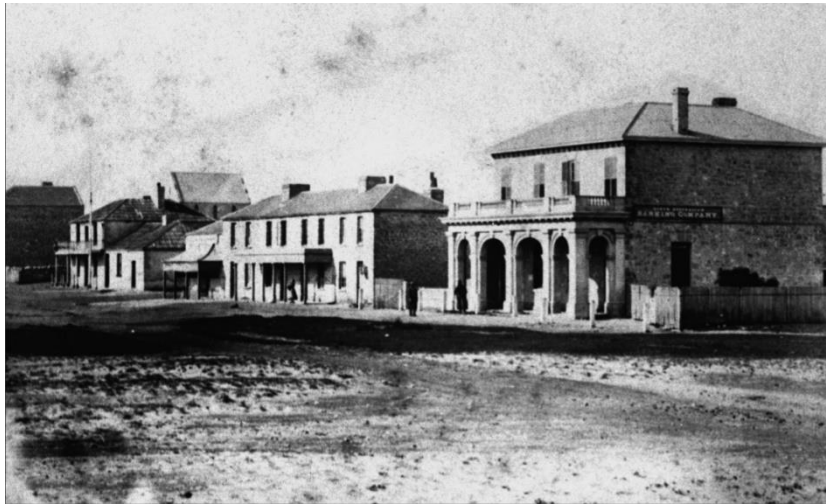
Campbell's Store and Cottages (left) and Bank House (SHP 12543), c.1880. Note the store to the left of the building and the eight windows to upper level on the terrace cottages.
