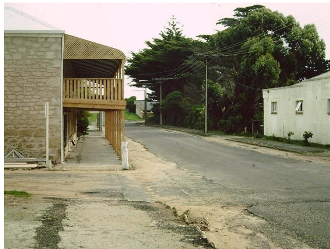
View of the building showing the timber balcony including lattice work, c.1983.
