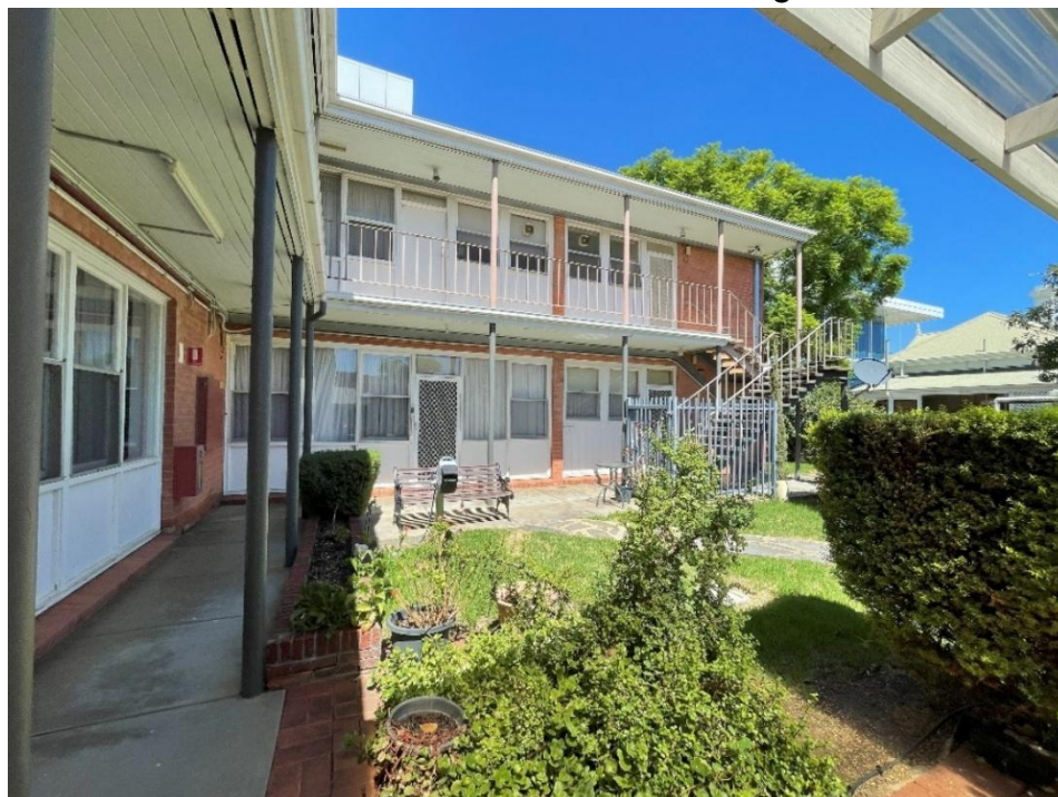
Portion of northern elevation of Lorna Hosking House.
