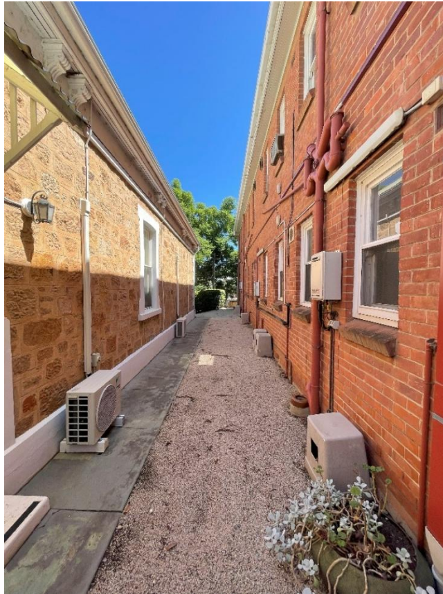
Portions of the southern elevation of Vasey Flats and northern elevation of Jean Rouse Villa.
