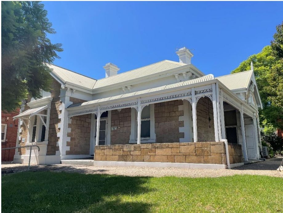
Western elevation of Jean Rouse Villa.
