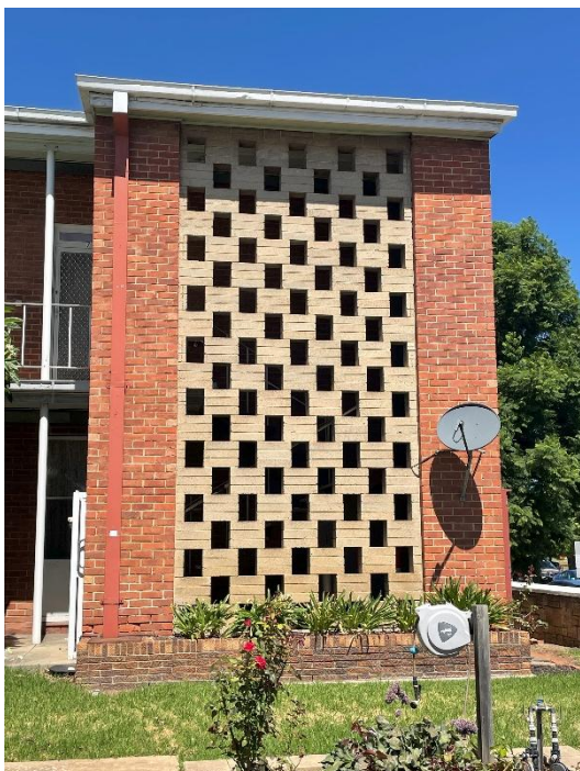
Protruding stairwell with hit and miss cream brick detailing to northern elevation of Vasey Flats (west).
