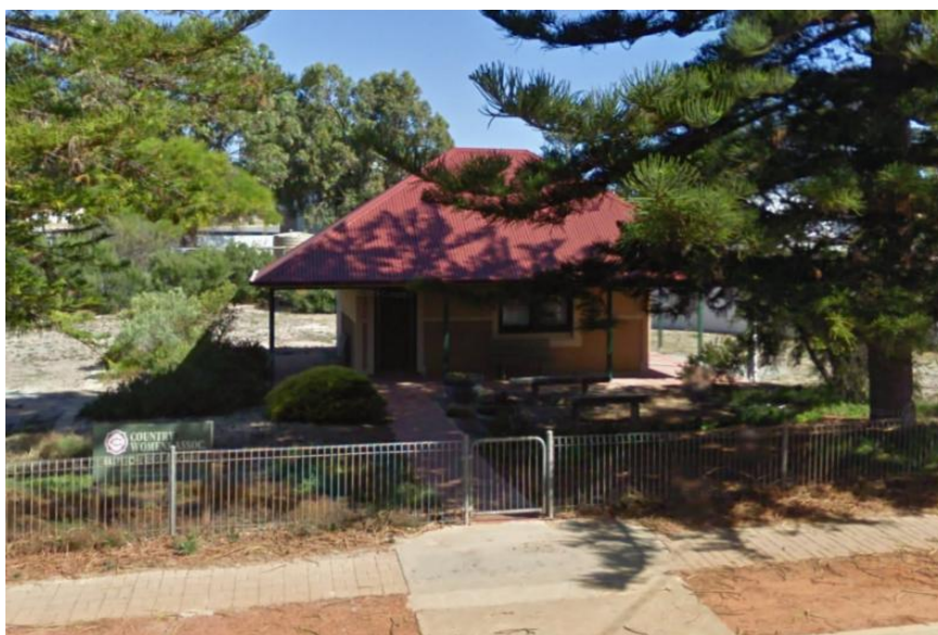
Hall – CWA Clubroom (SHP 14204), 9 Memorial Drive, Elliston.
