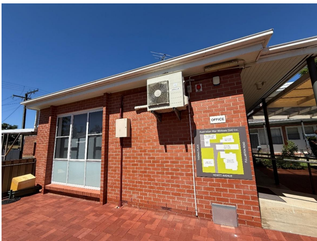
Portion of northern elevation of Lorna Hosking House.
