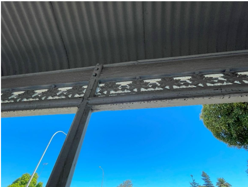
Cast iron railing along northern verandah fascia of Vasey House.
