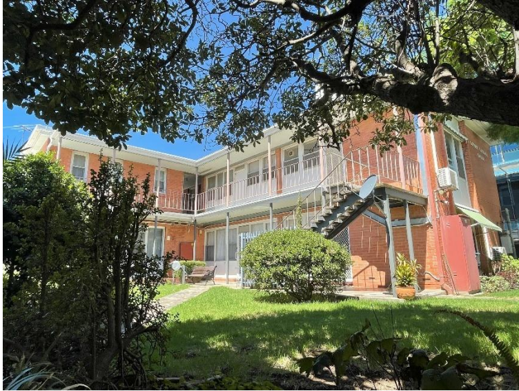
North-western view of Lorna Hosking House
