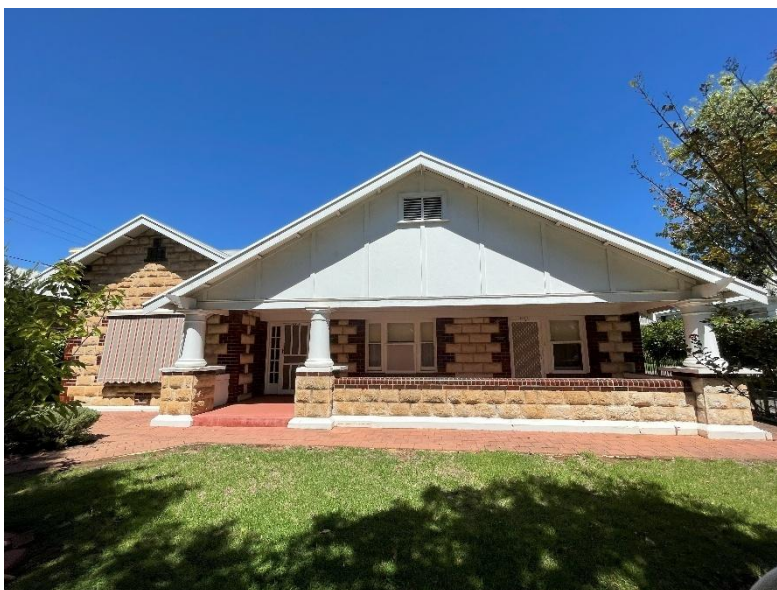
Northern elevation of 2A Hewitt Avenue (Joyce Mobsby Cottage and Joan Hogben Cottage)
