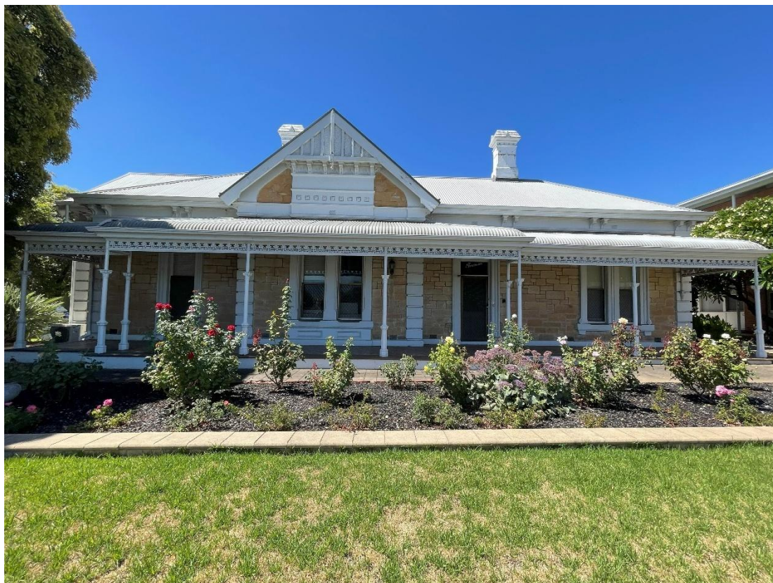
Western elevation of Vasey House.
