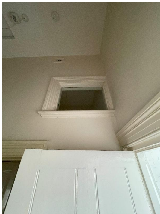
Interior of Vasey House (southern half)
