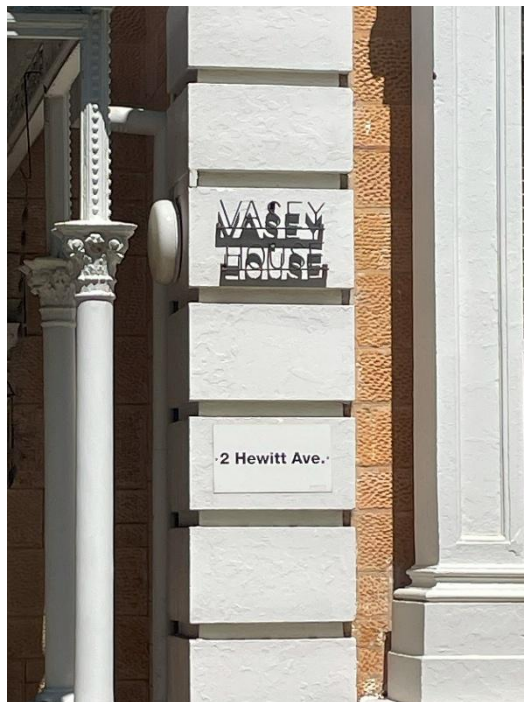
Name plate on quoins on northern elevation of Vasey House.
