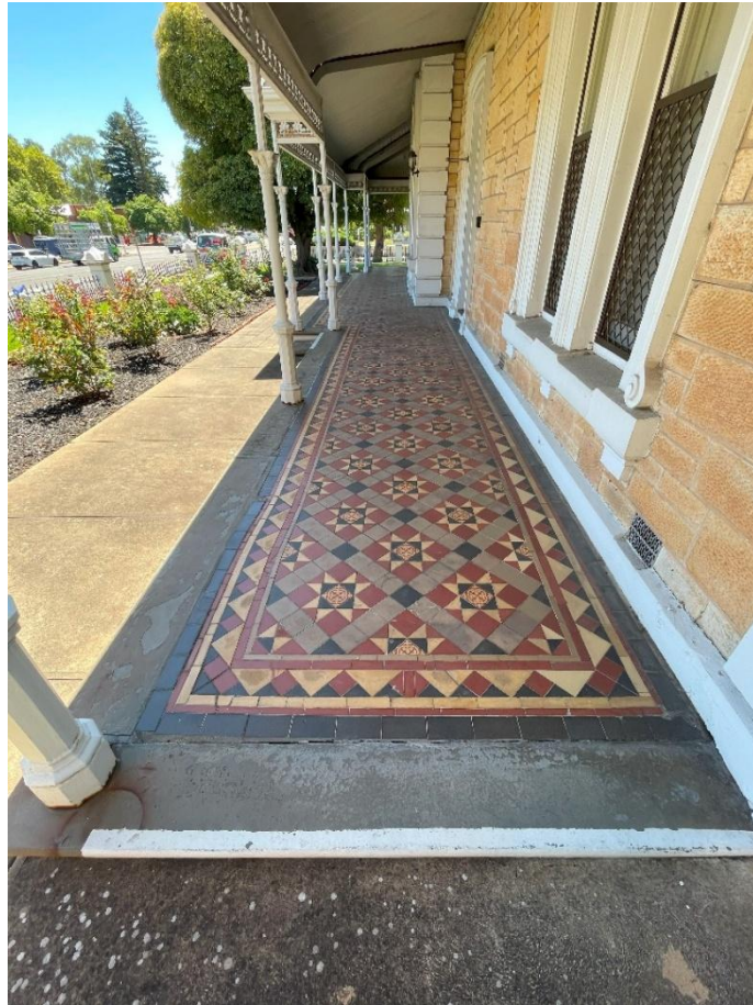
Verandah western elevation of Vasey House, note tessellated tiles.
