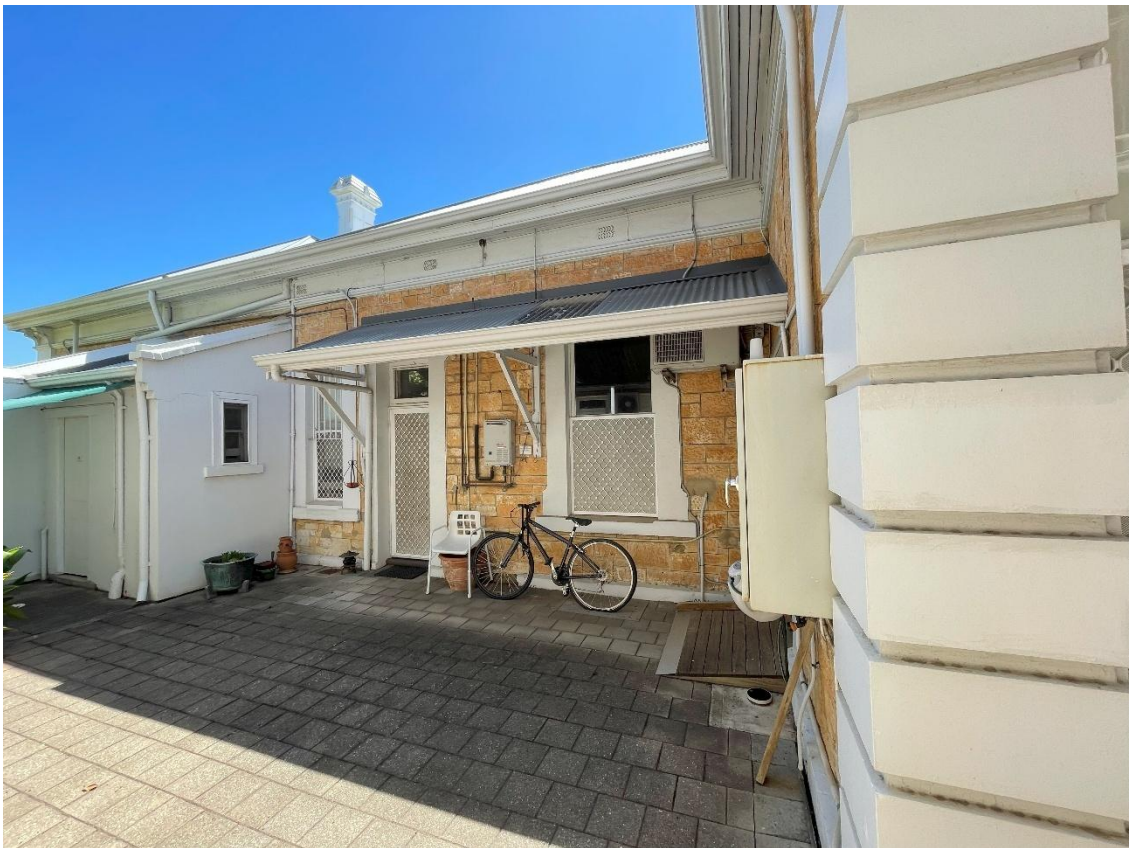
Portion of southern elevation of Vasey House.
