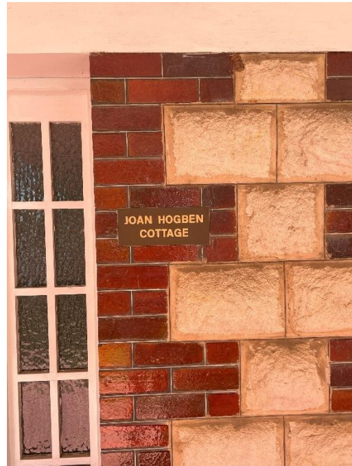
Nameplate for Flat 2 of 2A Hewitt Avenue.
