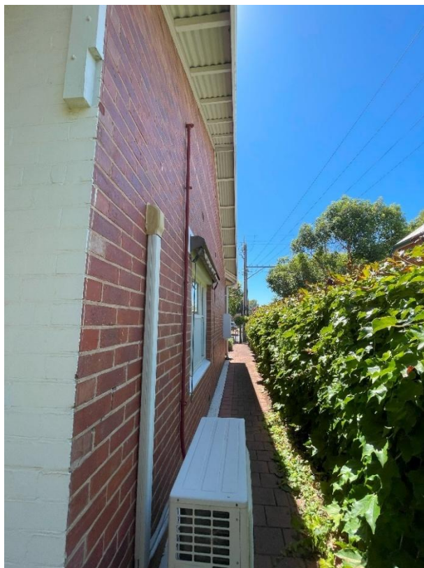
Portion of eastern elevation of 2A Hewitt Avenue.
