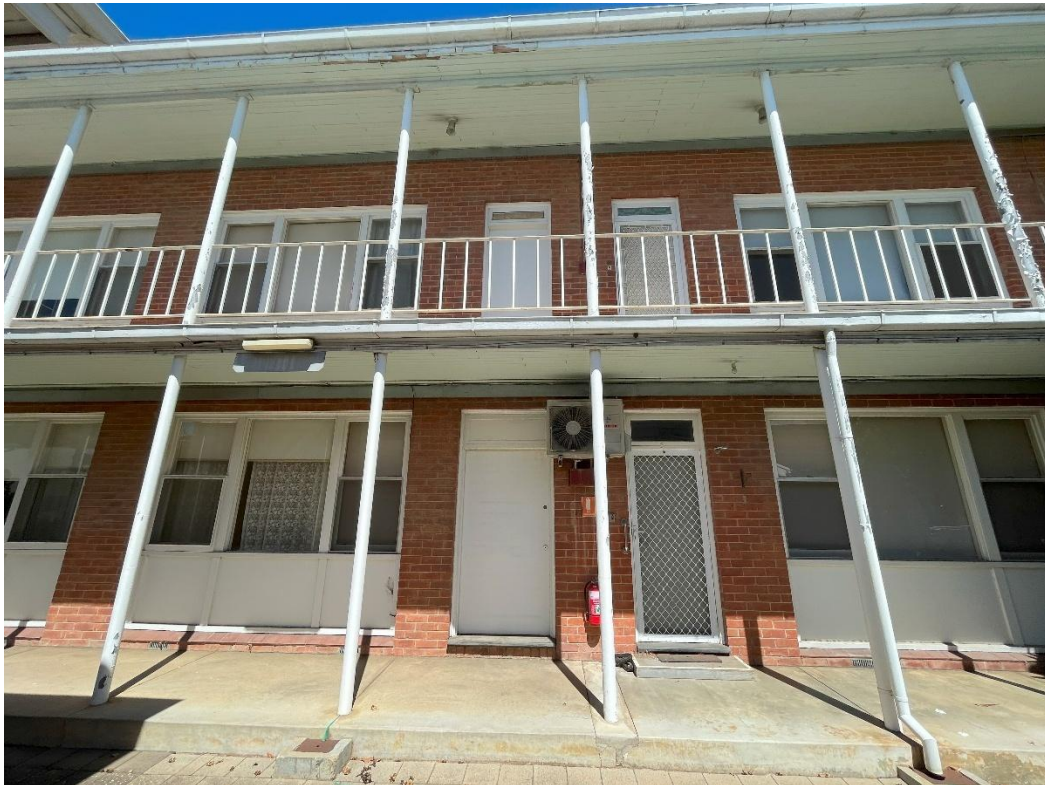
Portion of northern elevation of Vasey Flats.
