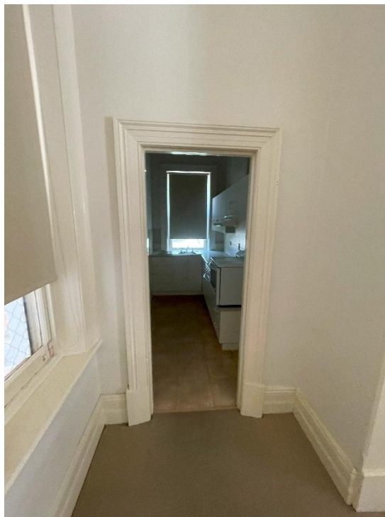
Interior of Vasey House (southern half)
