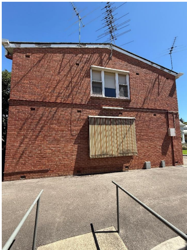
Eastern elevation of Vasey Flats.
