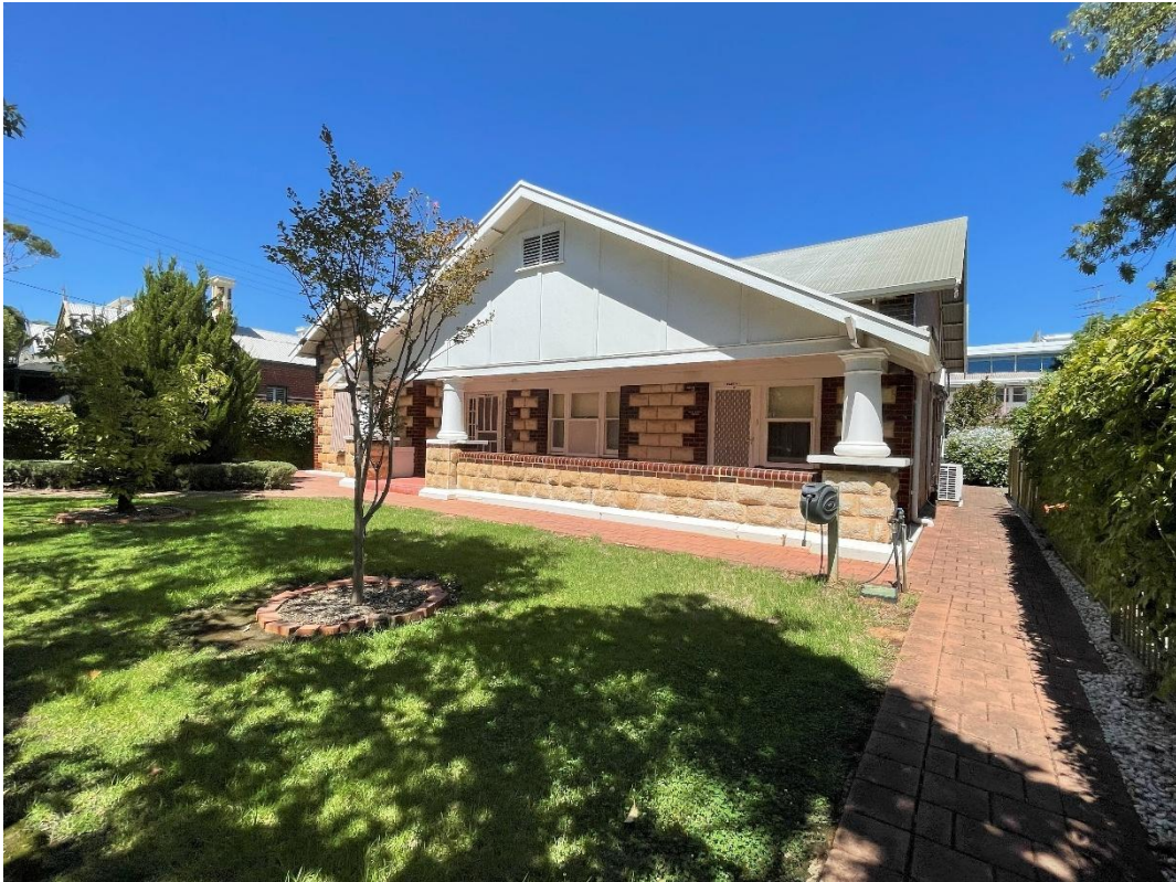
Portion of northern elevation of 2A Hewitt Avenue.
