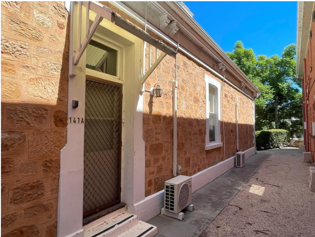
Portion of northern elevation of Jean Rouse Villa.
