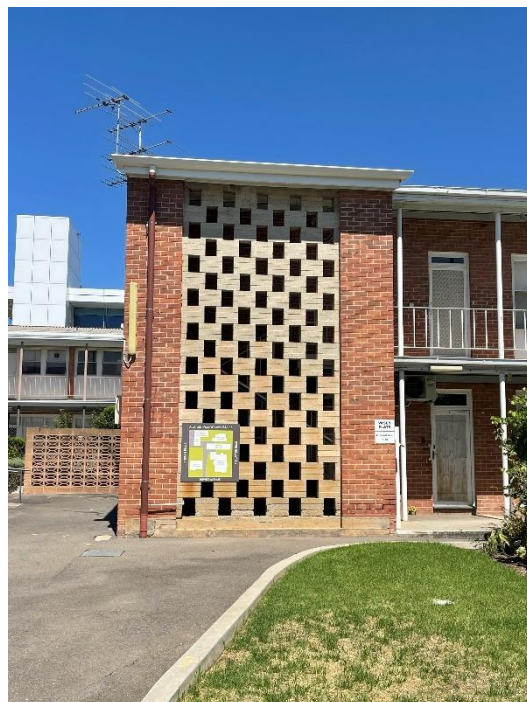
Protruding stairwell with hit and miss cream brick on northern elevation of Vasey Flats (east).
