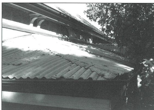
Lead hip capping on a verandah
