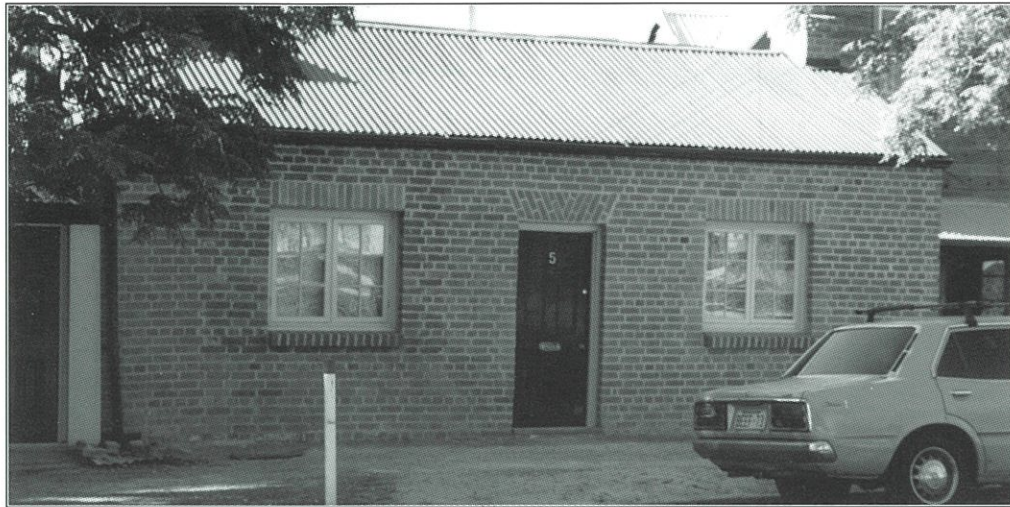
Gable roofed cottage in Willunga
