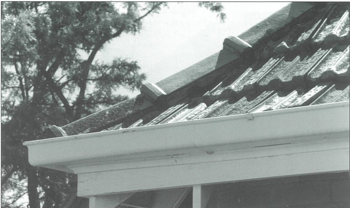
Original Ogee gutter replaced by D gutter
