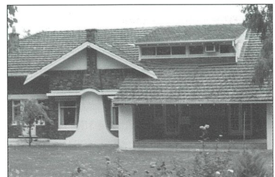
Tiled roof on Tudor Bungalow
