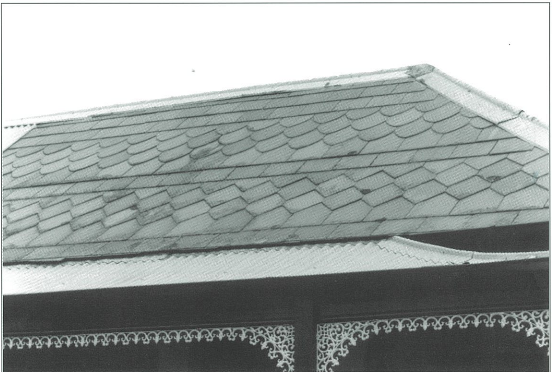
Detail of patterning of roofing slate Note use of three different slates
