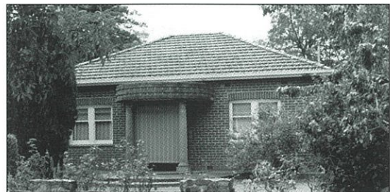
Diagonal roofing tiles
