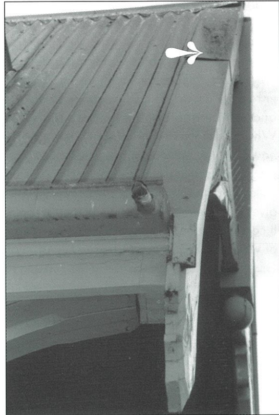
Historic gable design compromised by replacing original timber capping with new folded metal capping
