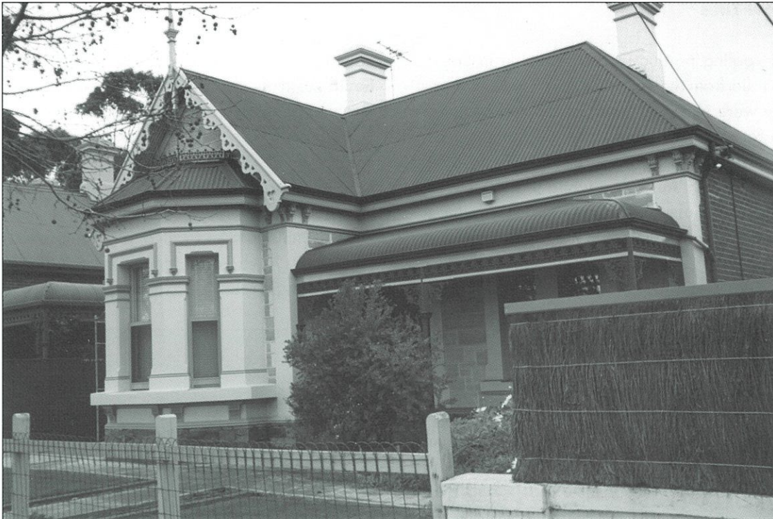
A villa in Norwood roofed with corrugated steel. Note bull-nosed roof on verandah and decorated hipped bay window roof.
