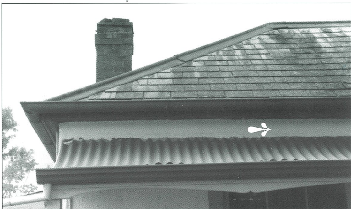
Verandah roof with rendered flashing
