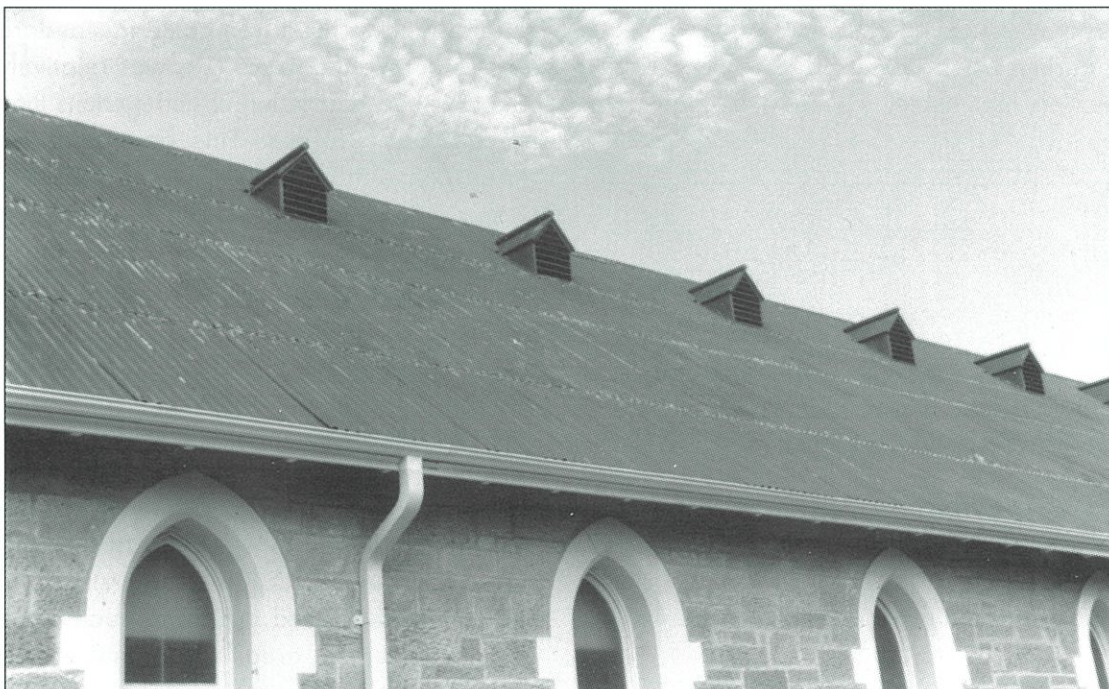
Church hall roofed with original 6'0" long sheets of corrugated iron. Note the pattern or texture the small sheets make.
