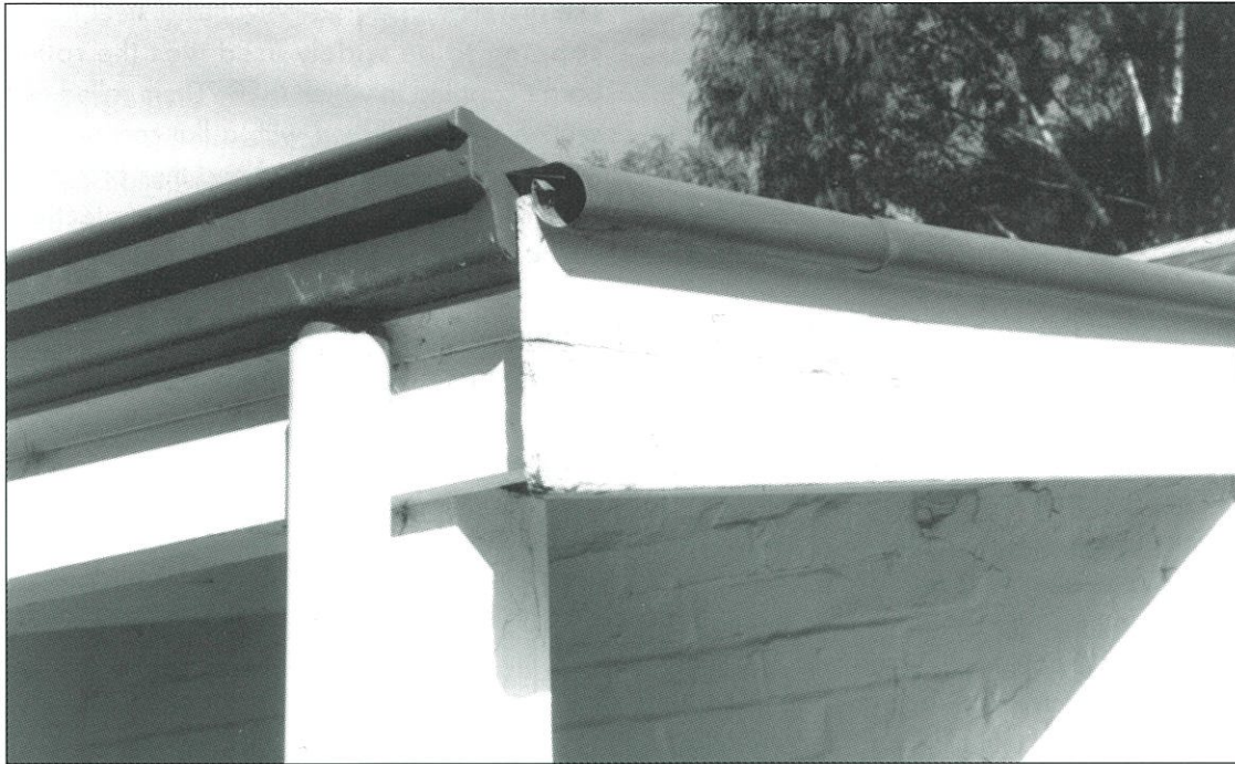
Rolled barge capping on lean-to
