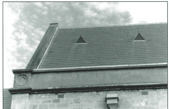
Gablette vents in slate roof
