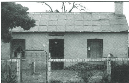
Cottage in Penola with metal tile roof
