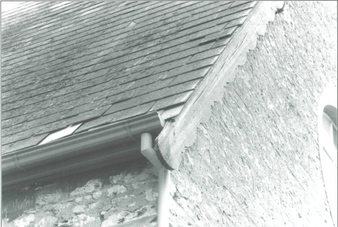
Detail of a slate roof gable end Note verge detail and loose slates
