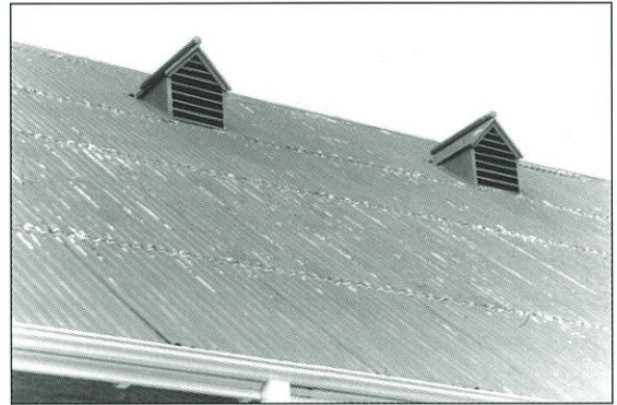
Roof vents in corrugated steel roofing. Note pattern created by roof cladding.
