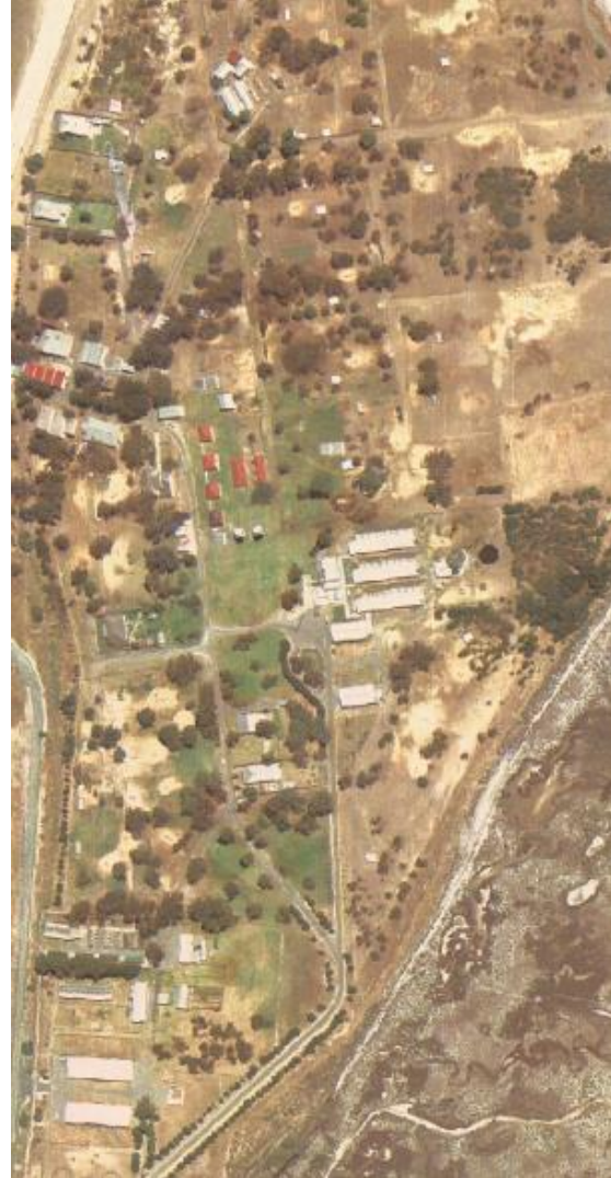
Aerial map of the station dated 1986-1989 illustrating the animal paddocks of the animal quarantine station. The feed sheds can be seen dotted around the human quarantine structures.
