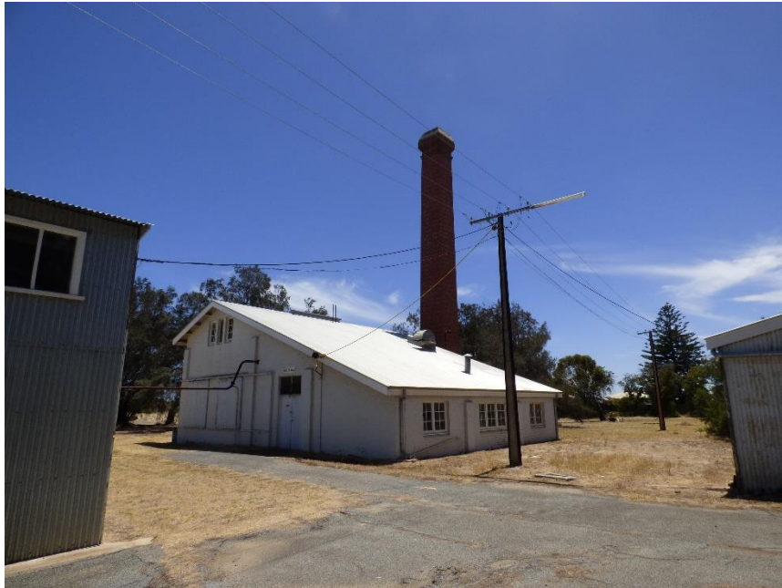
The boiler house and chimney.
