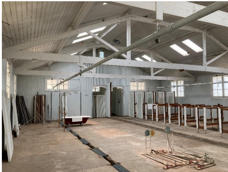
Interior of the bathing block. The cubicles were removed when the human quarantine station closed.
