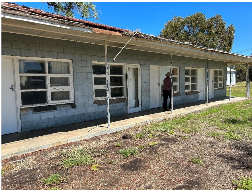
The eastern accommodation block in January 2024. This building was mainly used as a storeroom during animal quarantine.
