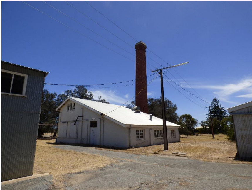
The boiler house and chimney.
