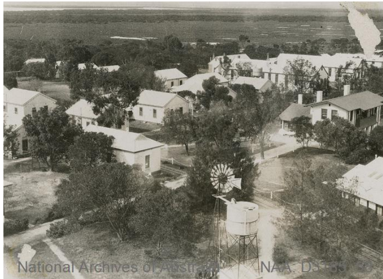
Tramway through the Torrens Island Quarantine Station in the 1920s.
