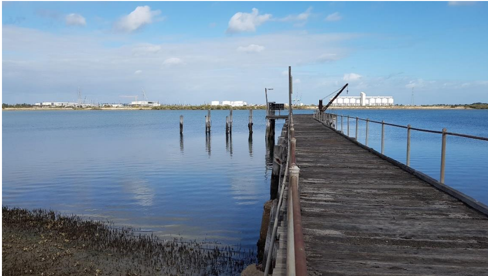
Human passenger jetty in 2021, note the crane.
