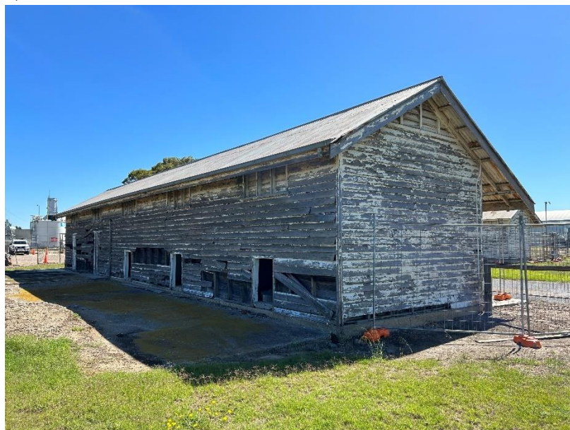
Rear of the horse stable with access doors.
