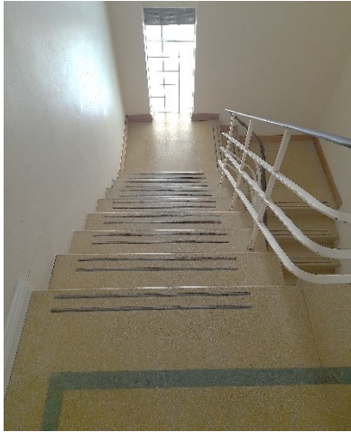
Internal stairwell with original terrazzo
