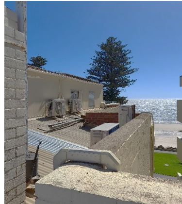
New structure built on former roof terrace area
