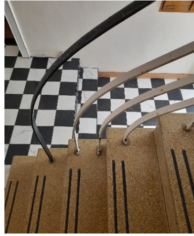
Internal stairwell showing original terrazzo treads, railing and new tiles
