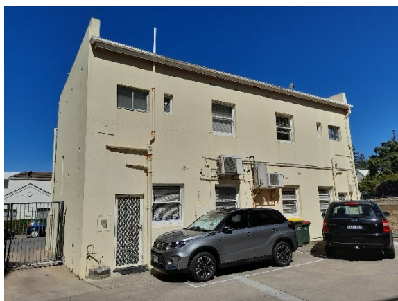
Rear view of freestanding townhouse block
