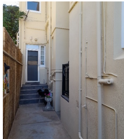
Former location of demolished reinforced concrete service stairs on southern side
