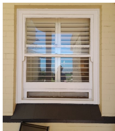
Remaining original window with integrated sliding flyscreen
