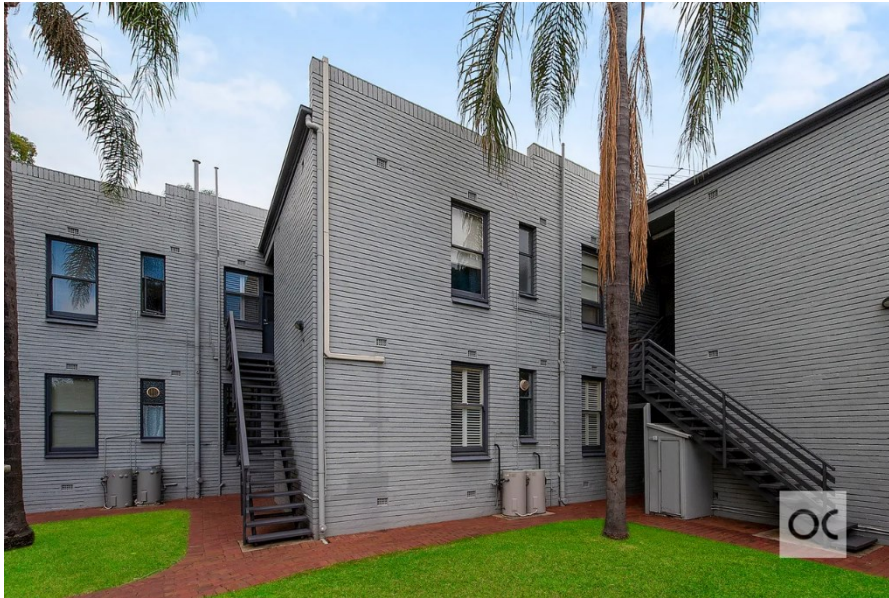
Rear view looking south-east
