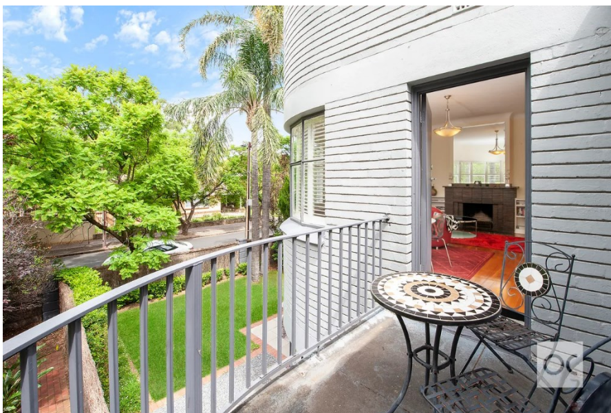
Upstairs balcony showing horizontal raked pointing
