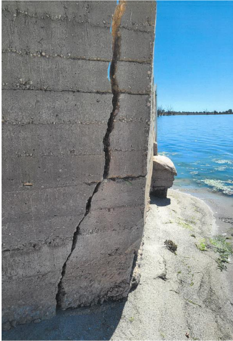
Nookamka No. 1 (Lake Bonney) Pumping Station Dam Wall Ruin, showing damage to northeastern corner, c.2012
