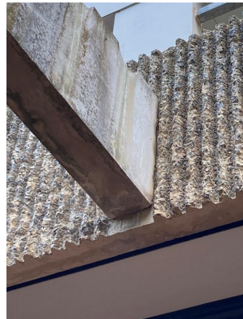
Examples of the balcony panels with exposed aggregate.
