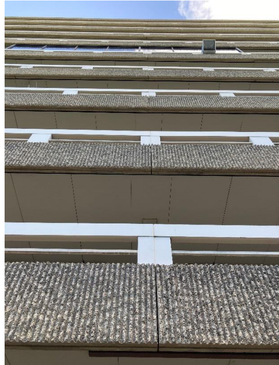
Balcony, showing the exposed aggregate concrete panels and balustrading.
