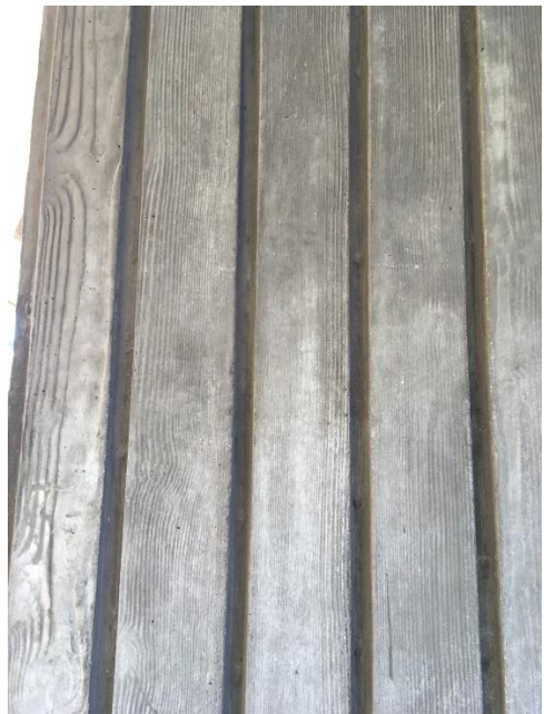
Example of the off-formwork to external columns.
