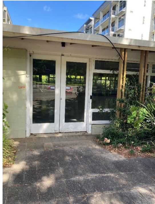
The chapel showing the southern elevation (left) and main entrance (right) note the hopper windows.
