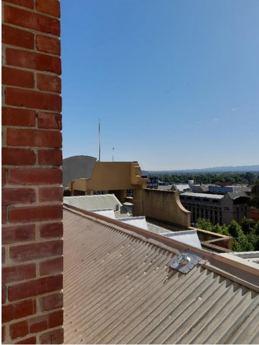
Hipped-roof and rear of the parapet wall.
