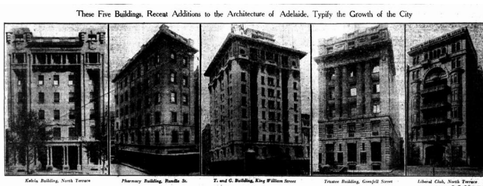
Five buildings the Mail believed exemplified 'Adelaide Growing Up' and showed the 'Remarkable Progress in [the] Metropolis', May 1926.
