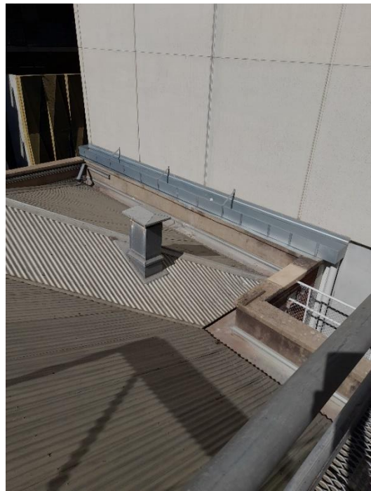
Hipped-roof at rear showing H-shape.
