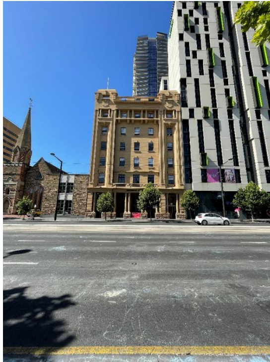
Front elevation of the Kelvin Building facing North Terrace.
