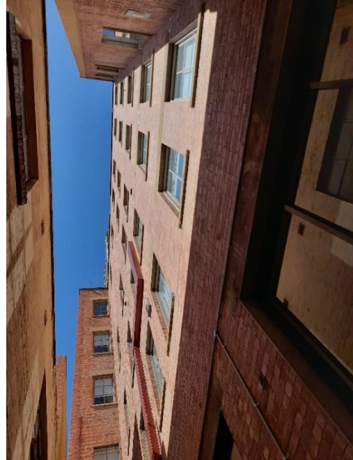
Eastern elevation revealing H-shape.
