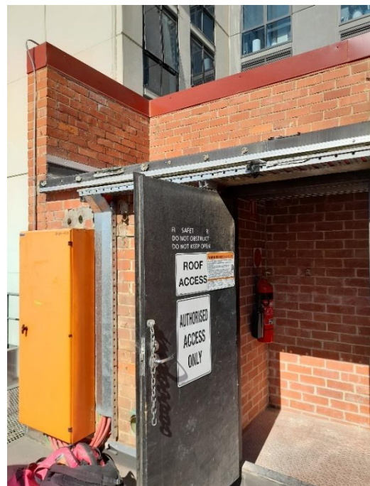
Entrance to roof.
