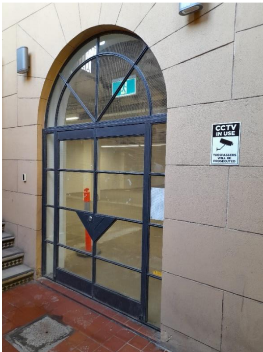
Steel-framed basement entrance.
