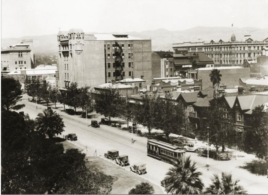
View of the Kelvin Building facing towards the east, c.1925-1927.
