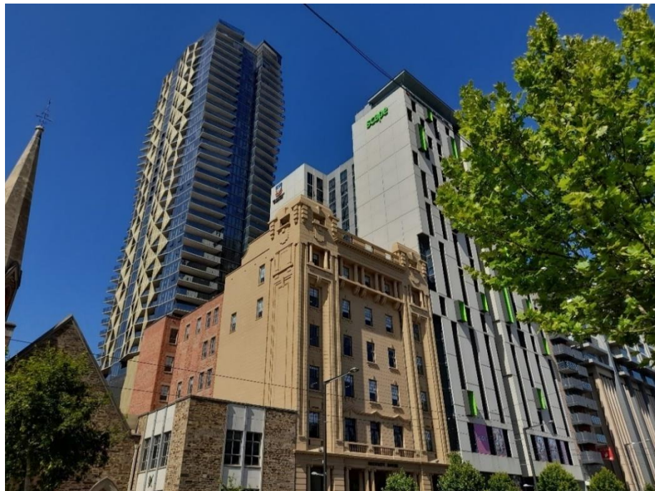
North-eastern corner of the Kelvin Building showing the front elevation and depth of return to eastern elevation and unrendered red-brick portion of the building, with internal bay to provide natural illumination.
