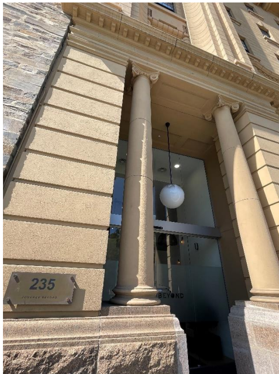
Left front porch on eastern elevation.
