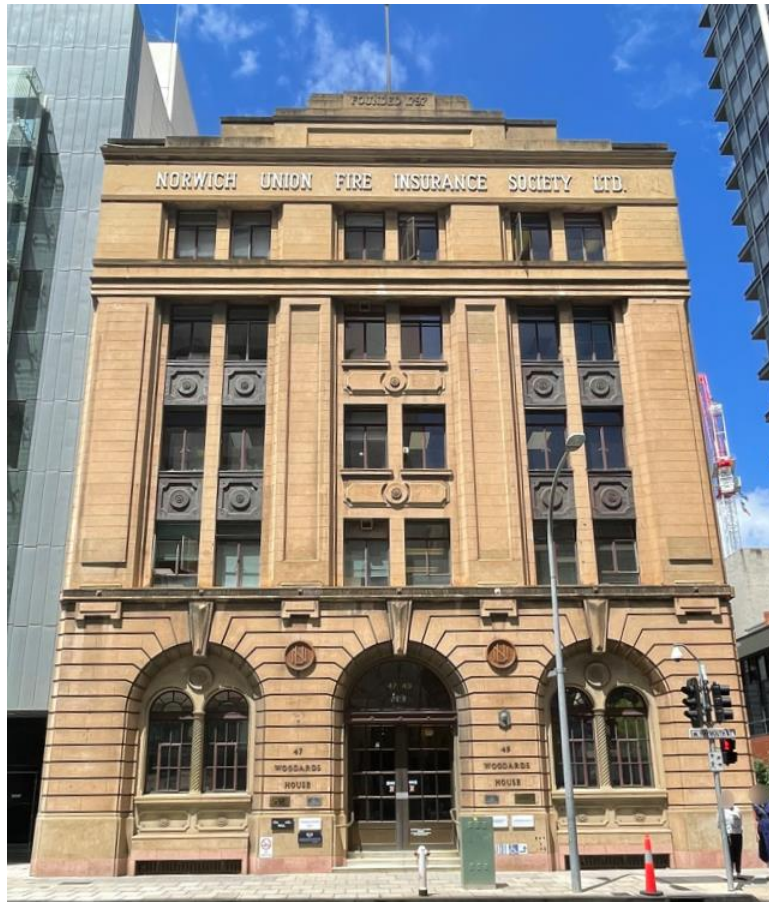
Woodards House (SHP 13106)
