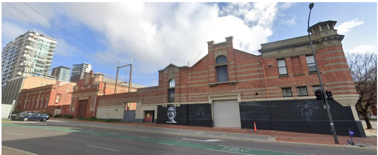
Tandanya (former Adelaide Electric Supply Company Power Station) (SHP 10984) (right), Former Adelaide Electric Supply Company Converter Station (SHP 10985) (middle) and Former Municipal Tramways Trust (MTT) No.1 Converter Station (SHP 10986) (left).
