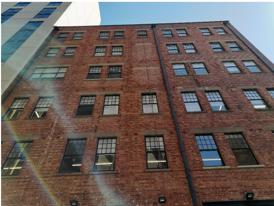
Southern rear elevation at the rear showing red-brick construction.
