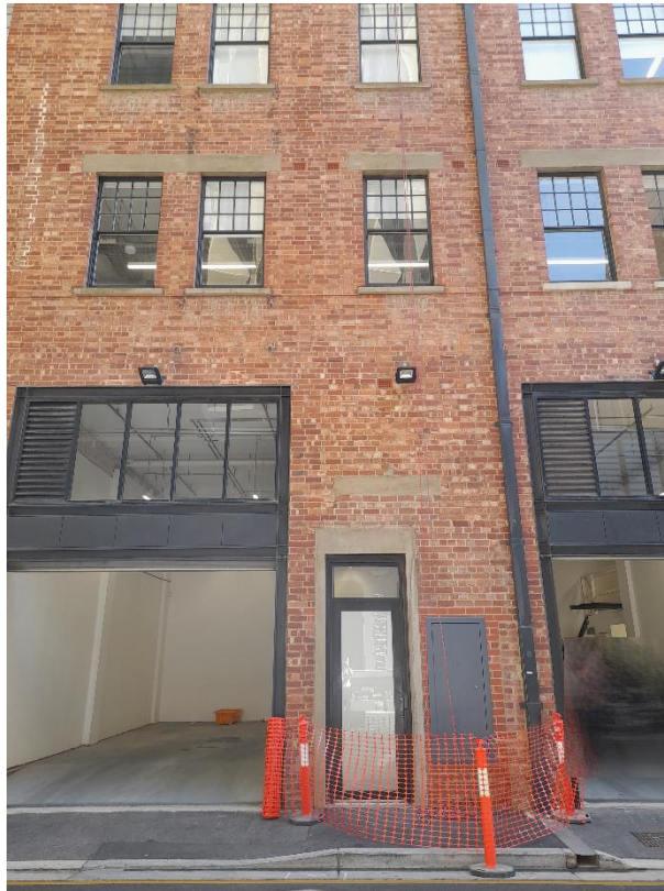
Southern elevation at the rear showing roller door garage entrances.
