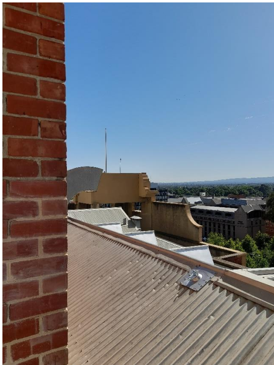
Hipped-roof and rear of the parapet wall.
