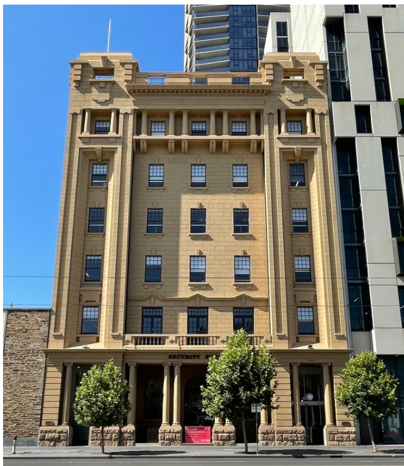
Kelvin Building, 233-236 North Terrace, Adelaide 5000
