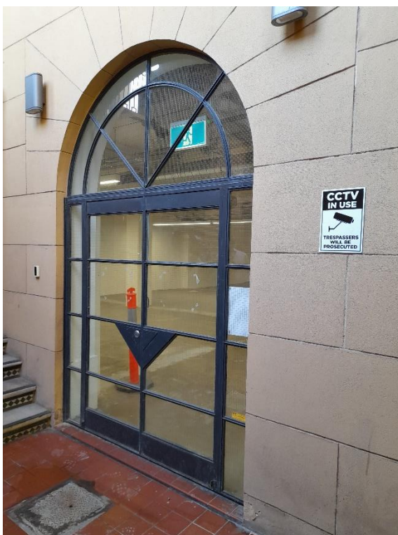
Steel-framed basement entrance.
