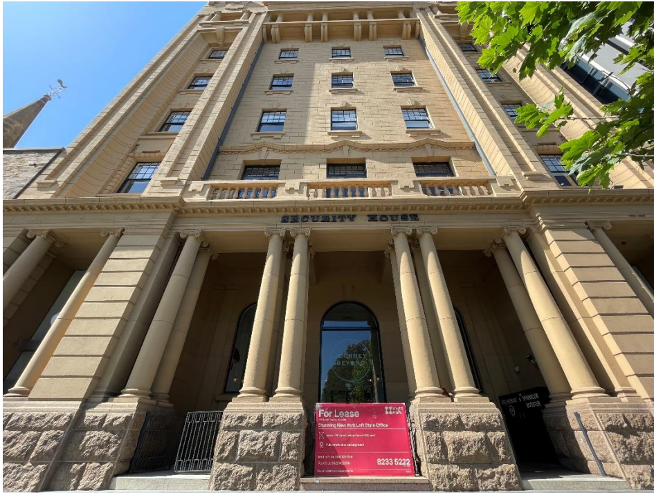
View of the front showing Ionic columns, rustication, and balustrade.
