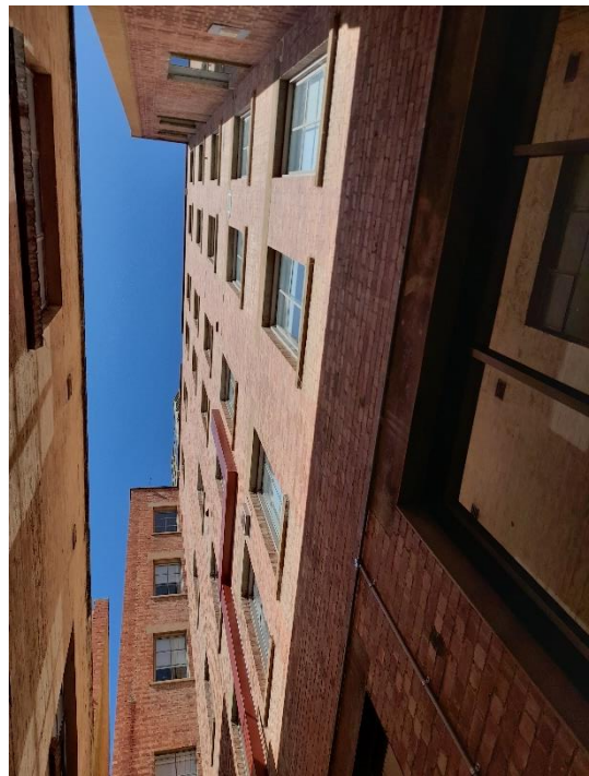
Eastern elevation revealing H-shape.
