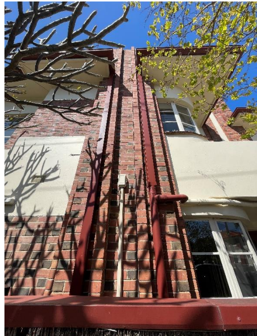
Northern elevation showing one of the chimney towers with Flemish bond coursework.
