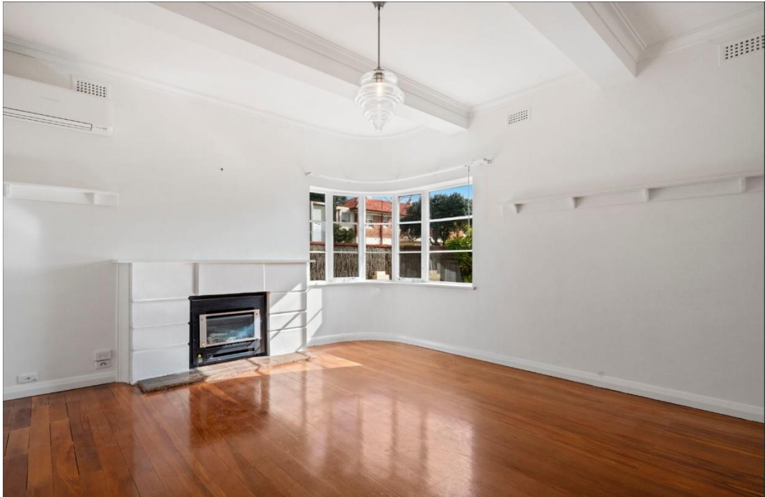
Lounge room of western downstairs flat, showing original fireplace, shelving and concrete beams supporting second storey floor.
