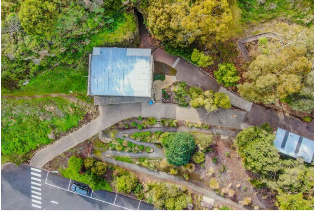
A portion of the Tantanoola Caves Conservation Park visitor information centre from above. The accessibility ramps leading to the cave entrance can be seen top left
