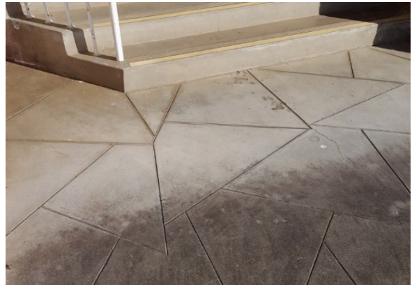
Concrete paving with triangular contraction pattern, 30 September 2023
