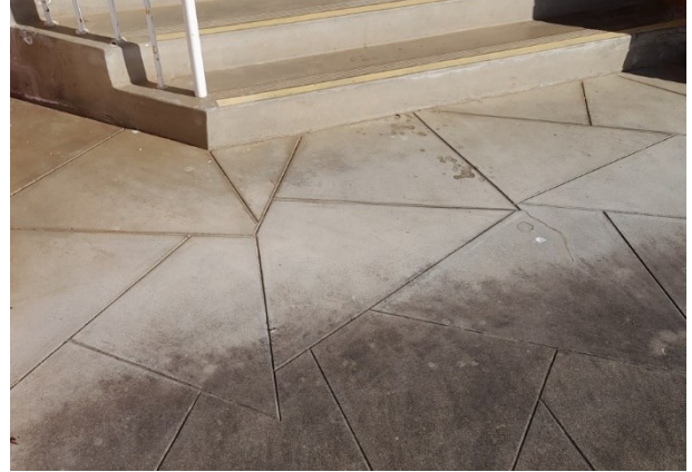
Concrete paving with triangular contraction line pattern, 30 September 2023
