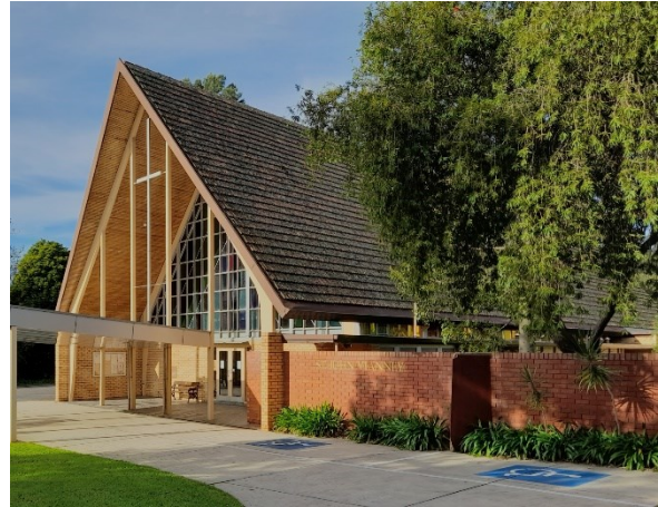
St John Vianney's Catholic Church, Burnside, 1962 (SHP 26543), is an example of a raised A-frame church
