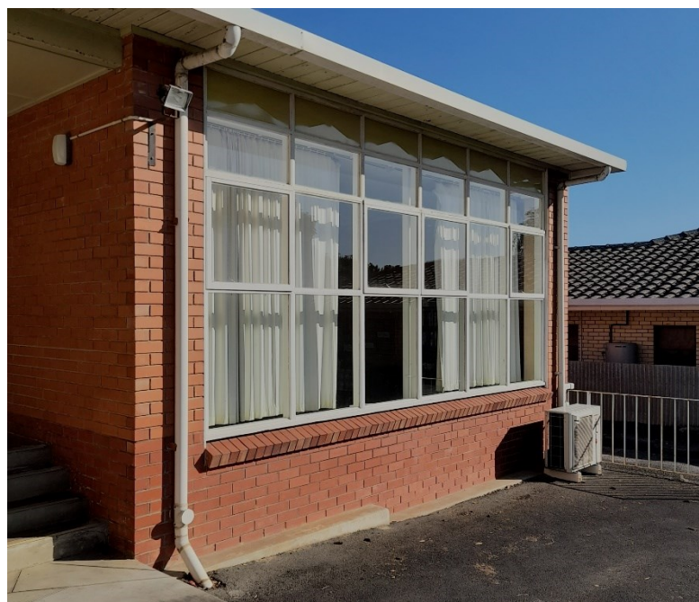
Kindergarten wing, 30 September 2023
