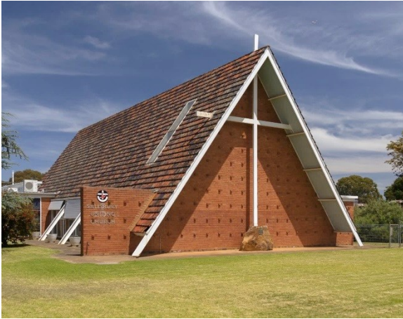
Former Salisbury Methodist Church, 1961, is an example of a true A-frame church
