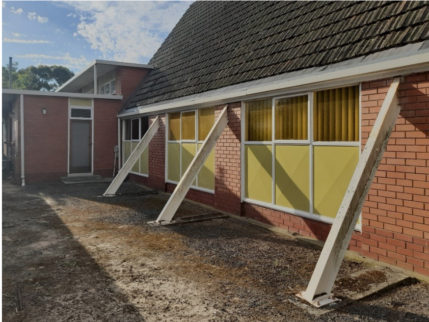
Southern side of chapel showing rolled steel 'buttresses' and 'Porcipanel' spandrels, 30 September 2023
